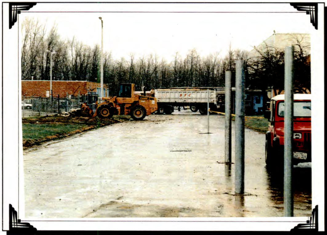
P-2 Loading of stockpiled soil (<5 ppm) onto trucks for off-site disposal.
