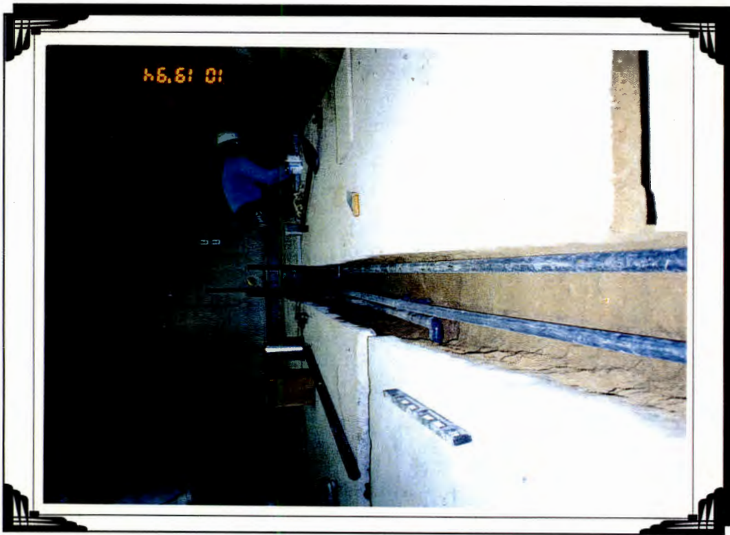
P-6 Installation of vapor recovery and air injection piping within trench in previous polysulfide room (AOC #5).
