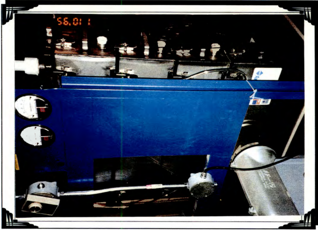
P-18 Three-tray air stripper (AOC #16).
