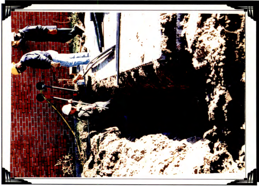
P-13 REW personnel installing recovery well piping along north side of treatment building pad (AOC #16).
