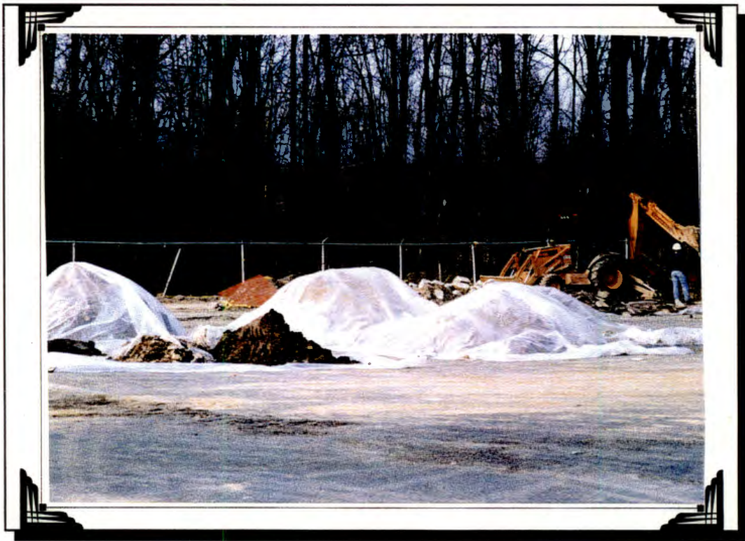
P-1 Excavated soil and debris (<5 ppm) stored on polyethylene sheeting east of the garage (AOC #16).
