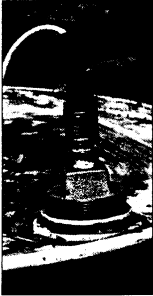
Product tank probe installed in a standard 2" NPT bung shuts the system off when the tank is full.
