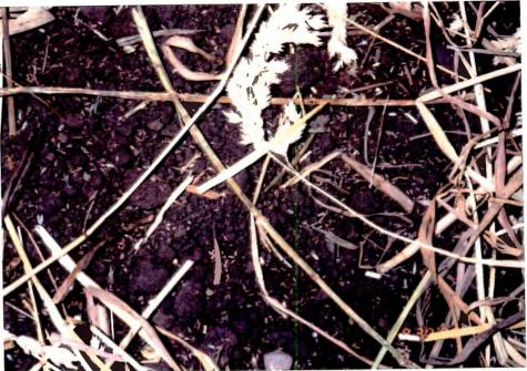
Status as of: AUGUST 30, 1996 Description: The contractor seeded the work zone as shown and then placed loose hay over the area.
