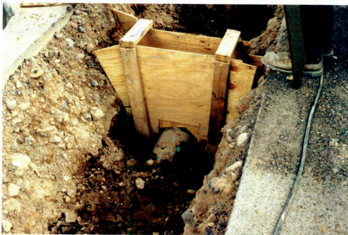
Seepage barrier formwork, typical
