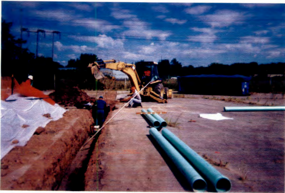
Storm sewer replacement activities, northwest storm drain system
