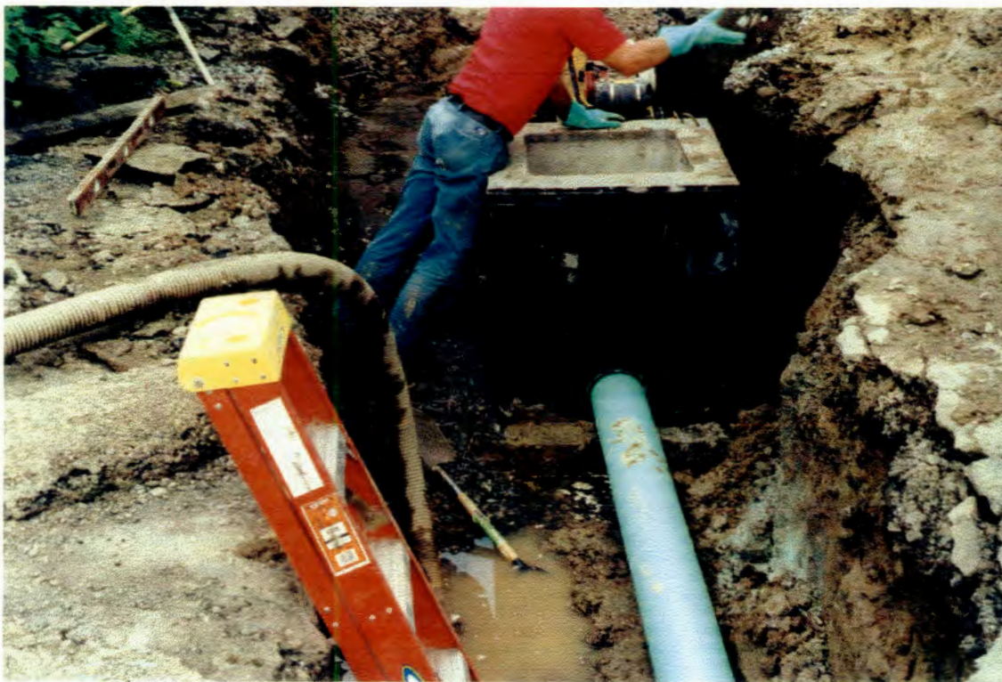
New Catch Basin 5 installation
