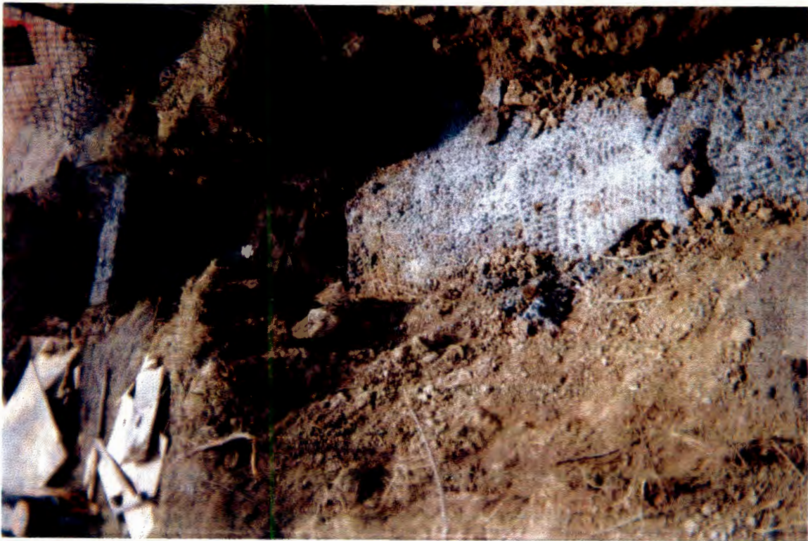
Completed seepage barrier/concrete encasement at water main crossing
