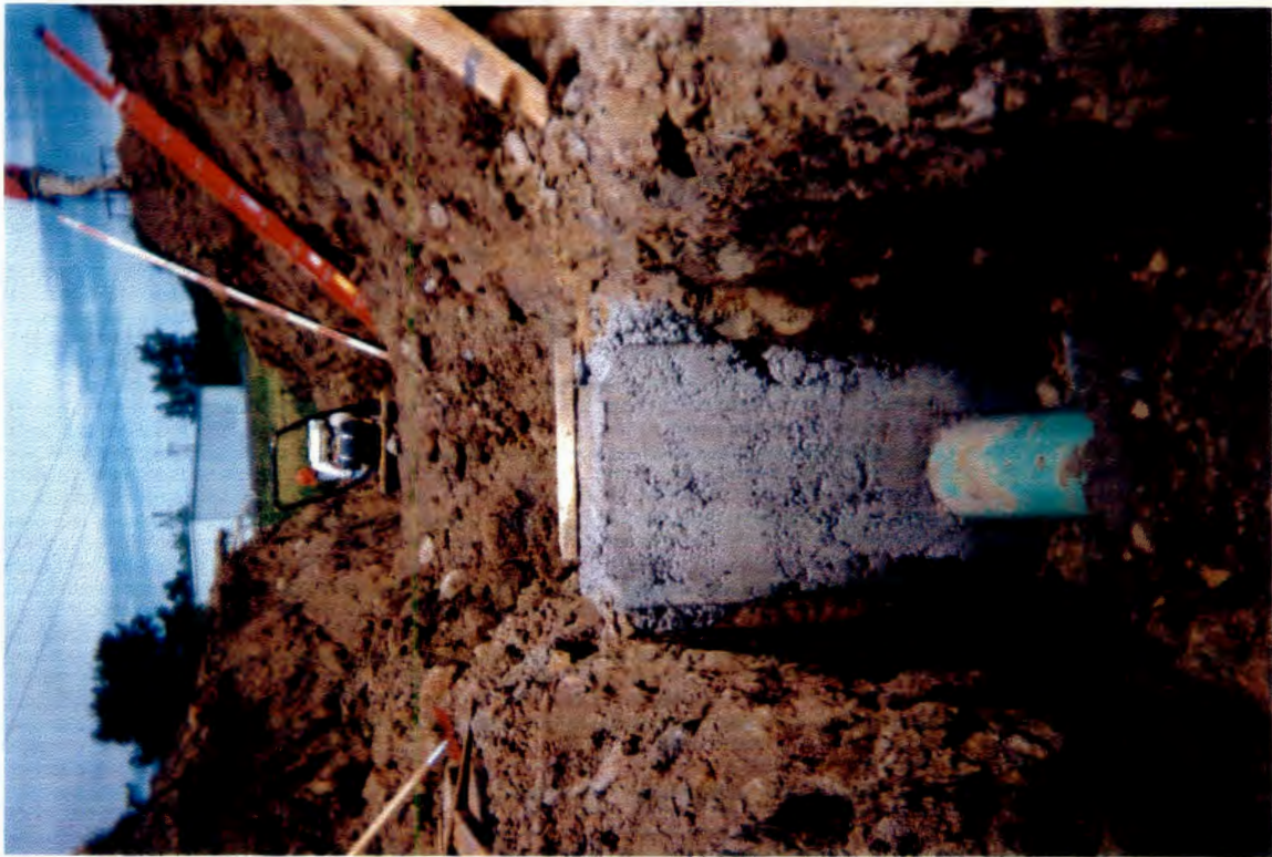
Completed seepage barrier
