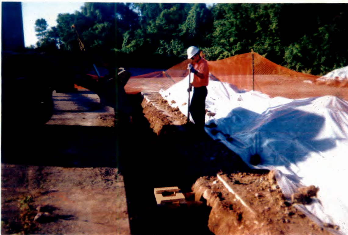
Trench backfill and seepage barrier
