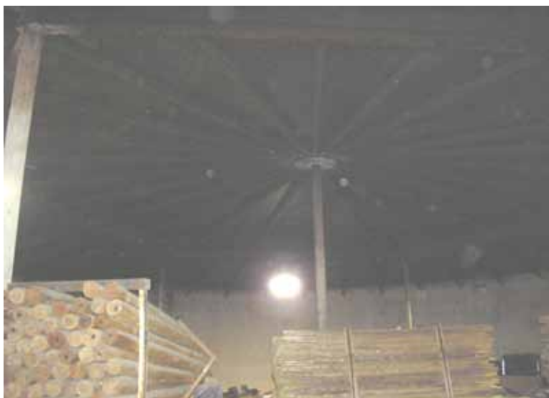
Photo 6: View of the spiral roof supports and columns of the storage tank. Date: 1/9/2009.
