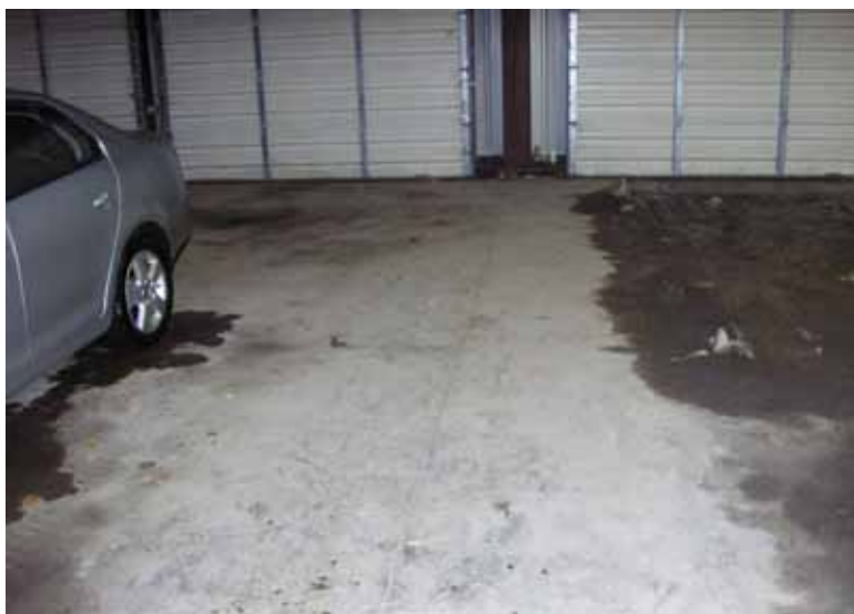
Photo 6: View of the Butler Fence garage flooring; no cracks were observed. Date: 1/8/2009.
