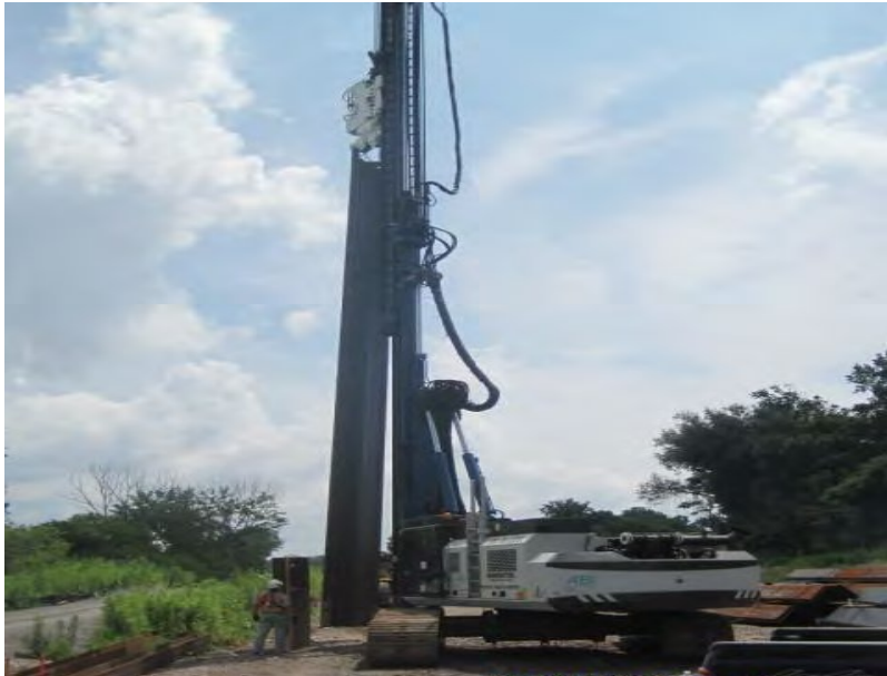
Figure 5: Installation of West Wall IRM
