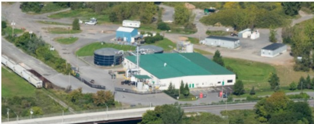
Figure 4: Willis-Semet Groundwater Treatment Plant
