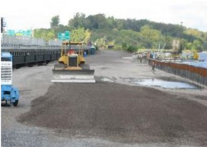
Figure 3: Installation of Willis-Semet Hydraulic Containment System IRM
