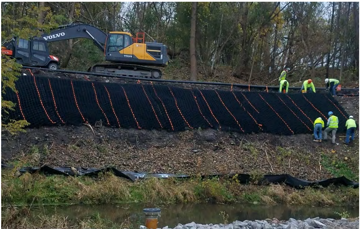
Week of October 27, 2019: Installation of Geocell
