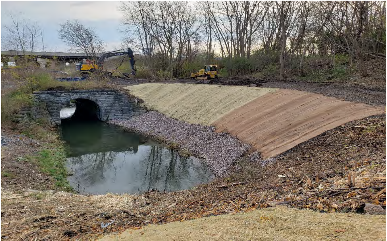
Week of November 3, 2019: Final Cover at OW-4 Slope
