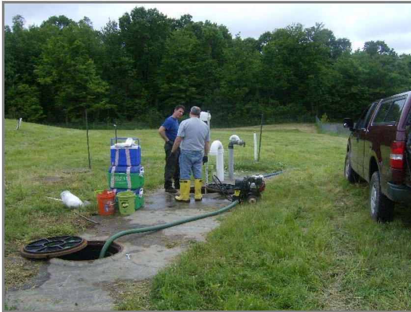
In pumping mode. We were draining the manway riser.
