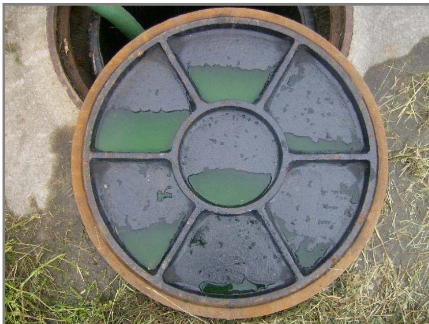
Tank manhole cover
