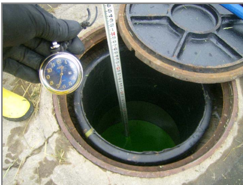
Pumping down the manway riser
