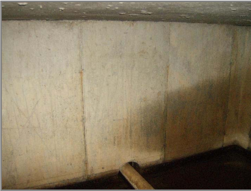
Outlet pipe which leads to the discharge point into the amphibian breeding pond.
