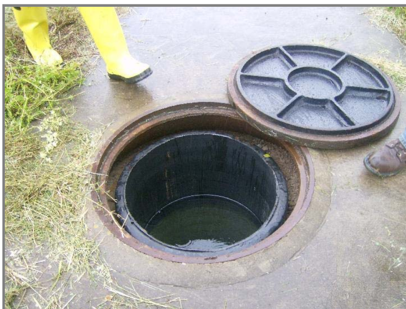
Manhole open, tank end.
