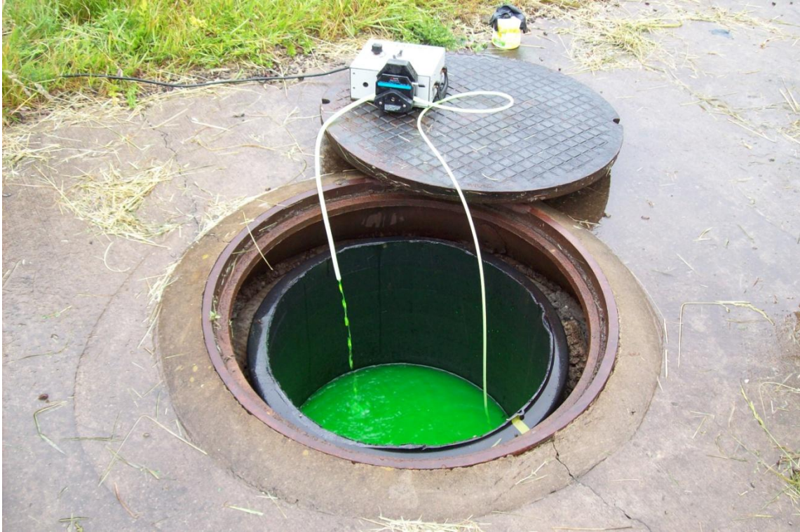
Photo 3: Fluorescent dye in leachate collection tank.
