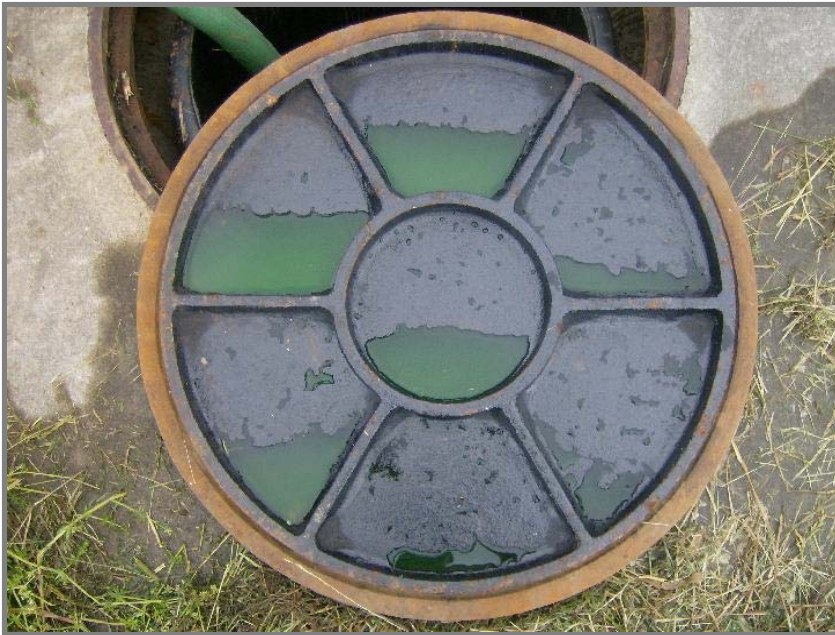
Tank manhole cover
