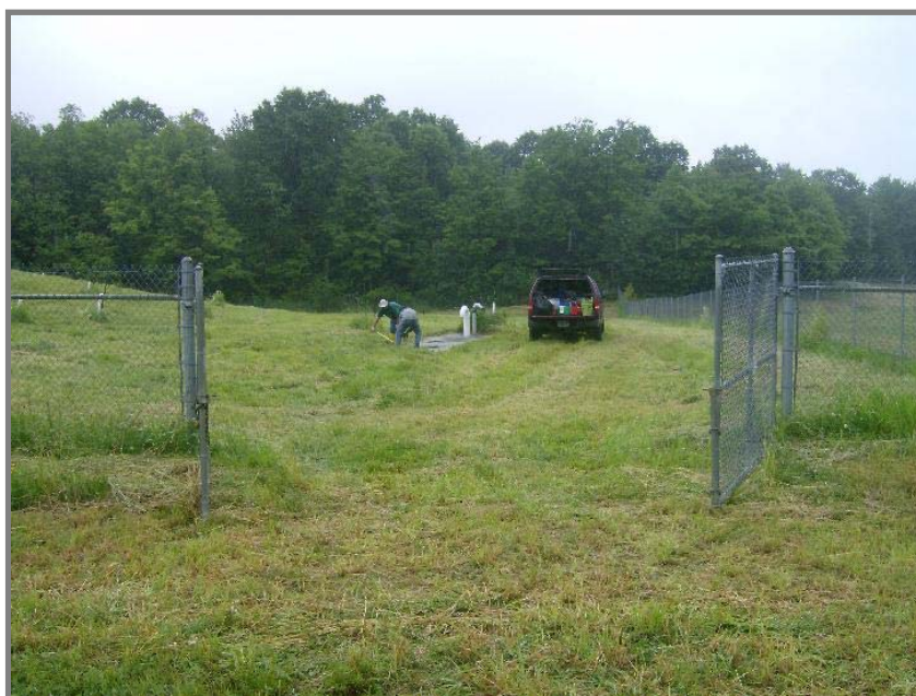
Gated access to the landfill. Jeremy and Payson are opening the manhole covers in the leachate tank area.
