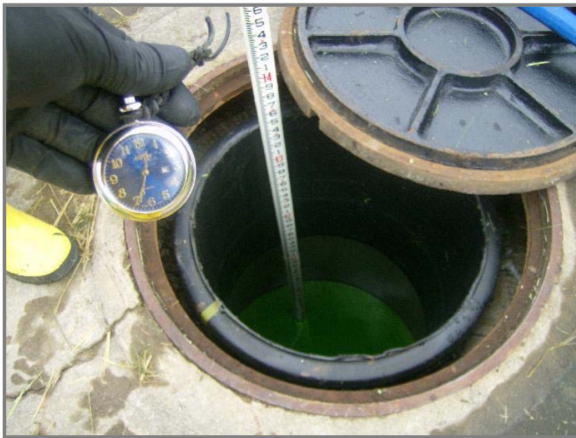
Pumping down the manway riser
