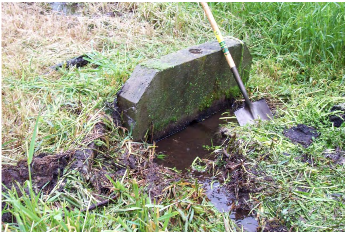
Photo 1: Discharge structure to Amphibian Breeding Pond.
