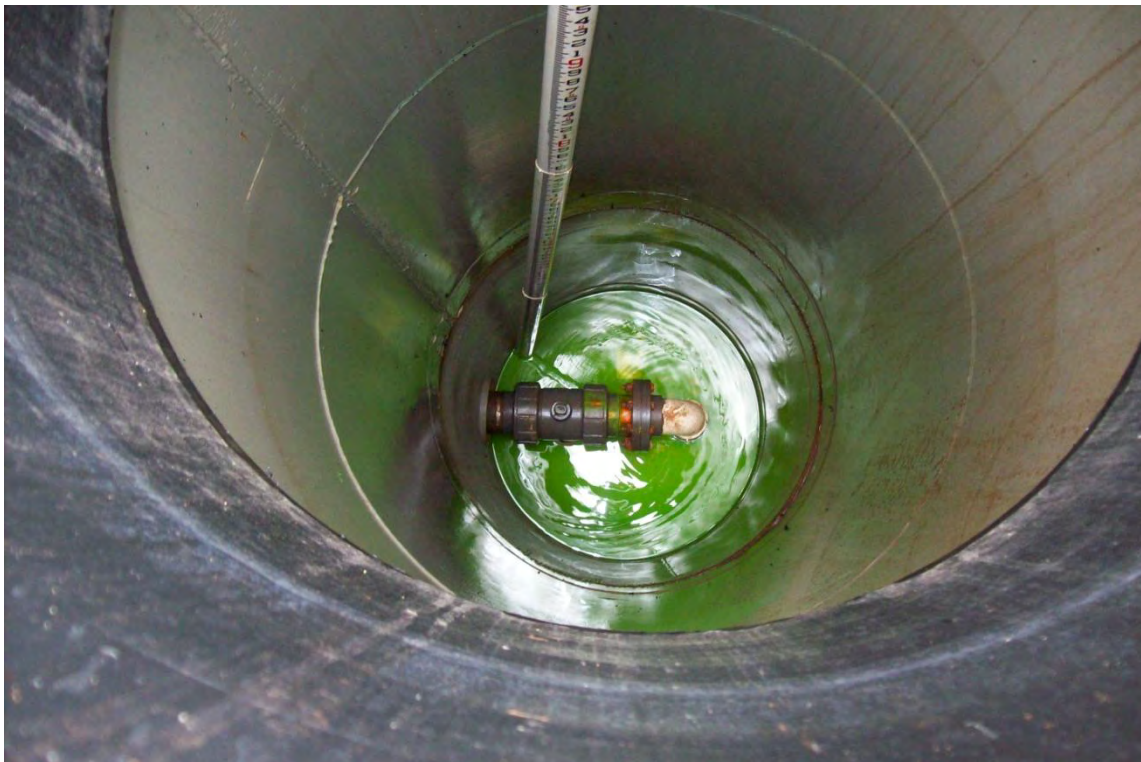
Photo 4: Inlet pipe manway and control valve.
