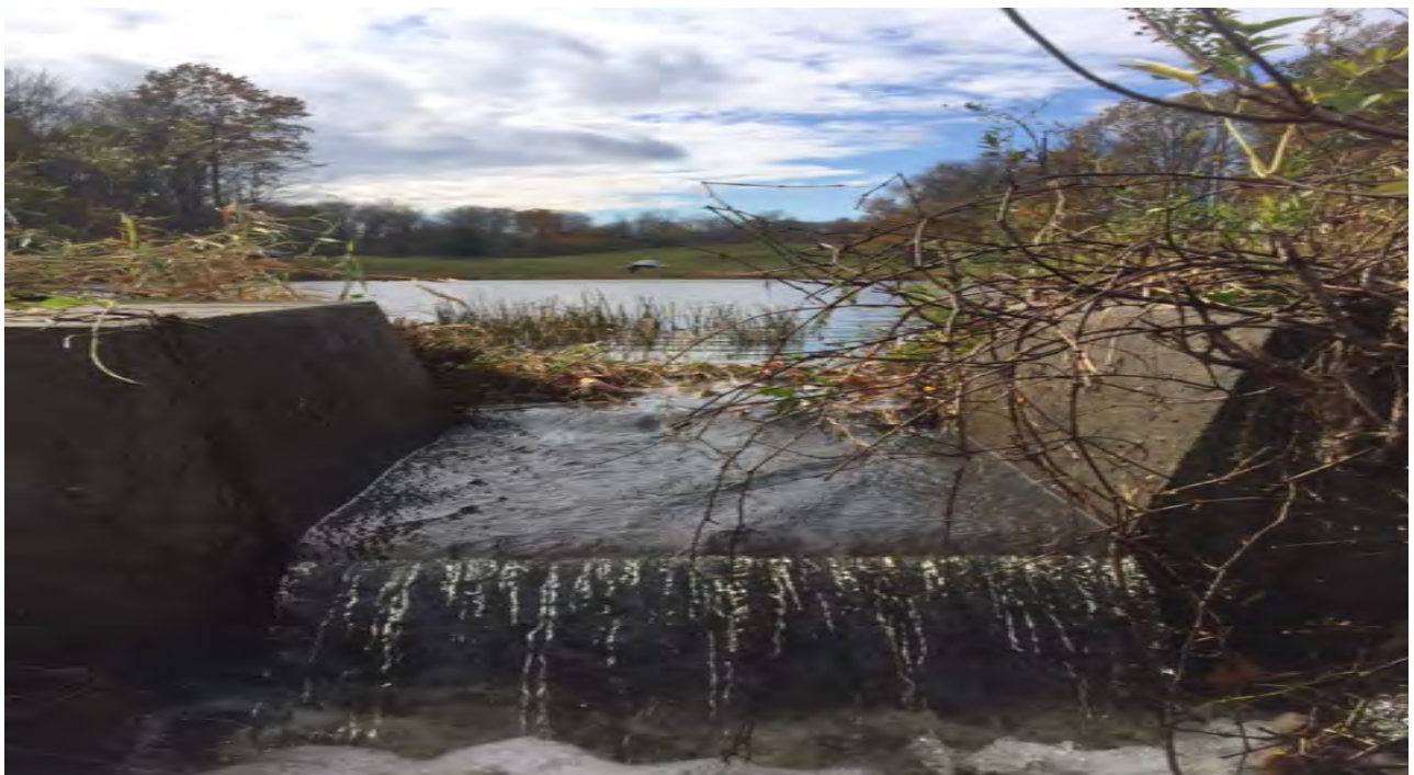
ABP Discharge Structure (cleaned)
