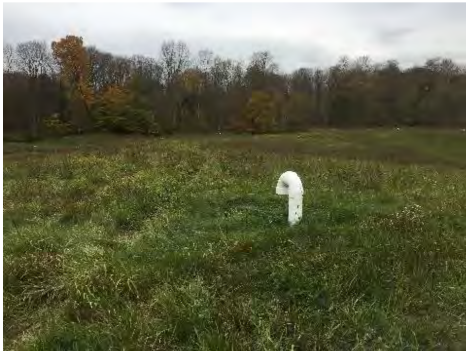
East side of landfill, facing southwest
