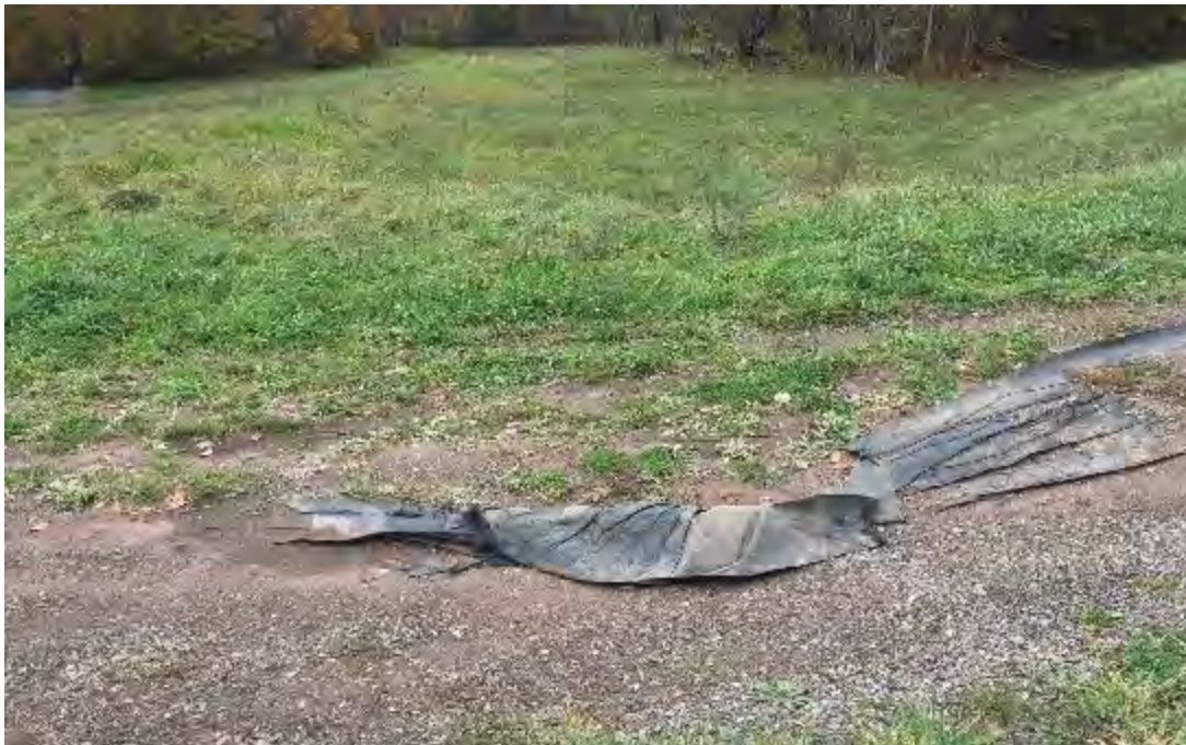
Exposed road fabric for access road
