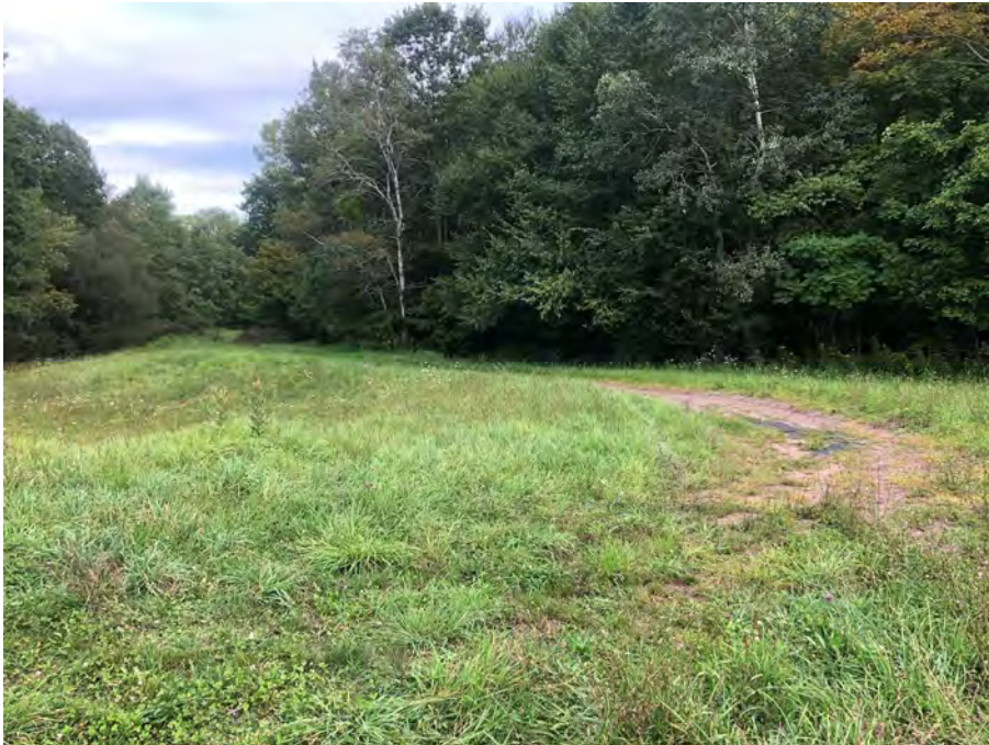
Exposed road fabric on access road
