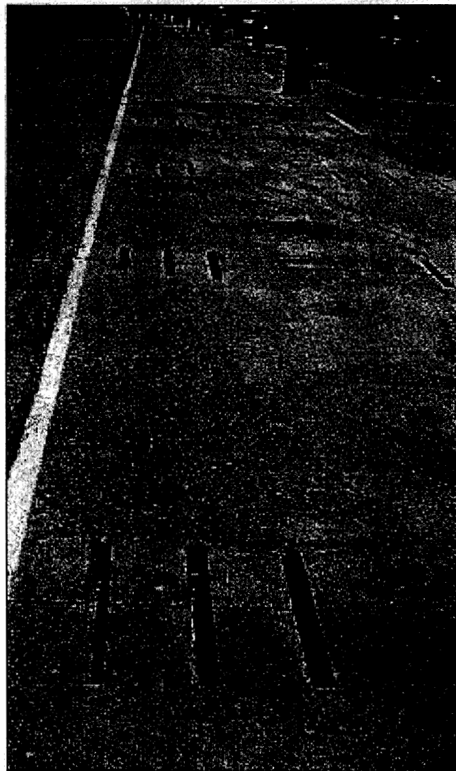
High-production slot cutting has been the driving force behind the renewed interest in dowel bar retrofit.
