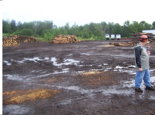
Ponding water on the cap the whole capped area needs to be regraded.
