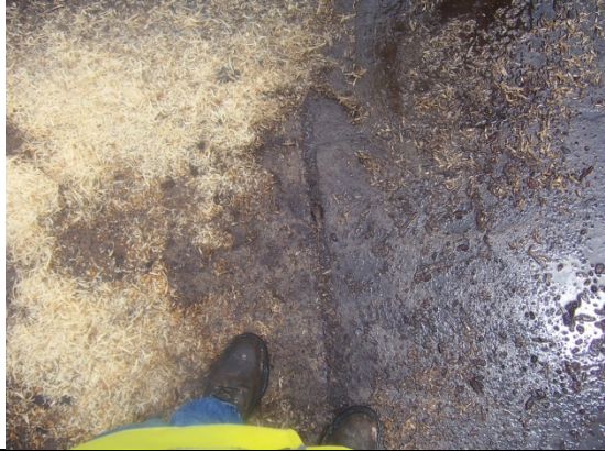
Thin stone cover in the yard. Soil was mixed in with wood chips making the surface was soft.
