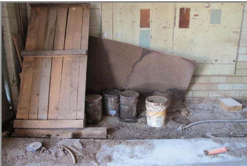
Interior showing waste liquid in containers.
