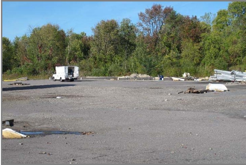
Our DEC sampling van is here parked near MW-3. View looking across the former kiln area.
