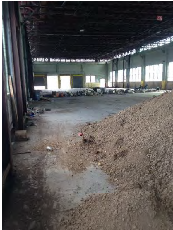
Gravel pile and debris in block building – facing east.
