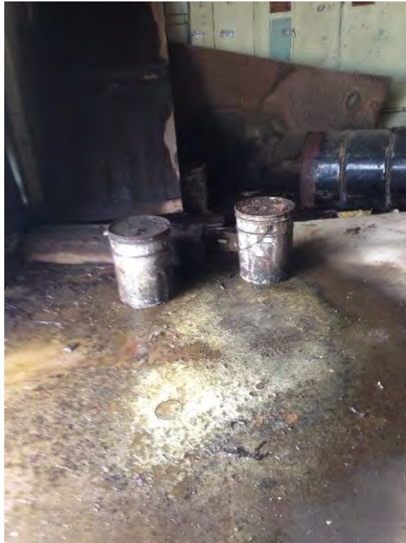
Leaking buckets and drum on north side of block building.
