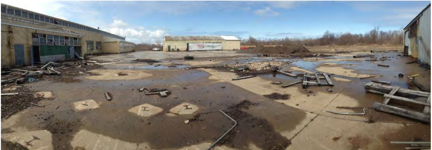
Concrete cap in Yard Area – Panoramic photograph from west to north.
