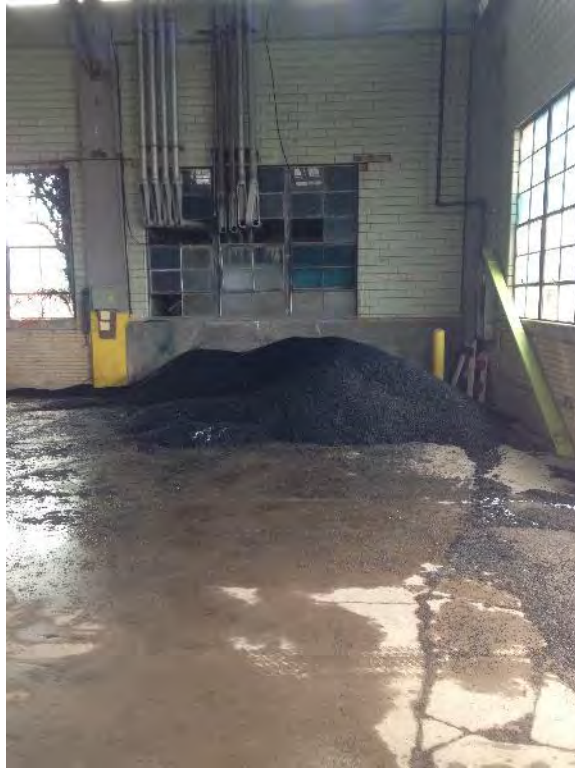
Asphalt pile in southwest corner of block building
