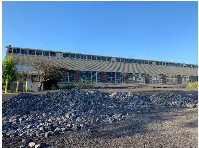
View of eastern silo and buildings. View of stockpiles facing monitoring wells MW-1 and MW-2R.
