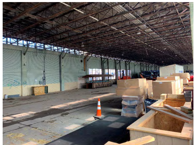
Interior view of onsite building.
