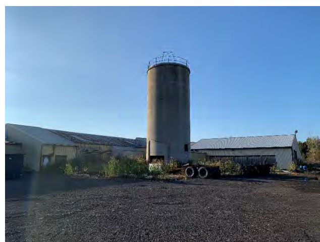
View of eastern silo and buildings.
