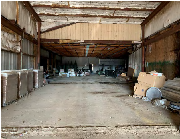
Interior view of northern building.
