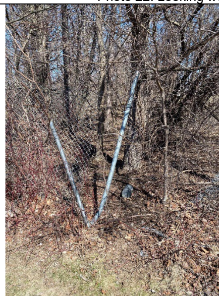
Photo 24: Damaged fence line without secure gate to access MW-6 on southern edge of Site
