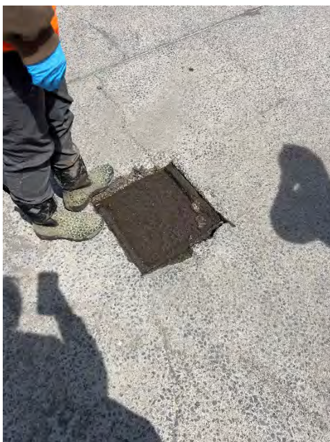
Pooling and hole in concrete cap.
