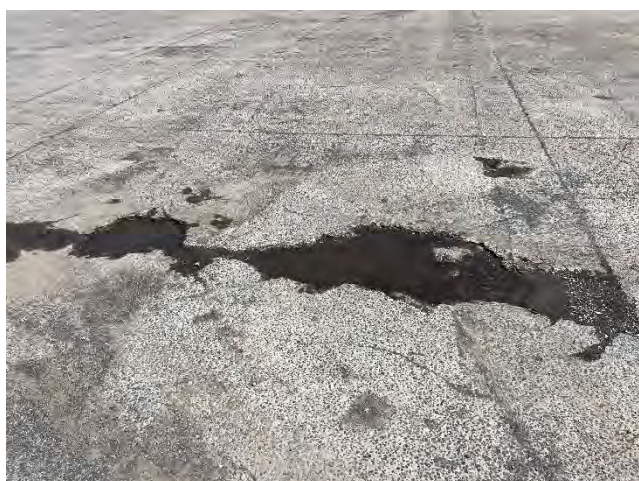
Cracks and pooling in concrete cap.
