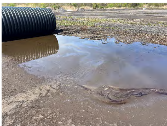
Surface water pooling between concrete cap and soil cap with observed product and sheen.
