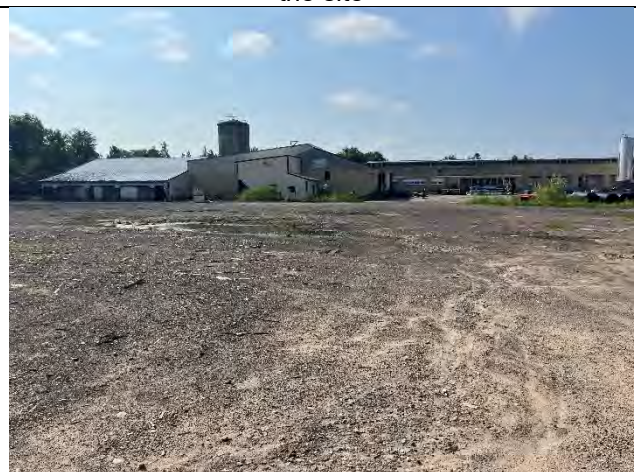
View from northwest quadrante of soft cap looking southeast. Small – medium puddles were observed on the soft cap.
