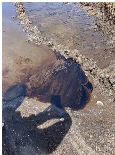
Surface water pooling between concrete cap and soil cap with observed product and sheen.
