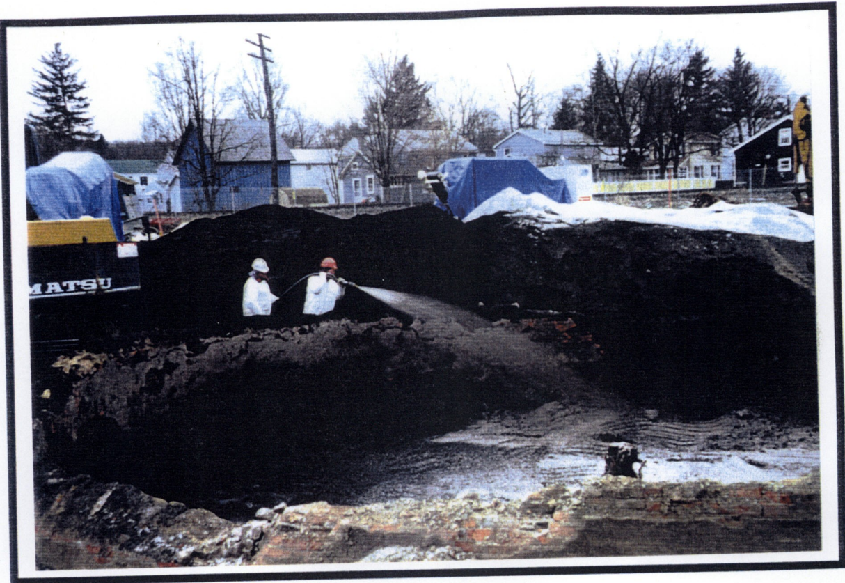
Photograph 5 Application of Con-Cover to control odor.
