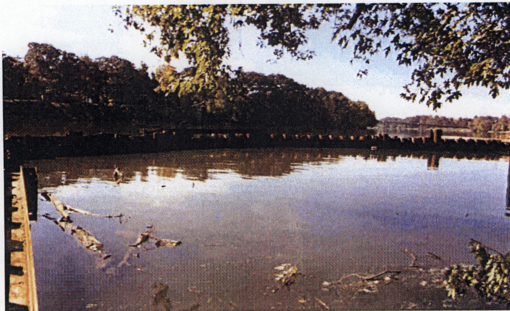
Cofferdam Complete prior to Dewatering
