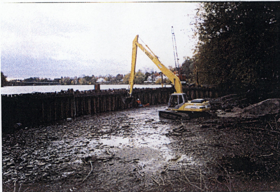
Excavation of River Sediment
