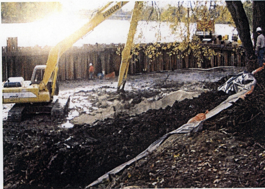
Blending River Sediment and CKD, Temporary Shoreline Staging Area
