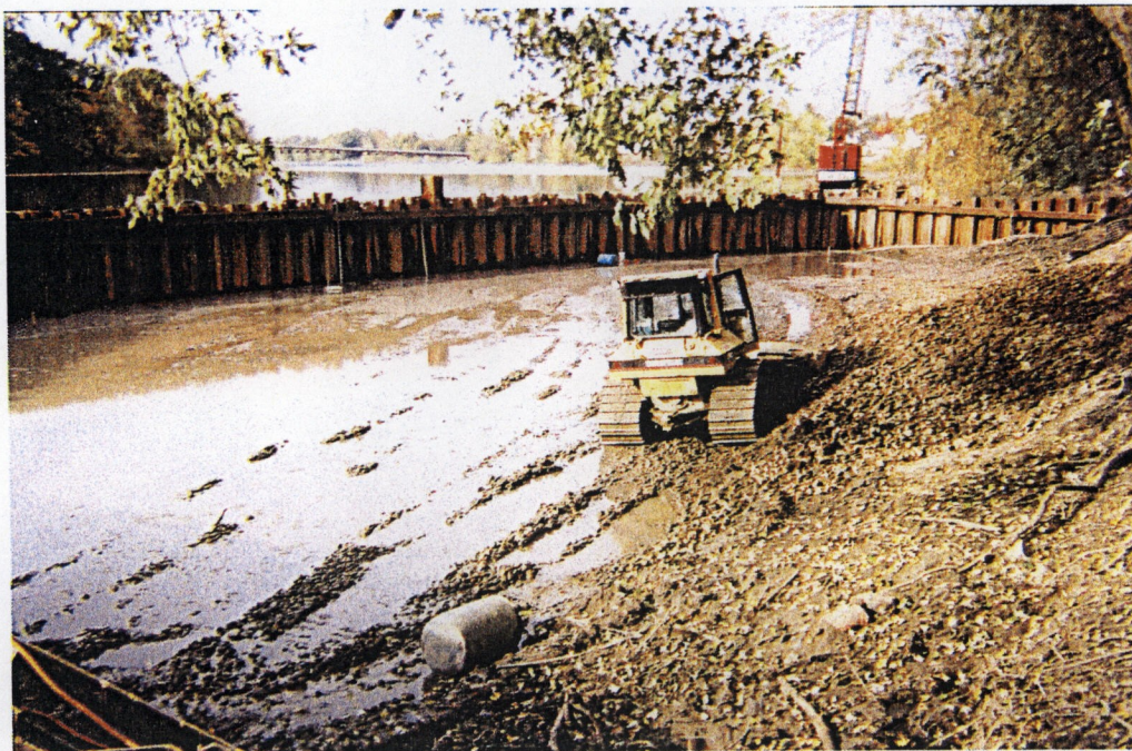
River Bottom Restoration with Cobbles
