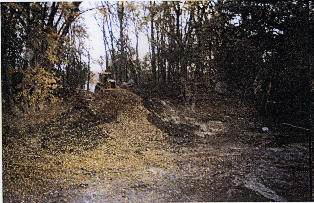
River Bottom Restoration with Cobbles
