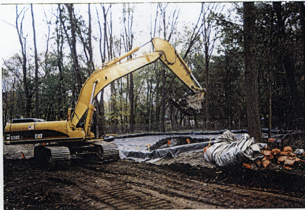
Stockpiling of Stabilized Sediment in Lined Staging Area
