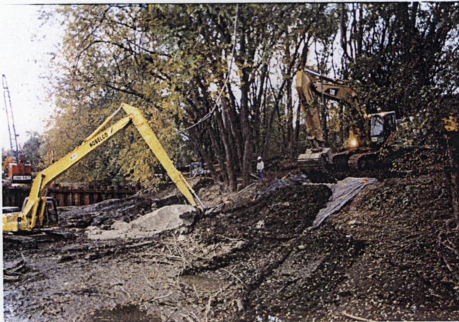
Blending River Sediment with CKD, Removal of Stabilized River Sediment
