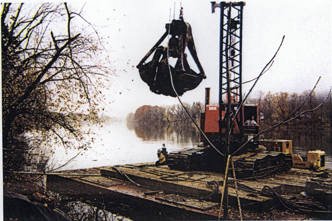
Clamshell Dredging of Impacted Materials at Outlying Areas
