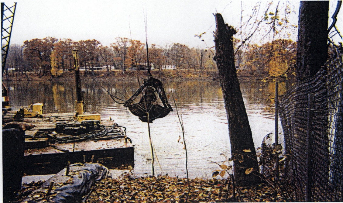
Clamshell Dredging of Impacted Materials at Outlying Areas
