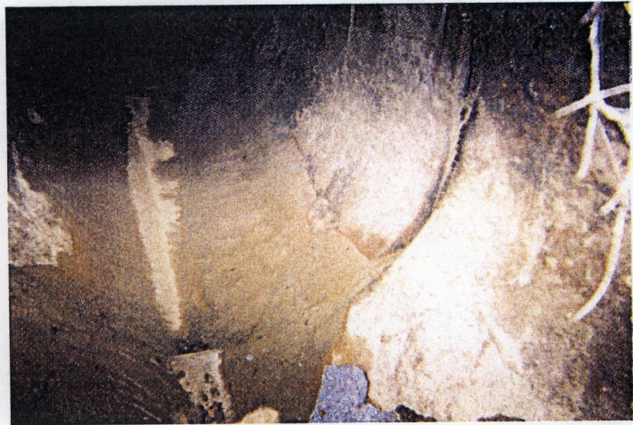
Non-MGP Impacted Termination Point of 24" Diameter Storm Drain
