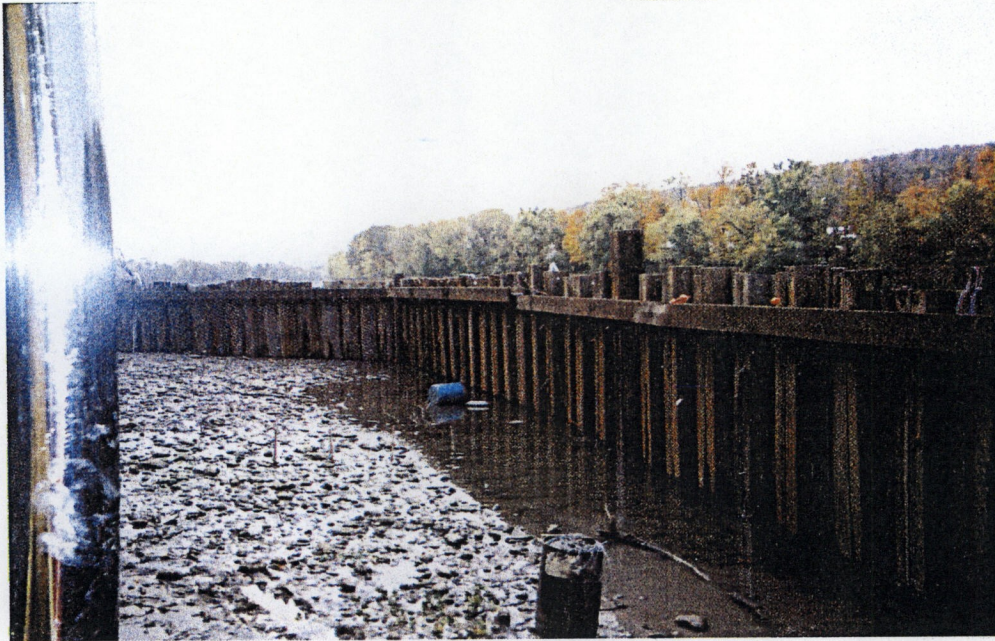
Dewatering within Cofferdam System
