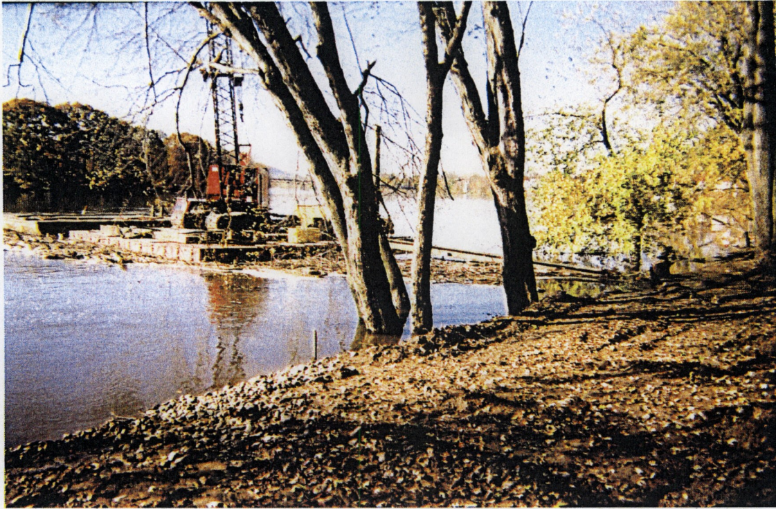
Removal of Cofferdam System
