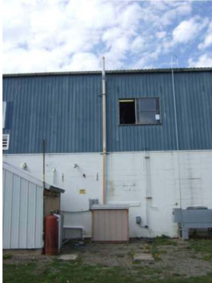
Former effluent piping from VM System with blower.
