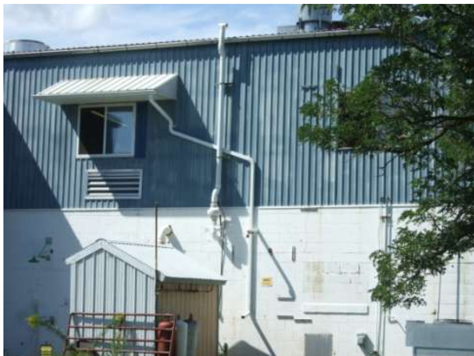
Modified effluent piping with in-line fan.
