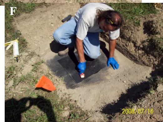
Adhesive caulk was used to seal the perimeter seam of the patch (G).
