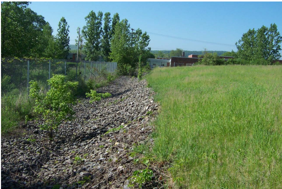
Photograph 3: Trees in drainage swale on east side of landfill, facing south.
