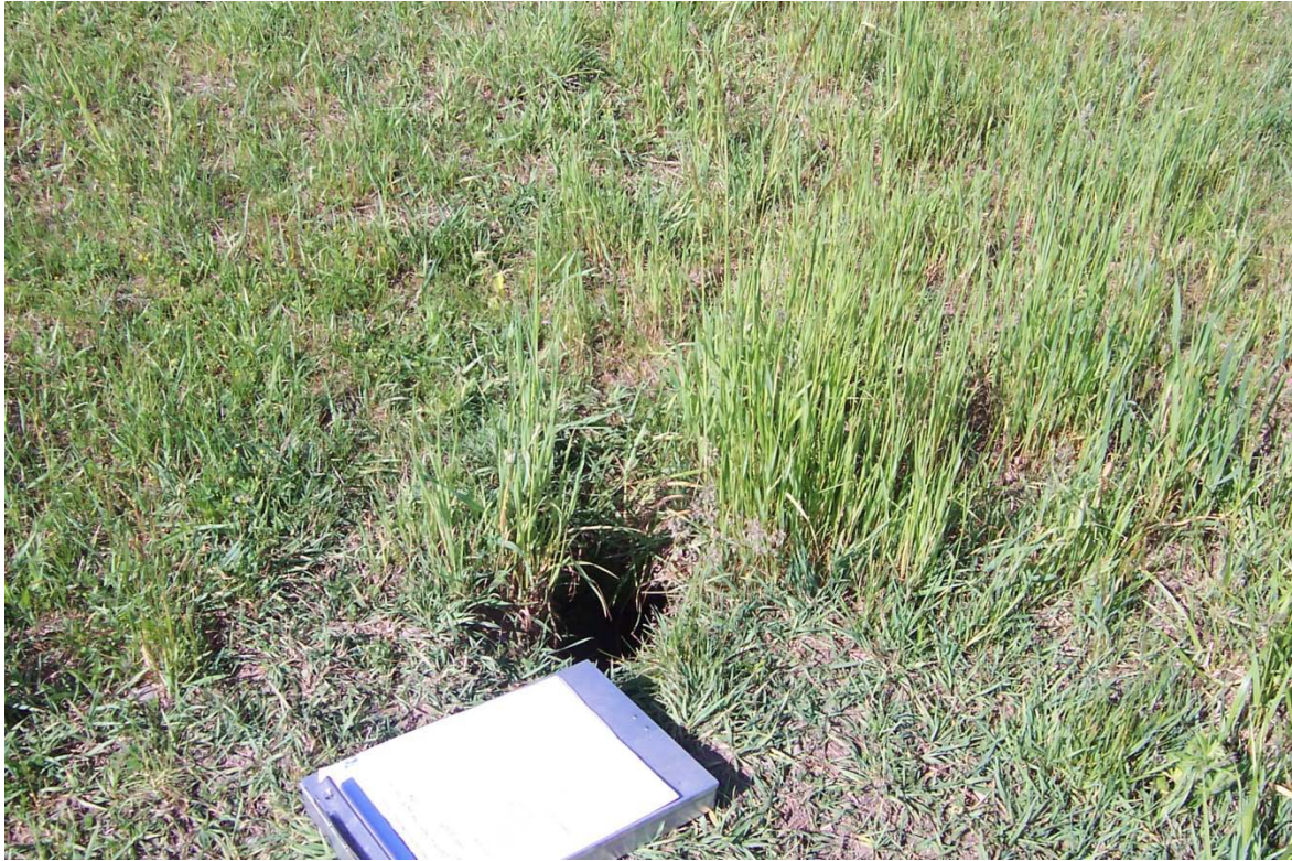
Photograph 1: Burrowing rodent hole on south edge of landfill cap.
