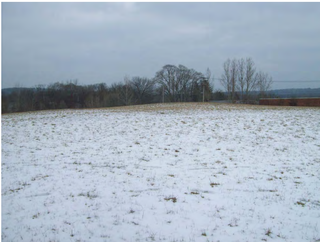
Photograph 4: Landfill cap from northwest corner, facing southeast.
