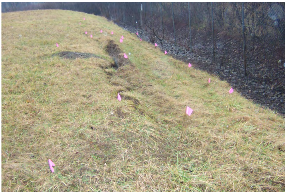
Photograph 1: Damage to cap along north end of landfill, facing west.
