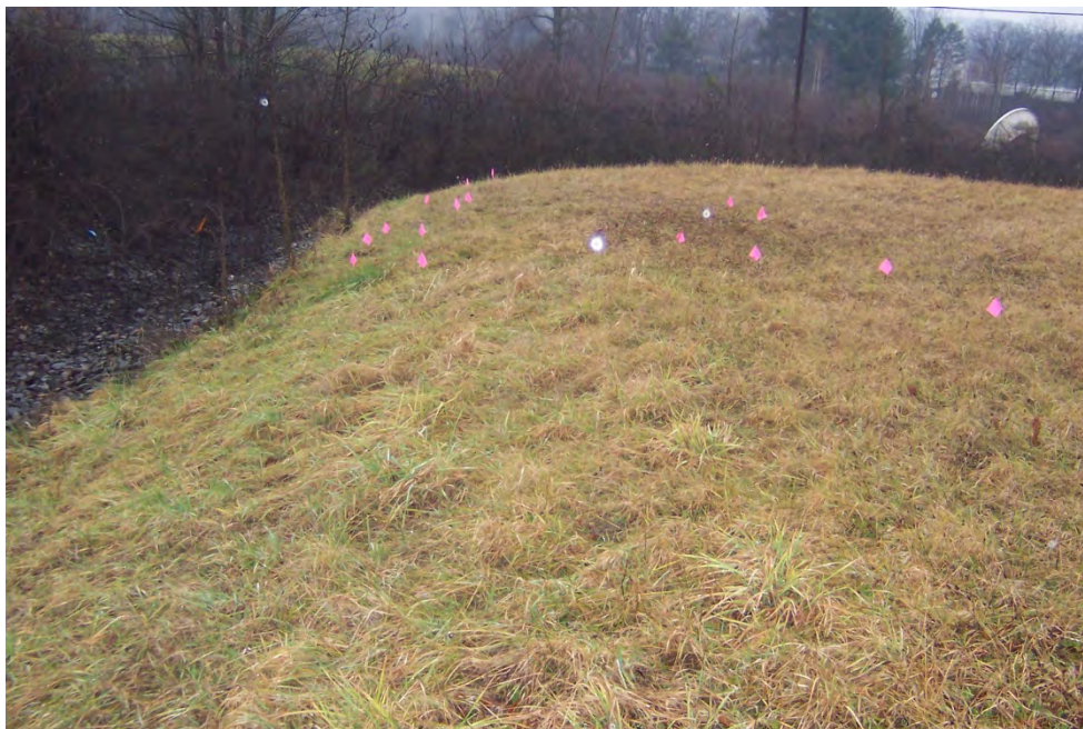
Photograph 2: Soil failure along south end of landfill, facing west.
