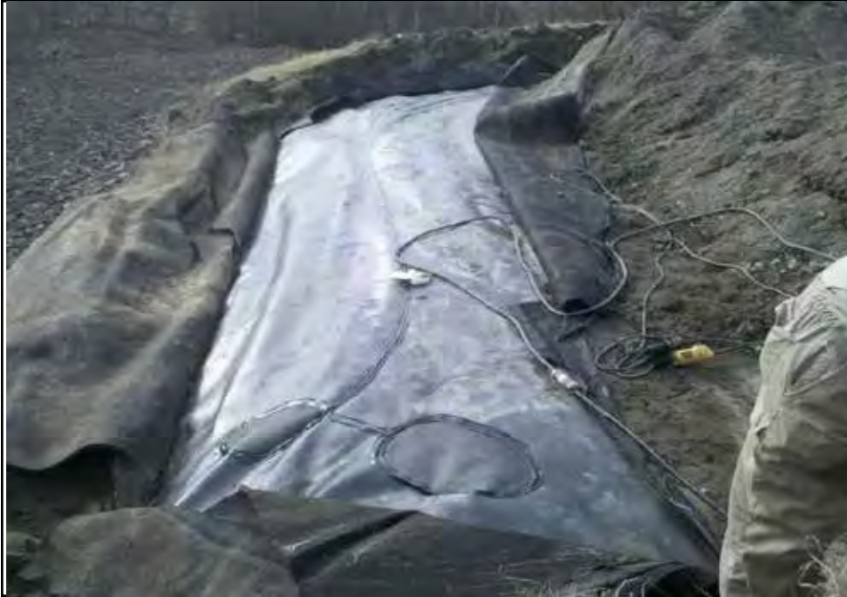
Finished liner repair. Folds and wrinkles removed.
