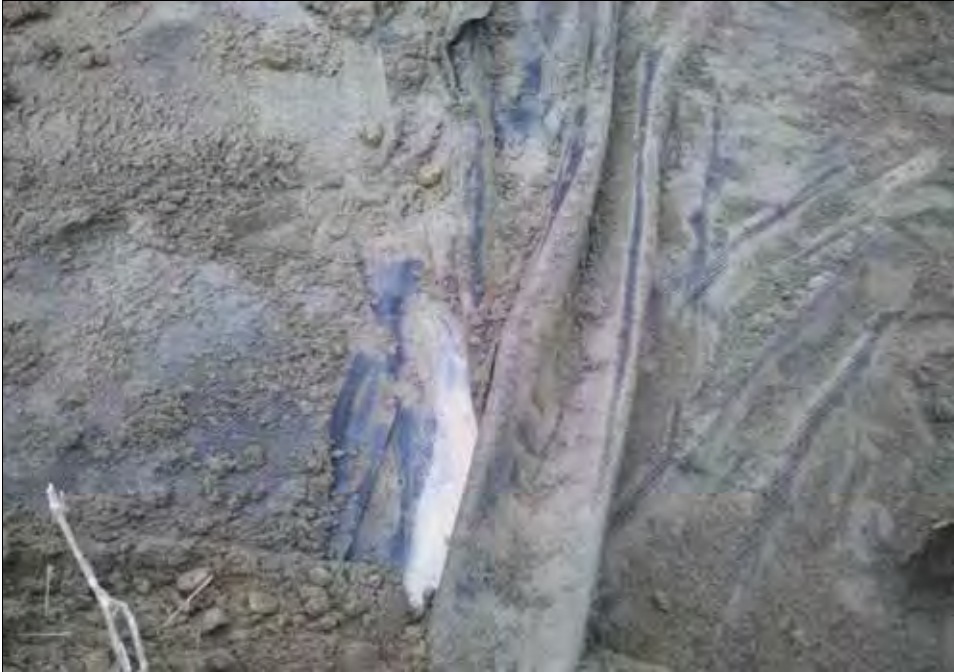
Liner fold in the northeast area.
