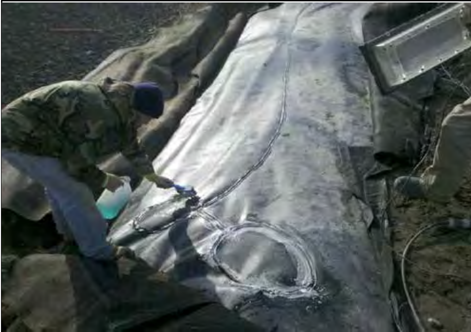
Vacuum testing of liner weld. No leaks found.
