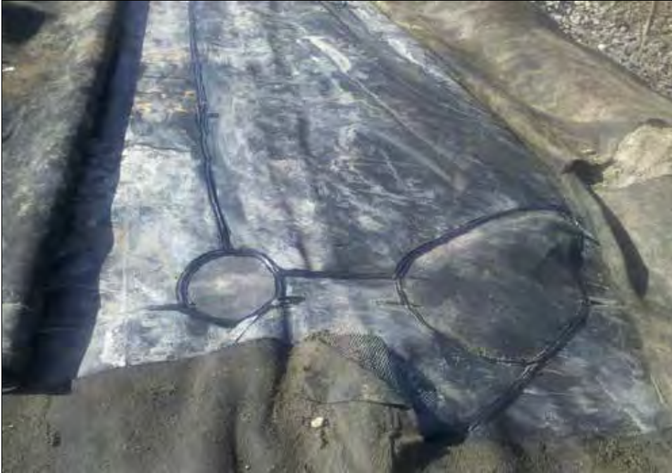
Finished patches and welds.
