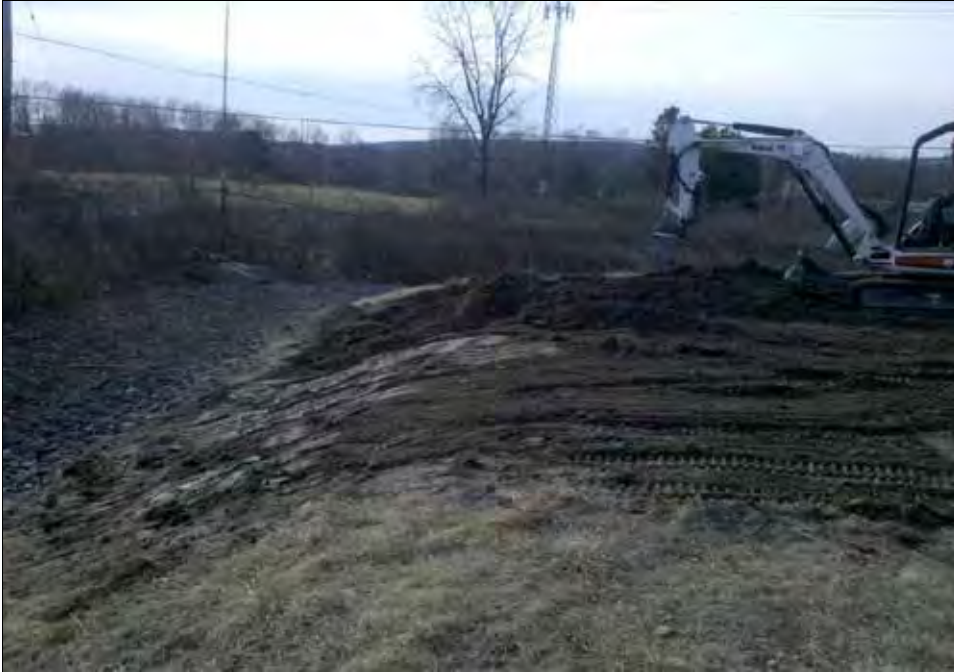
Backfilling repair areas.
