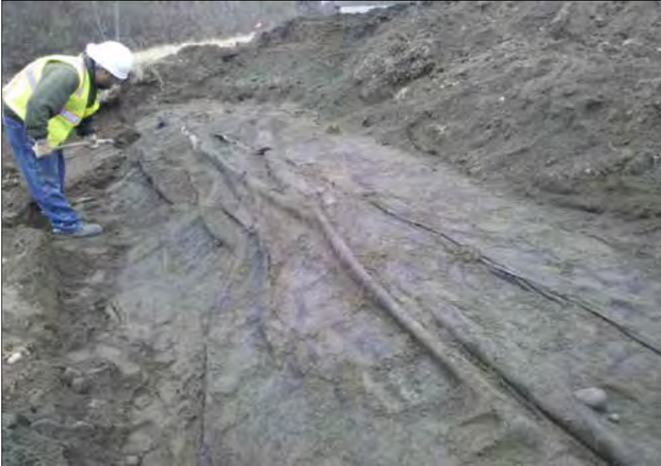
Inspecting fabric and liner.
