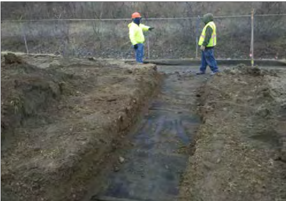
Exploratory trench extending towards the center of the landfill. No visible damage to fabric seams or liner.
