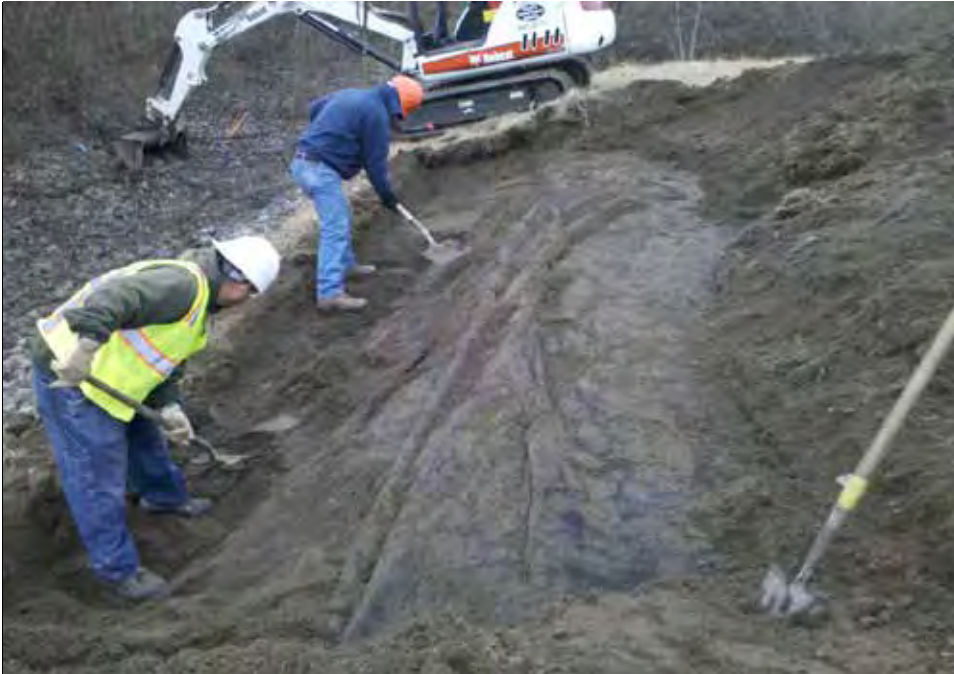
Aztech uncovers damaged area in southwest corner. Soil removed by hand to avoid damaging fabric or liner.
