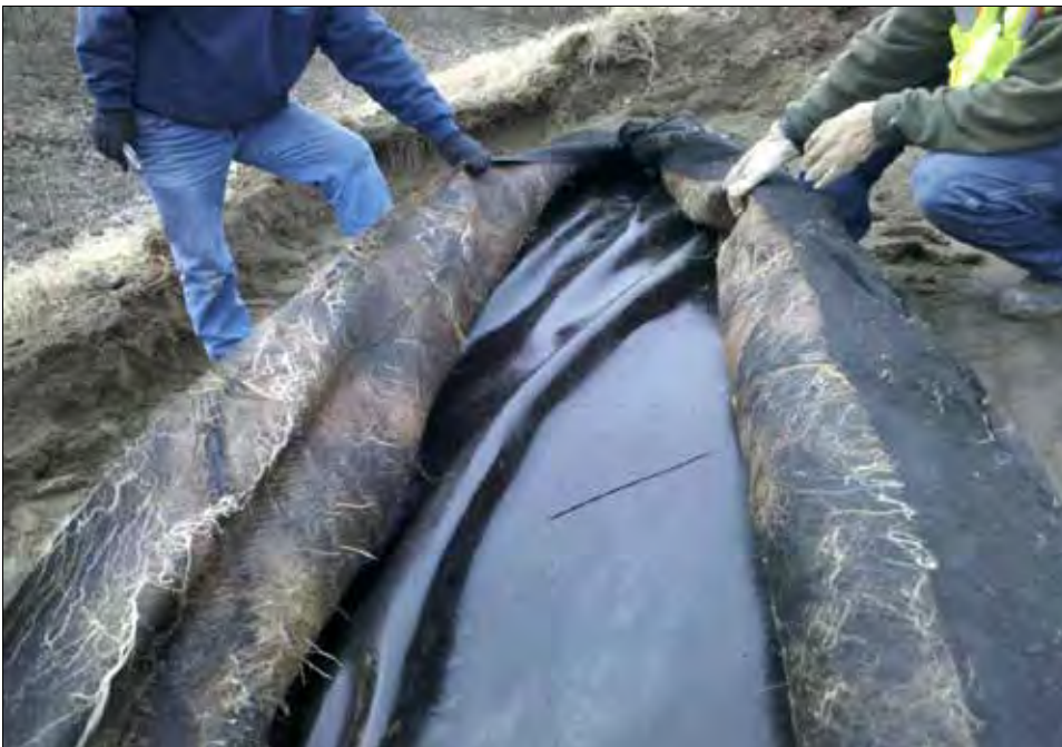
The exposed liner with wrinkles.
