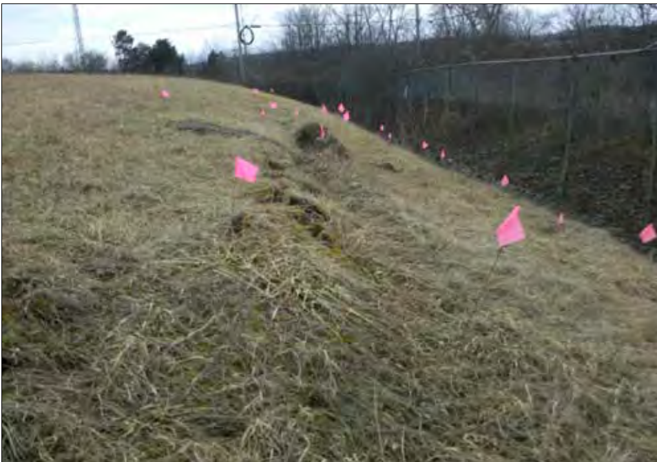
Liner visibly protruding through surface material.
