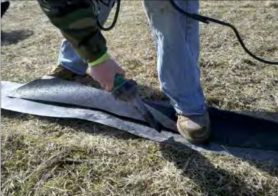
Preparing liner weld test strip.
