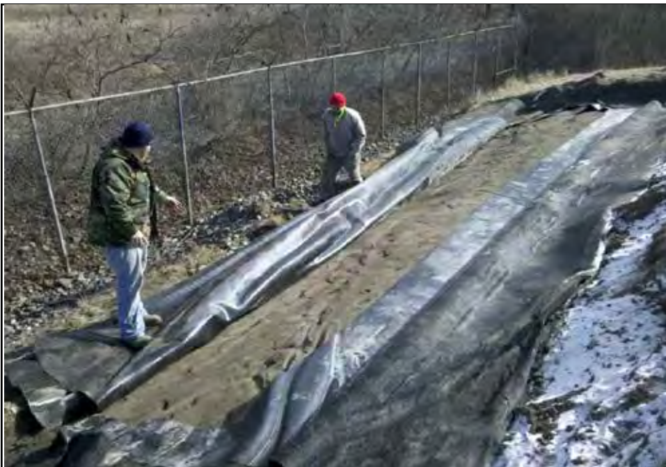
The liner is cut and slack removed.
