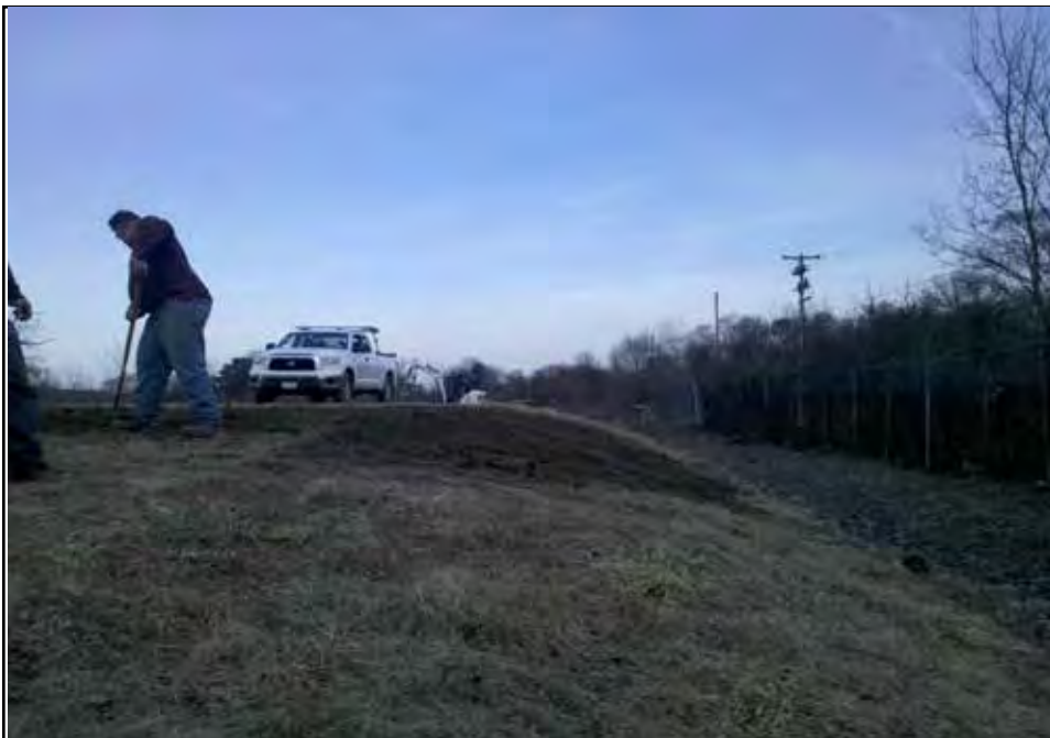
Rake and seed backfilled areas.
