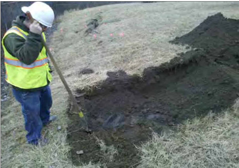
Aztech exposing liner with hand tools.
