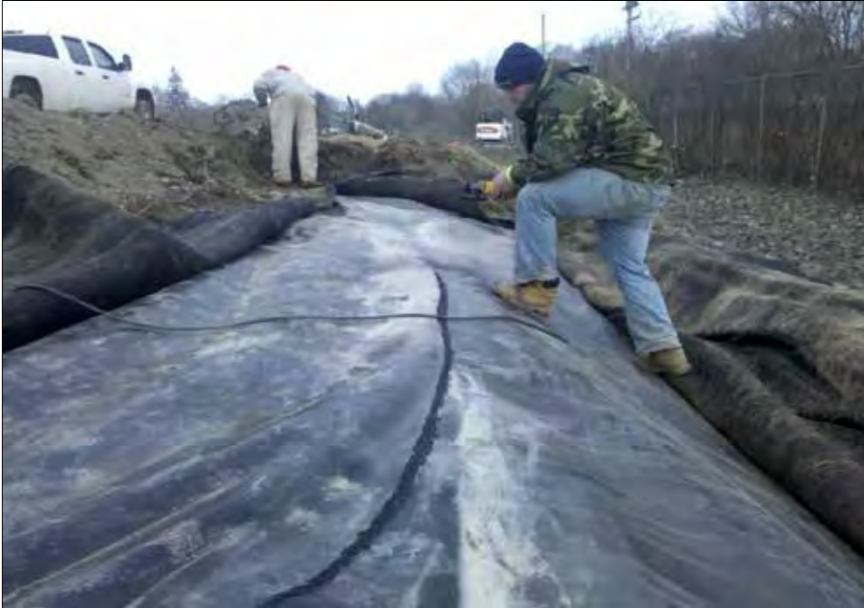
Grinding new seam in northeast area.
