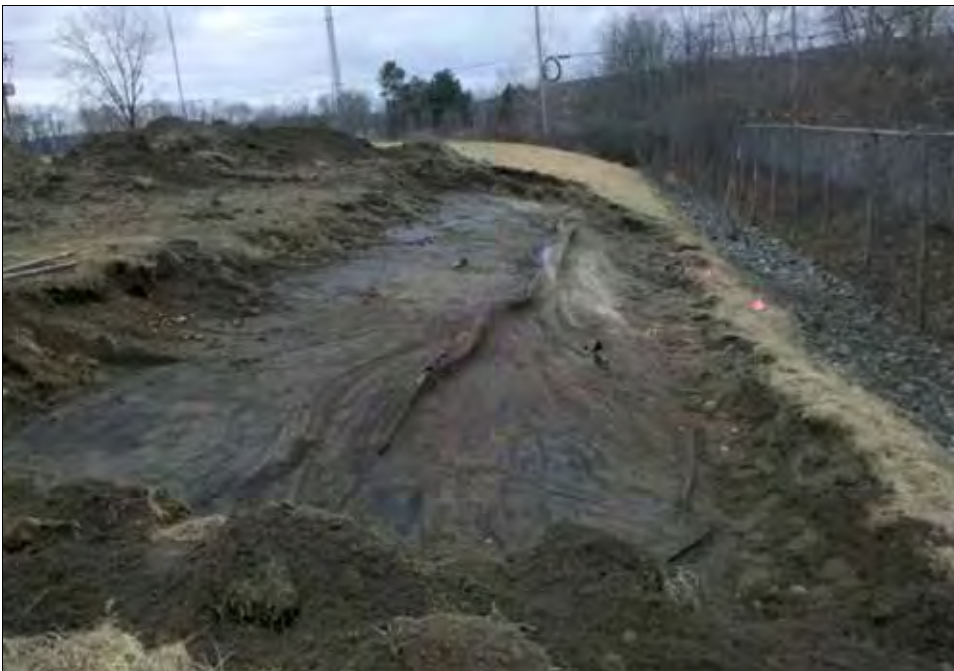
Liner fold extends approximately 50'.
