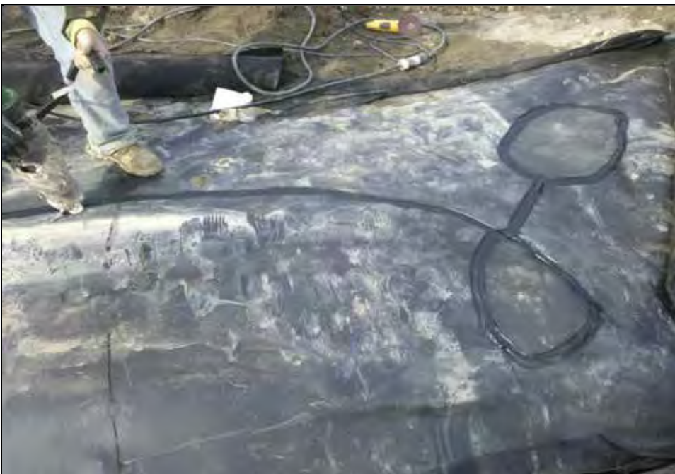
Extrusion welding new seam in the northwest area.
