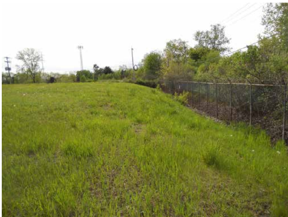
North side of landfill – looking west.
