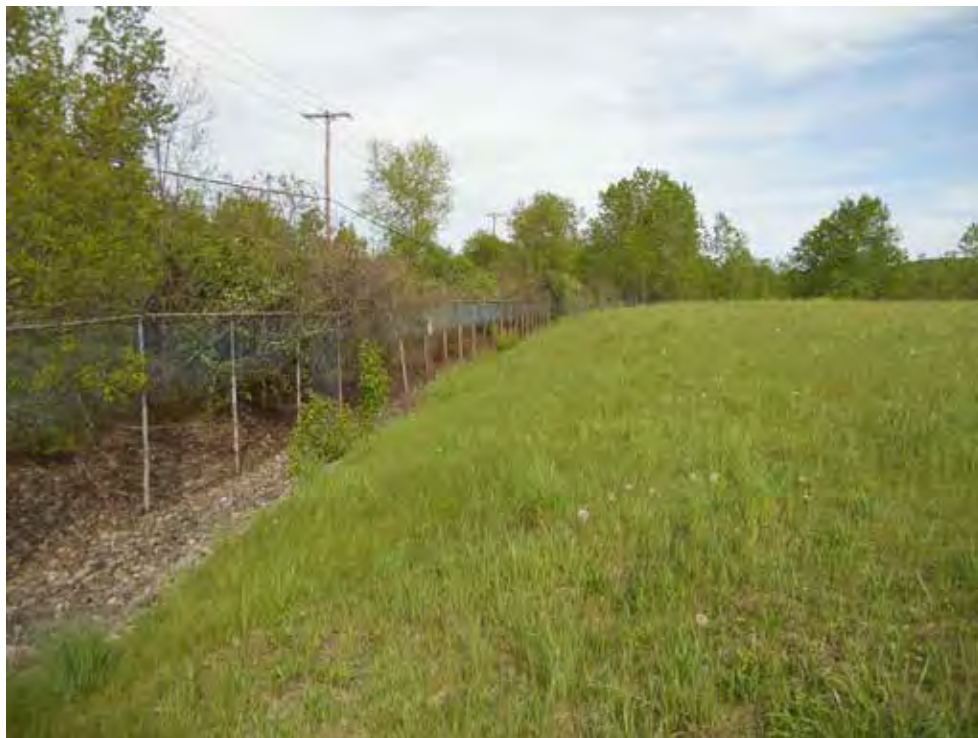
North side of landfill – looking east.
