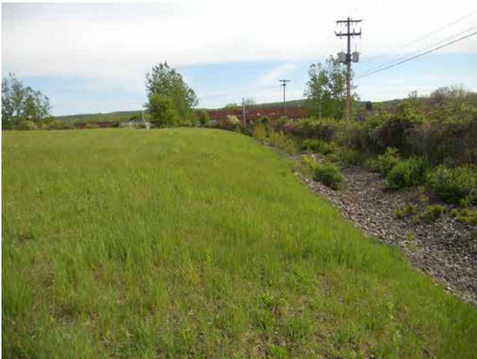
West side of landfill – looking south.
