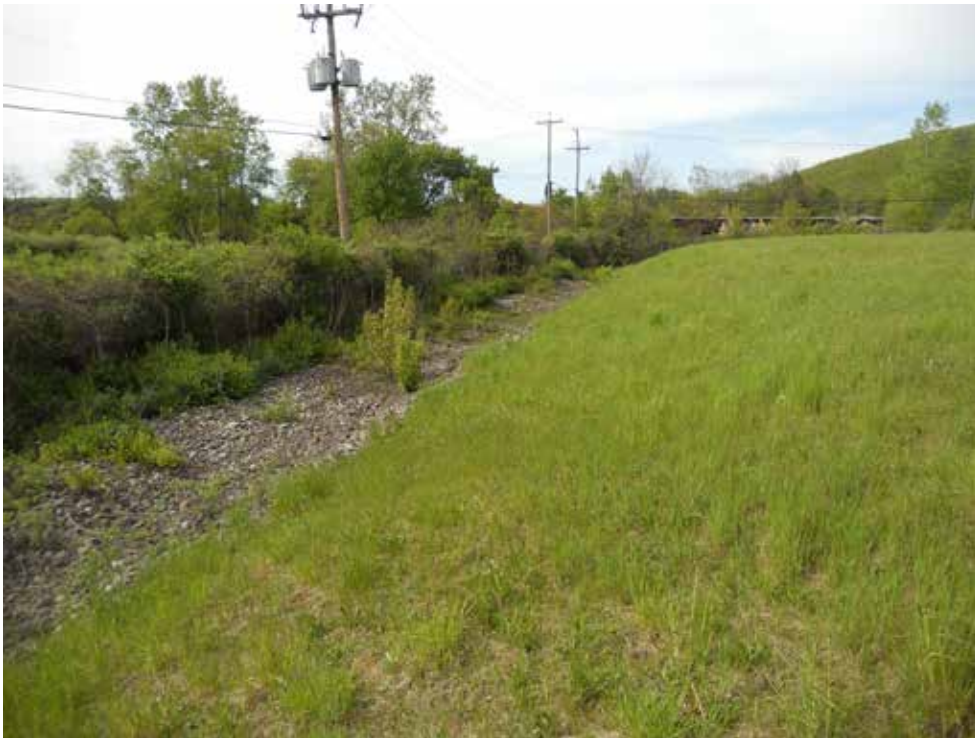
West side of landfill – looking north.
