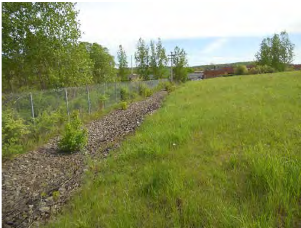
East side of landfill – looking south.
