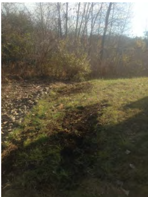
Northeast corner of landfill – facing east (11/10/14) following repairs
