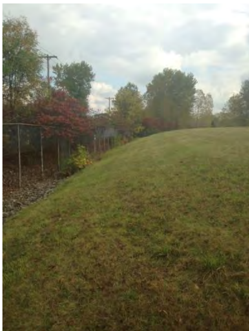
North side of landfill – facing east
