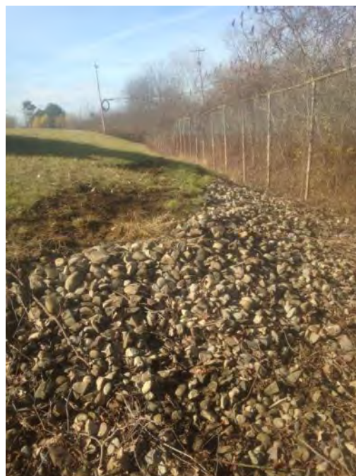
Northeast corner of landfill – facing west (11/10/14) following repairs
