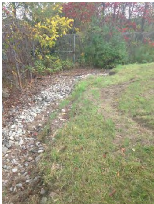
Northeast corner of landfill – facing east (10/1/14) Ruts visible from mower.
