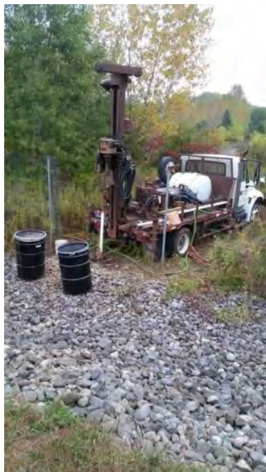
Drill rig set up at MW-9
