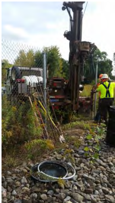
Parratt Wolff installing MW-9
