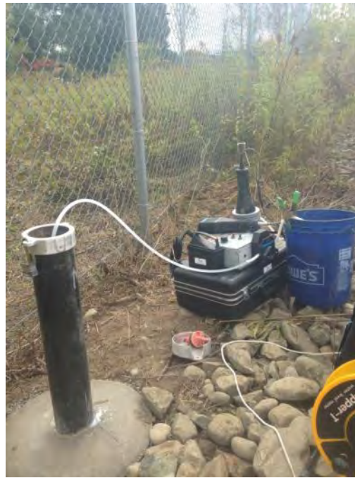
Well developing at MW-9
