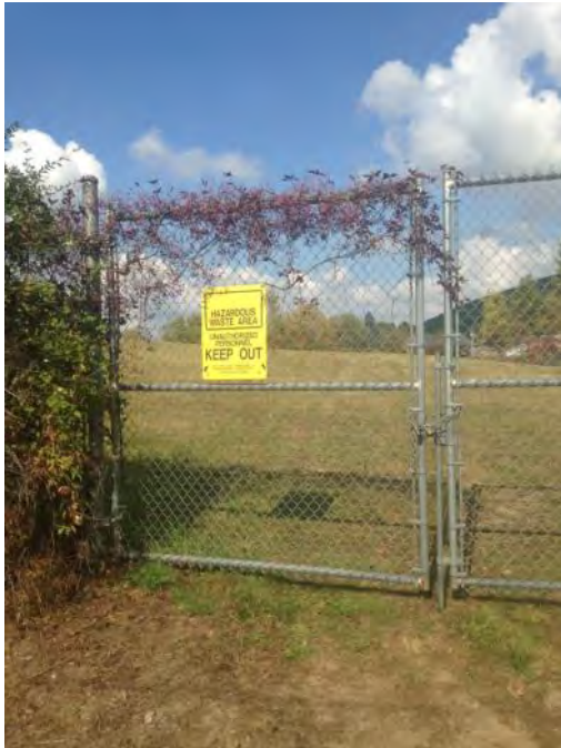
Landfill access gate
