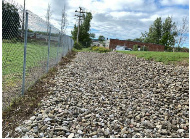
Photo 2: View of the drainage swale on the east portion of the site, which was dry during inspection activities. Looking south.
