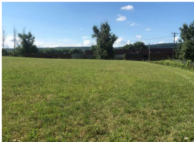
Photo 3: View looking south. Overview of the landfill cap.
