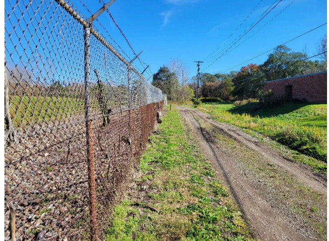
Photo 2: Looking east along the site boundary.
