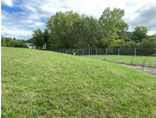
Photo 1: Overview of the east side of the landfill cap, facing north.
