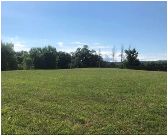
Photo 5: Looking southwest. Overview of the landfill cap.
