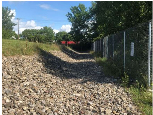
Photo 2: View looking north. Looking at the drainage trench located on the eastern boundary of the on-site landfill
