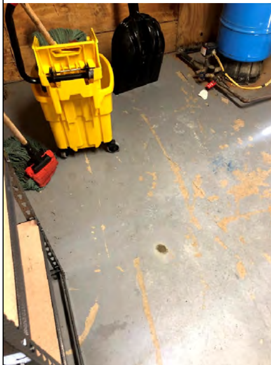
Vapor point from 754020-SV-1-2182024 after concreting (Structure 1)
