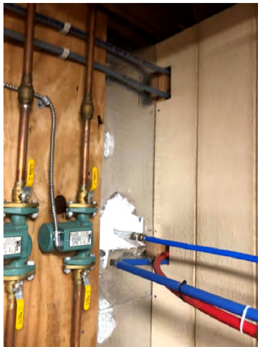
Holes in walls for plumbing at Structure 1
