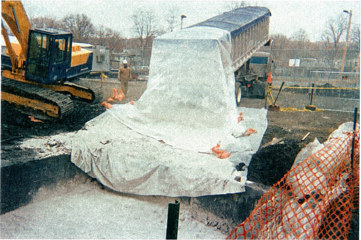
ITHACA COURT STREET FORMER MANUFACTURED GAS PLANT 2000 REMEDIATION PROJECT PHOTO NUMBER 9
