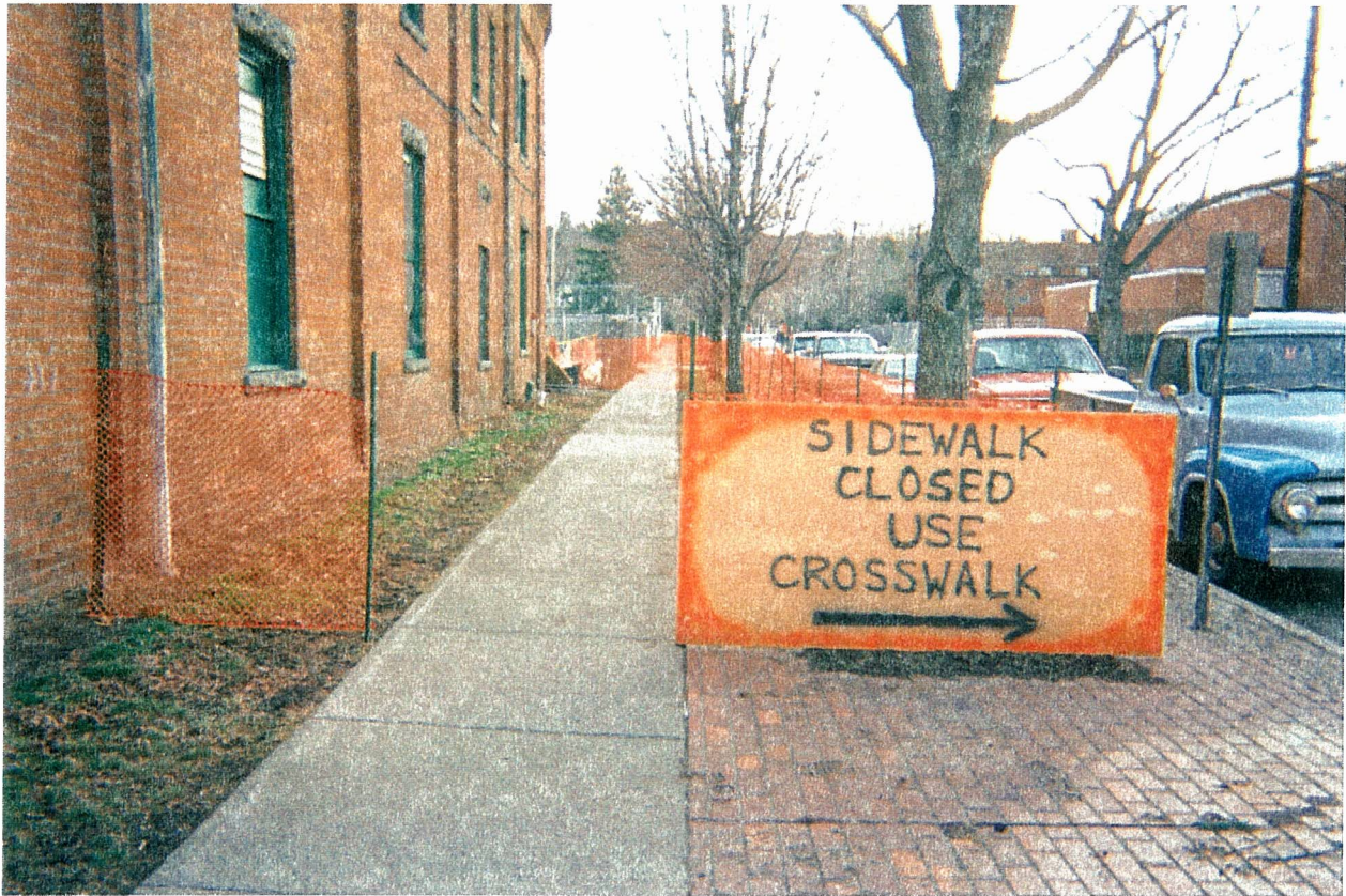
ITHACA COURT STREET FORMER MANUFACTURED GAS PLANT 2000 REMEDIATION PROJECT PHOTO NUMBER 1
