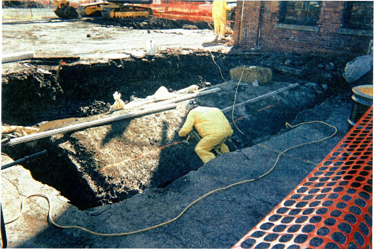
ITHACA COURT STREET FORMER MANUFACTURED GAS PLANT 2000 REMEDIATION PROJECT PHOTO NUMBER 4
