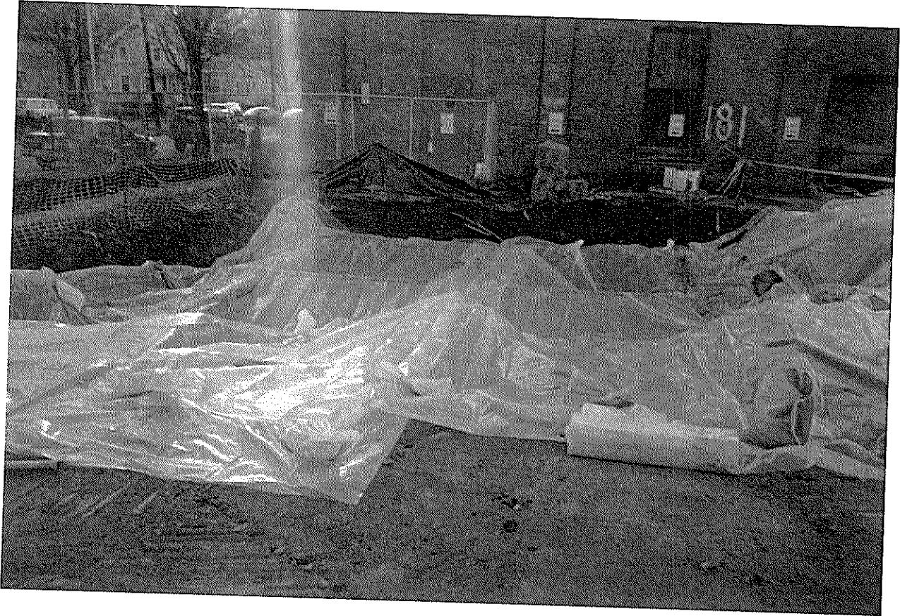
ITHACA COURT STREET FORMER MANUFACTURED GAS PLANT 2000 REMEDIATION PROJECT PHOTO NUMBER 8
