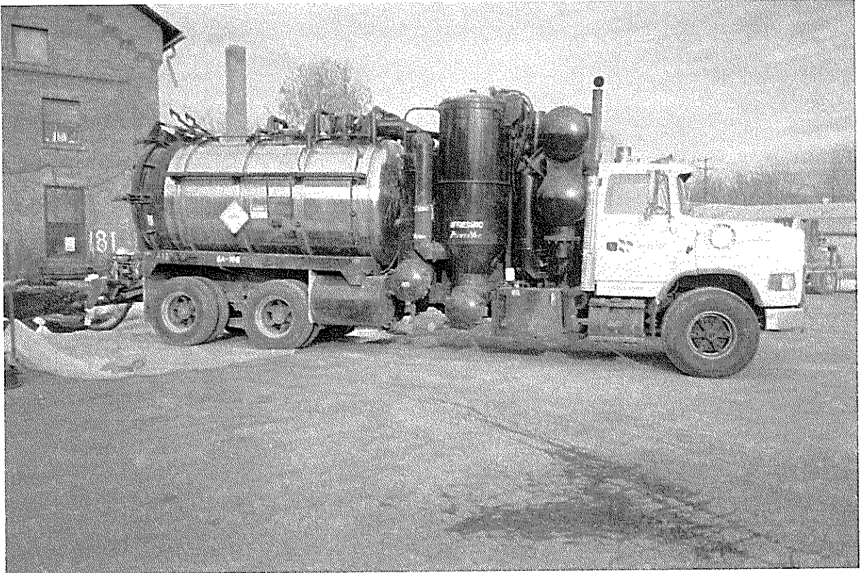
ITHACA COURT STREET FORMER MANUFACTURED GAS PLANT 2000 REMEDIATION PROJECT PHOTO NUMBER 2
