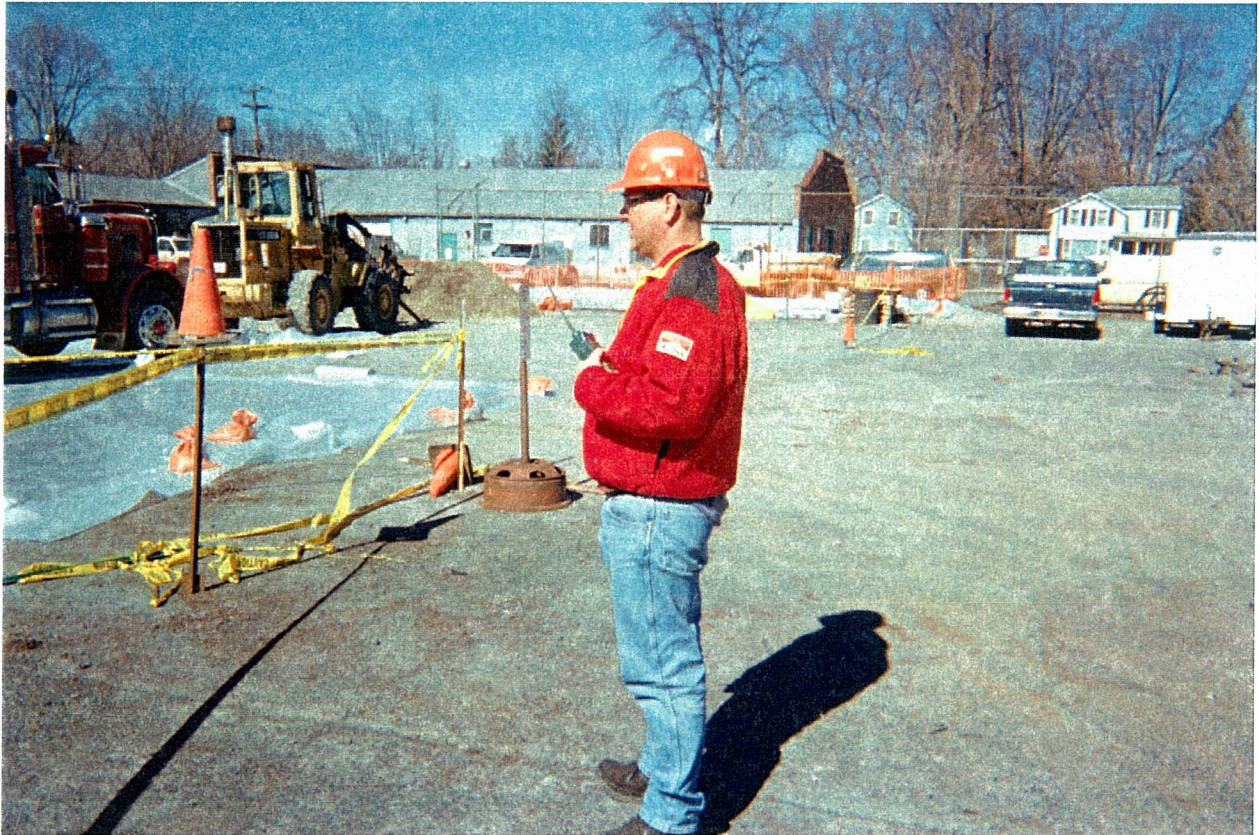
ITHACA COURT STREET FORMER MANUFACTURED GAS PLANT 2000 REMEDIATION PROJECT PHOTO NUMBER 3
