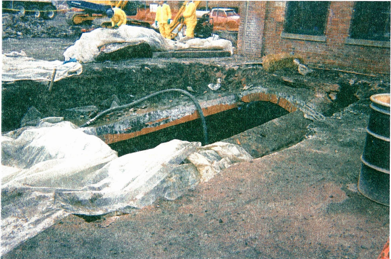
ITHACA COURT STREET FORMER MANUFACTURED GAS PLANT 2000 REMEDIATION PROJECT PHOTO NUMBER 5
