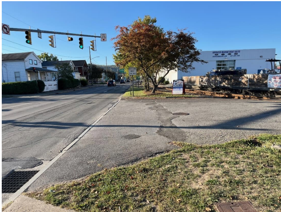
Wooden Duct IRM area along West Fulton Street facing south.
