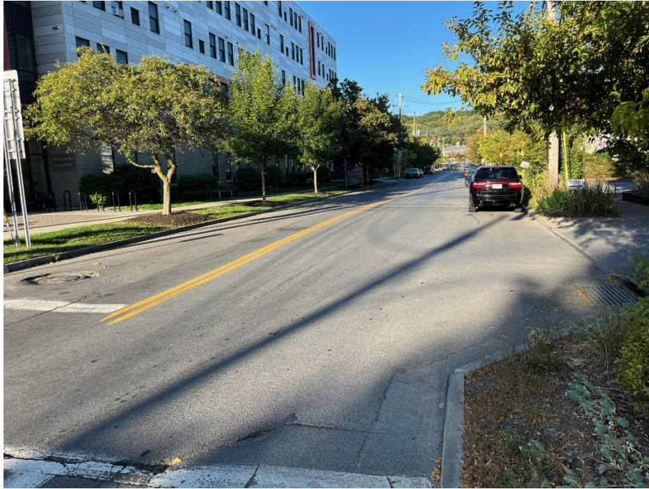
West Court Street from Meadow Street facing west.
