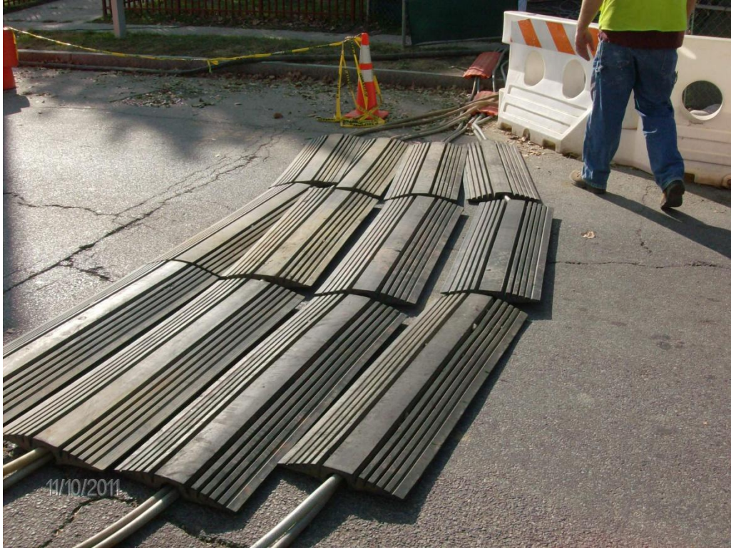
Photograph 3 – Close up view of hose ramps used in the street.
