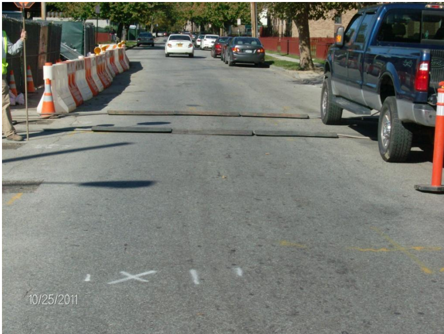
Photograph 2 – Hose ramps were used in the street to protect hoses from passing traffic.
