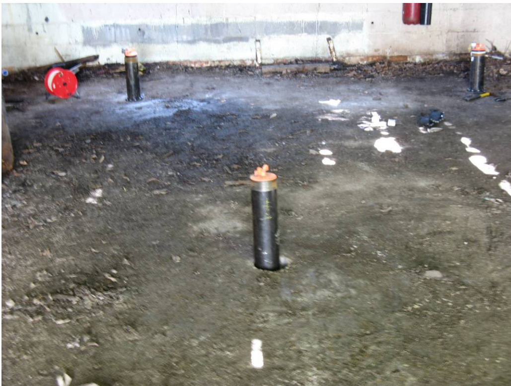
Monitoring Points 2, 3, and 4 located along west wall of south tank
