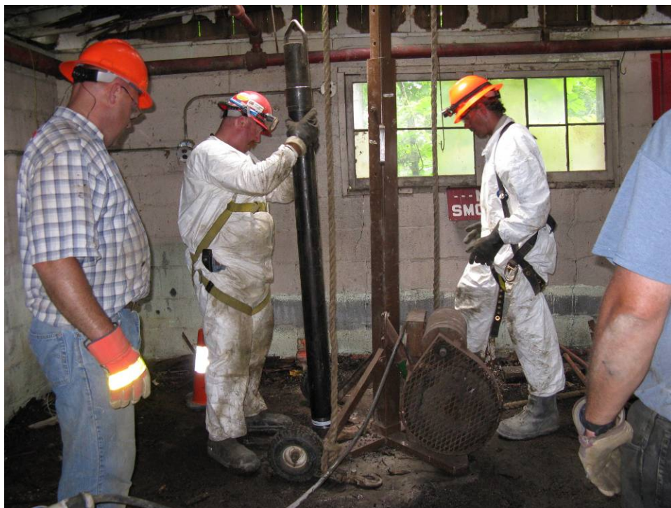
4" steel casing installation using portable cat-head
