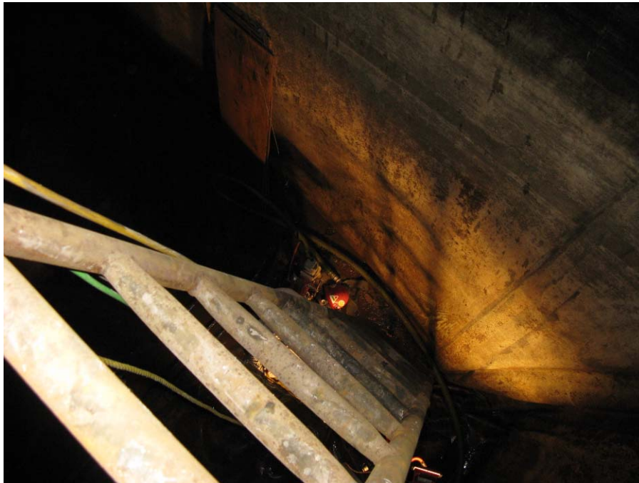
Fire Water Reservoir – Entering South Tank
