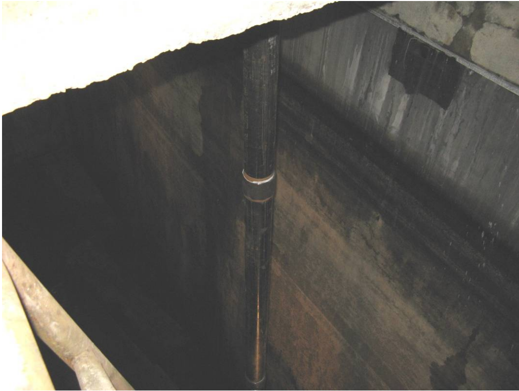
Installed casing for Monitoring Point 1
