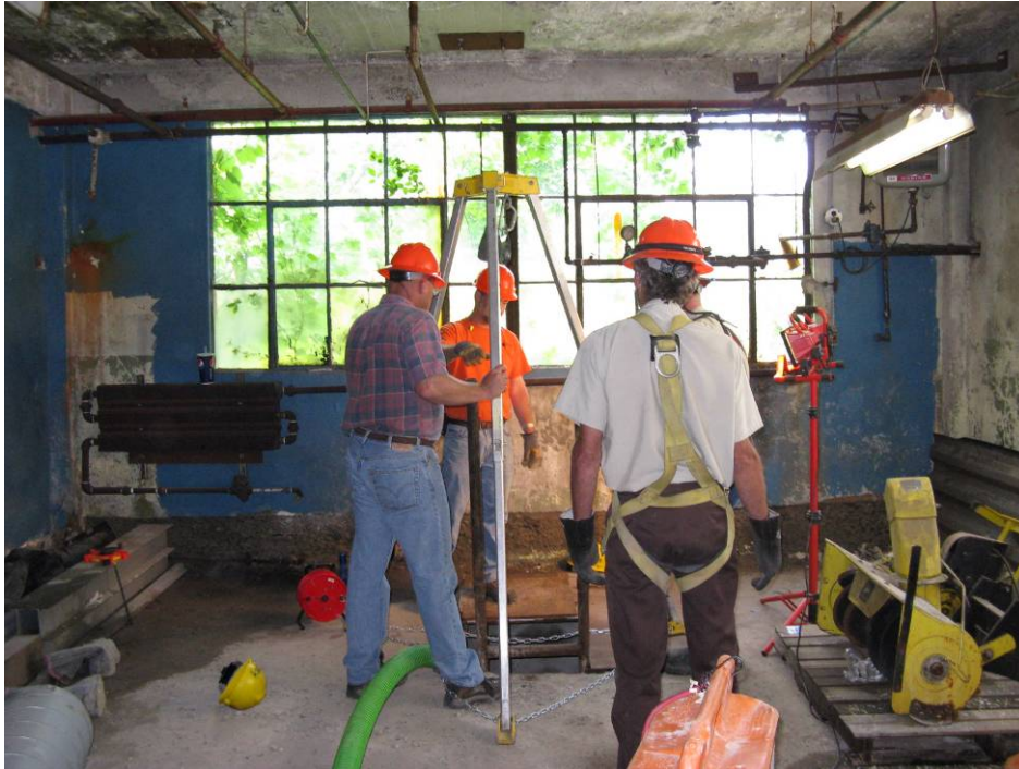
Permitted Confined Space Entry – South Tank
