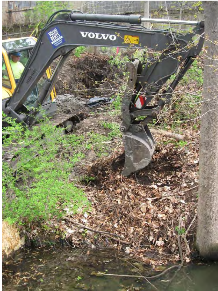
Photograph 28: Test pit installed to find the end of the pipe near the drainage ditch.
