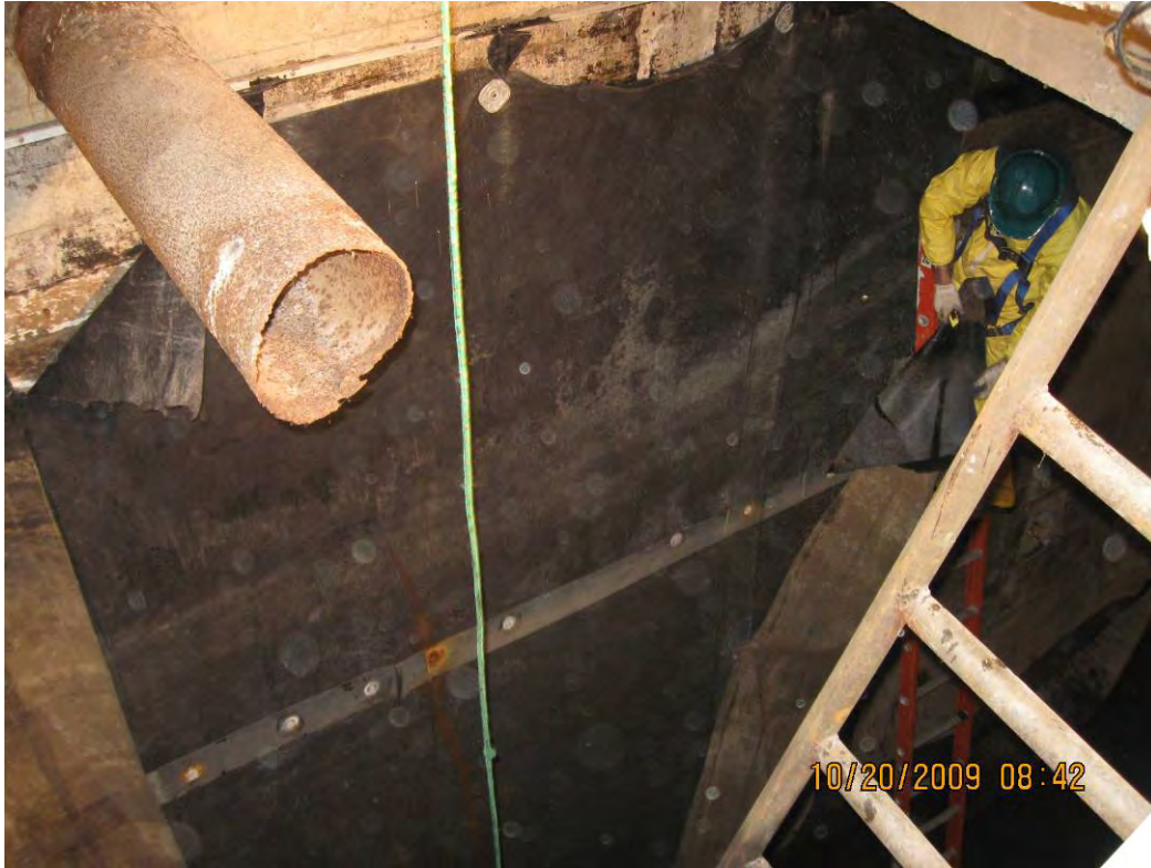
Photograph 3: Removing the EPDM liner inside the south tank.
