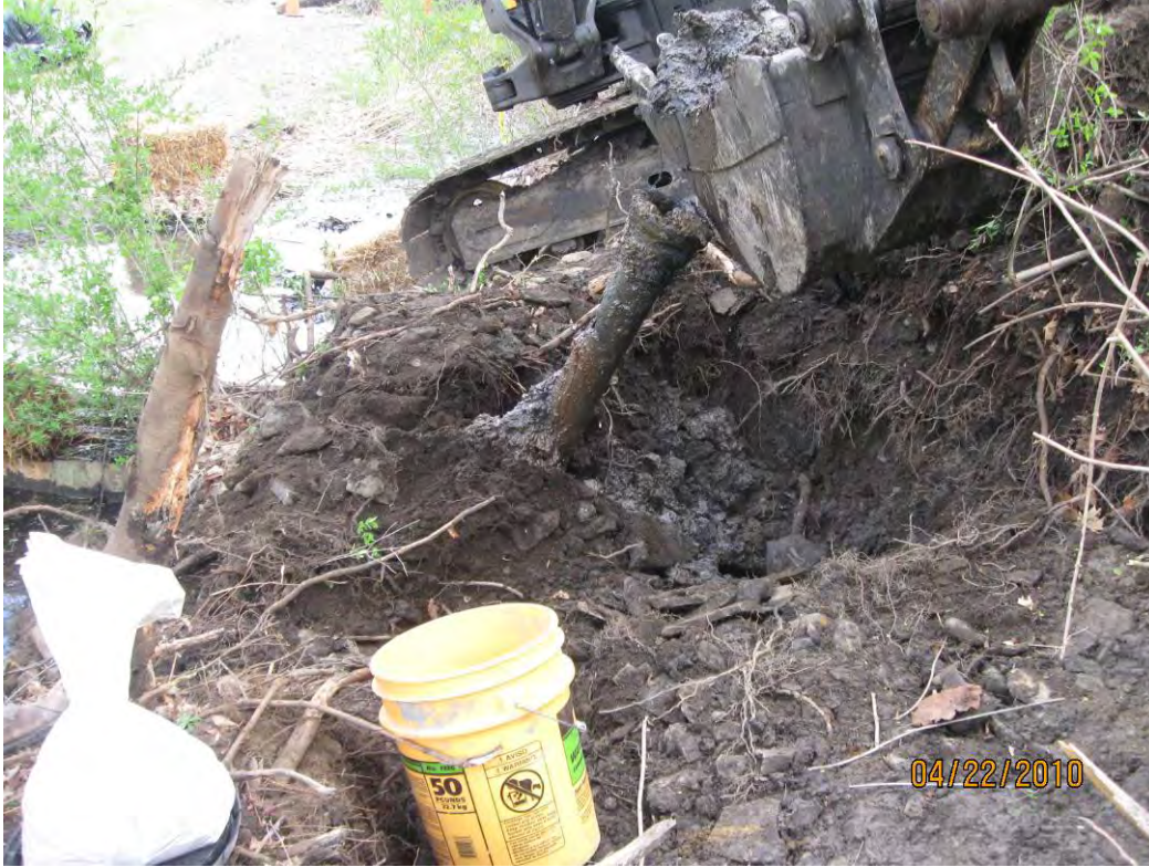
Photograph 29: Pulling the end of the pipe out of the test pit.
