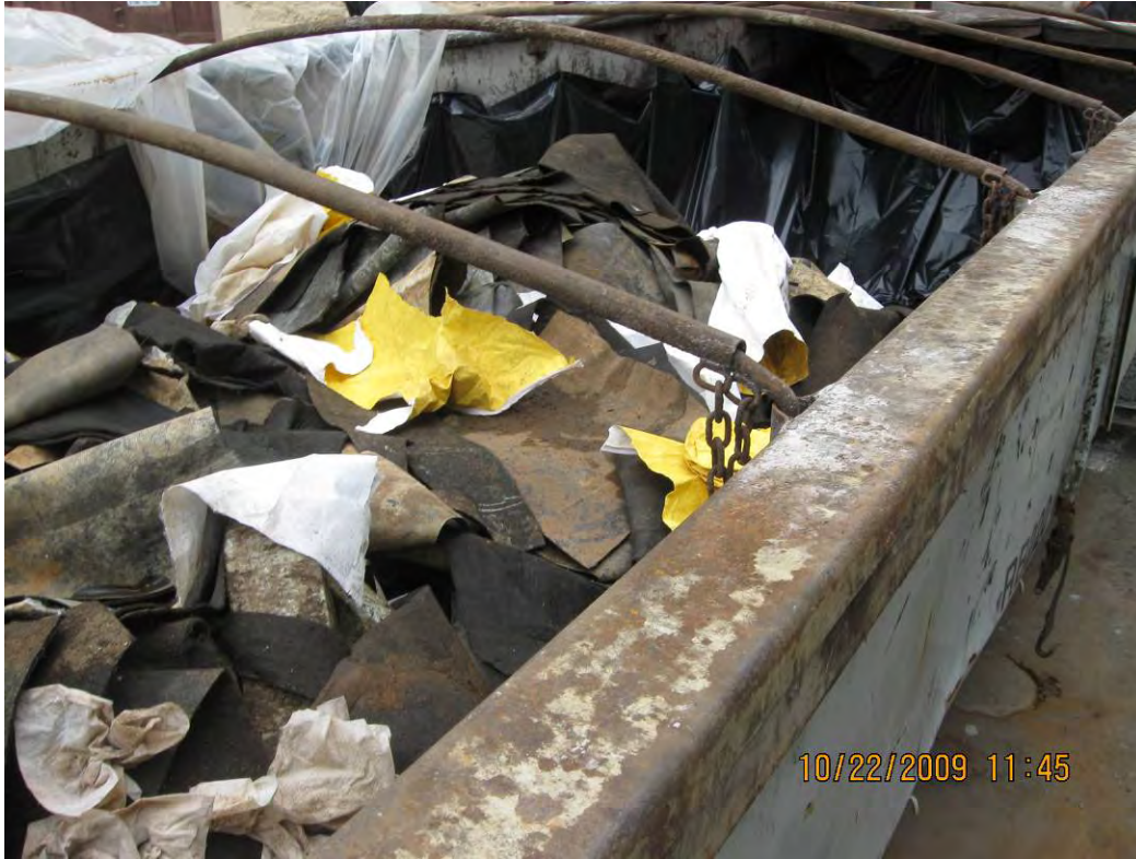
Photograph 11: Hazardous waste roll-off after the removal of liner from the reservoir.
