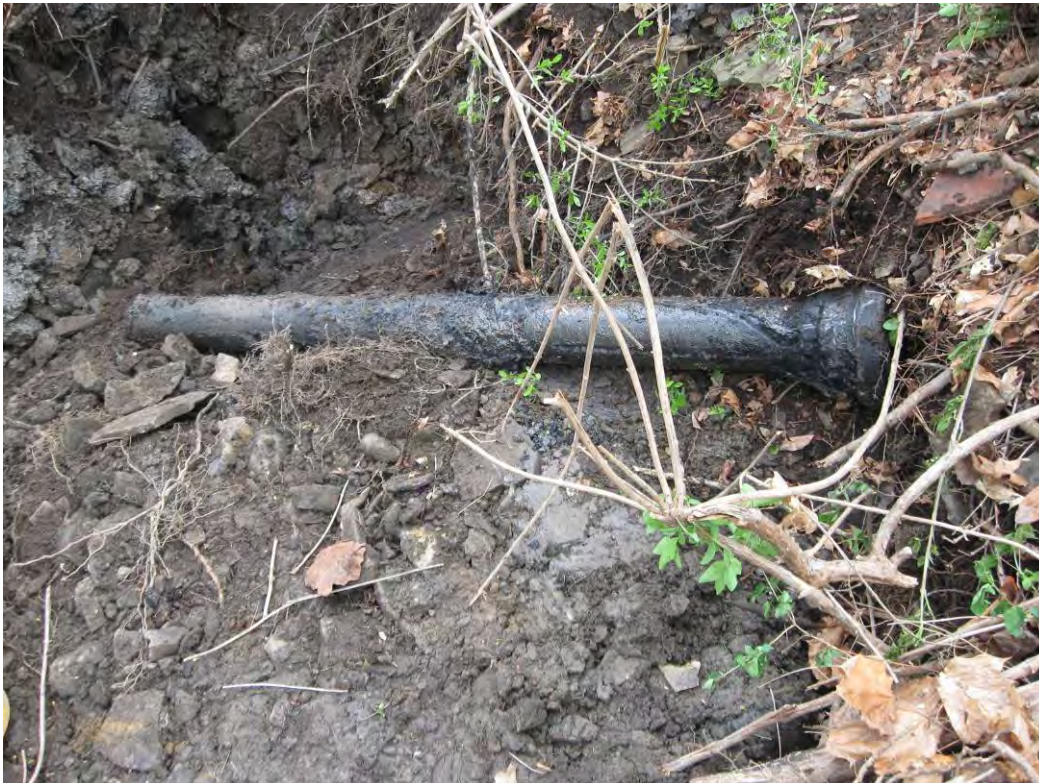
Photograph 30: The end of the pipe (6-foot cast-iron pipe) removed at the edge of the drainage ditch.
