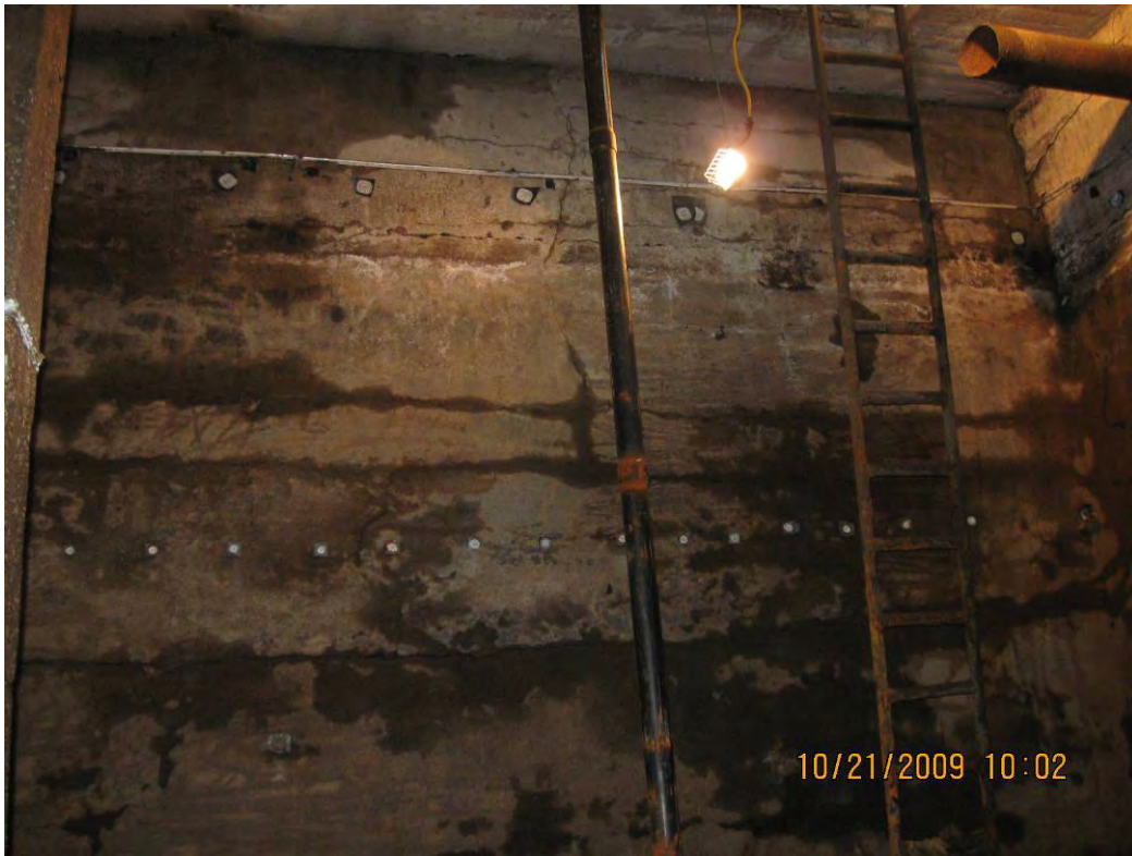
Photograph 6: West wall of the south tank after removal of the liner.
