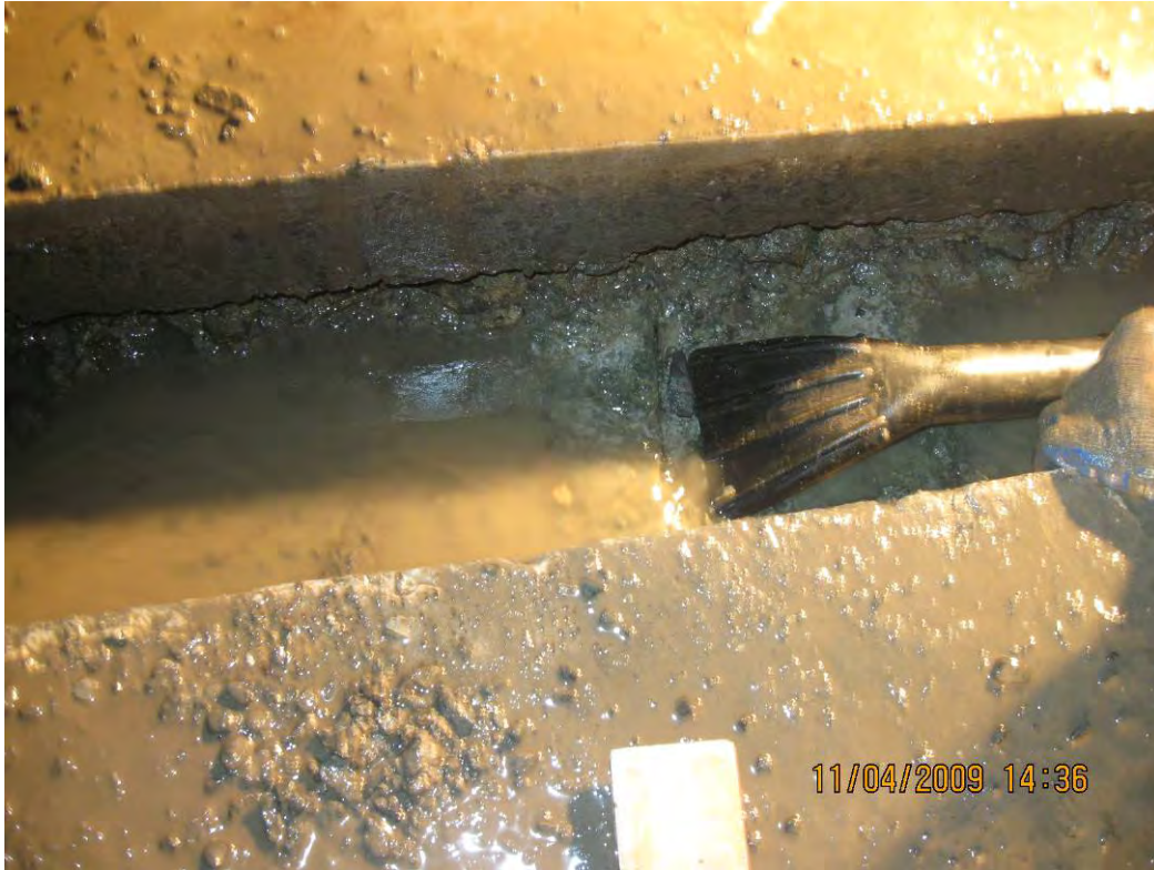
Photograph 15: Vacuuming water from a vertical joint located in T-1.
