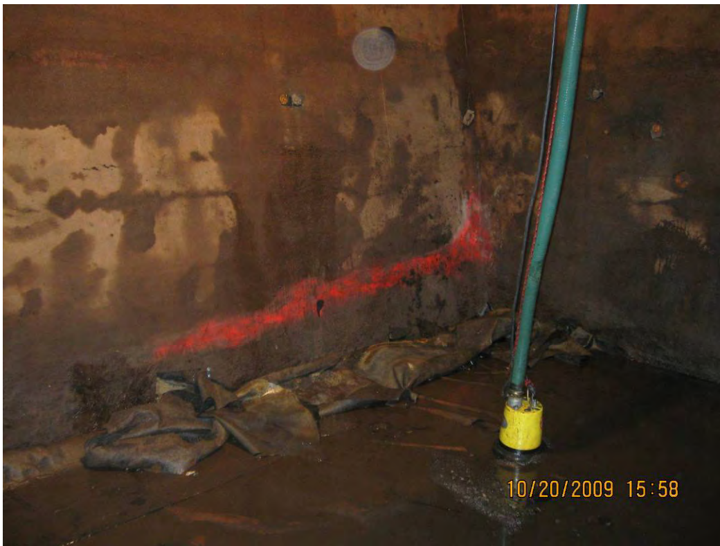
Photograph 4: Sealed crack that was painted.
