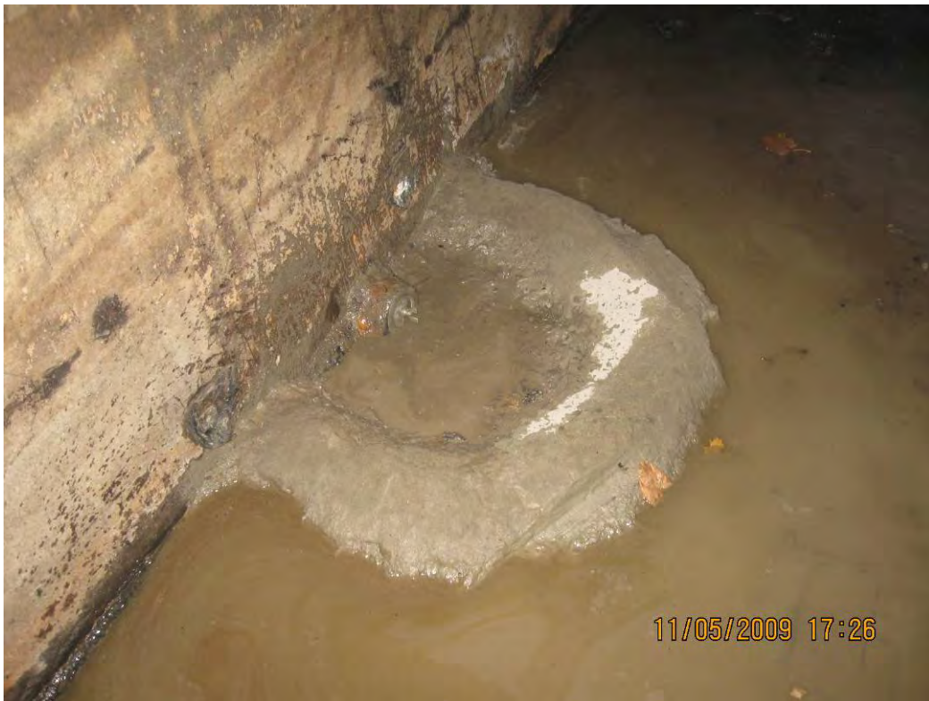
Photograph 21: Dam created around the pipe exiting the north tank to allow for fiber optic viewing.
