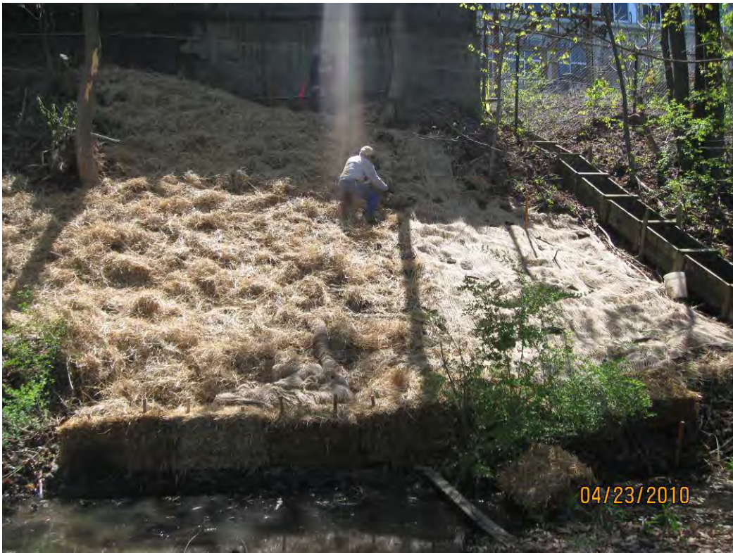
Photograph 32: Installing hay and erosion mat over the excavated areas.
