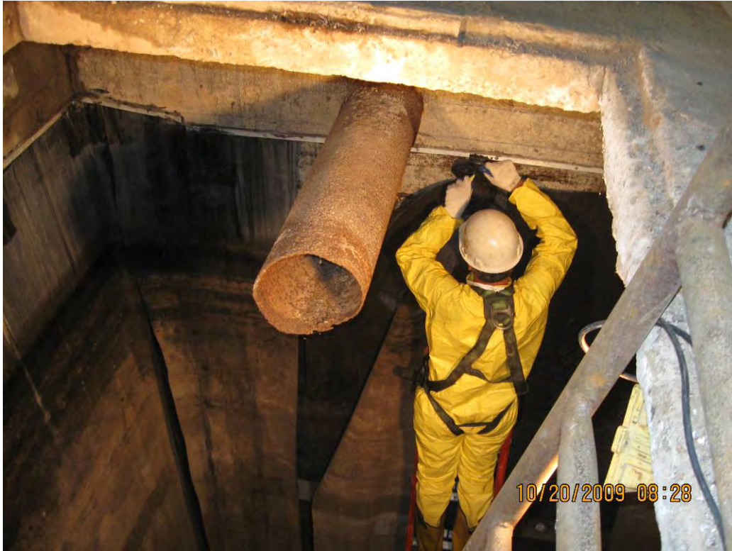
Photograph 1: Cutting the EPDM in strips inside the south tank.
