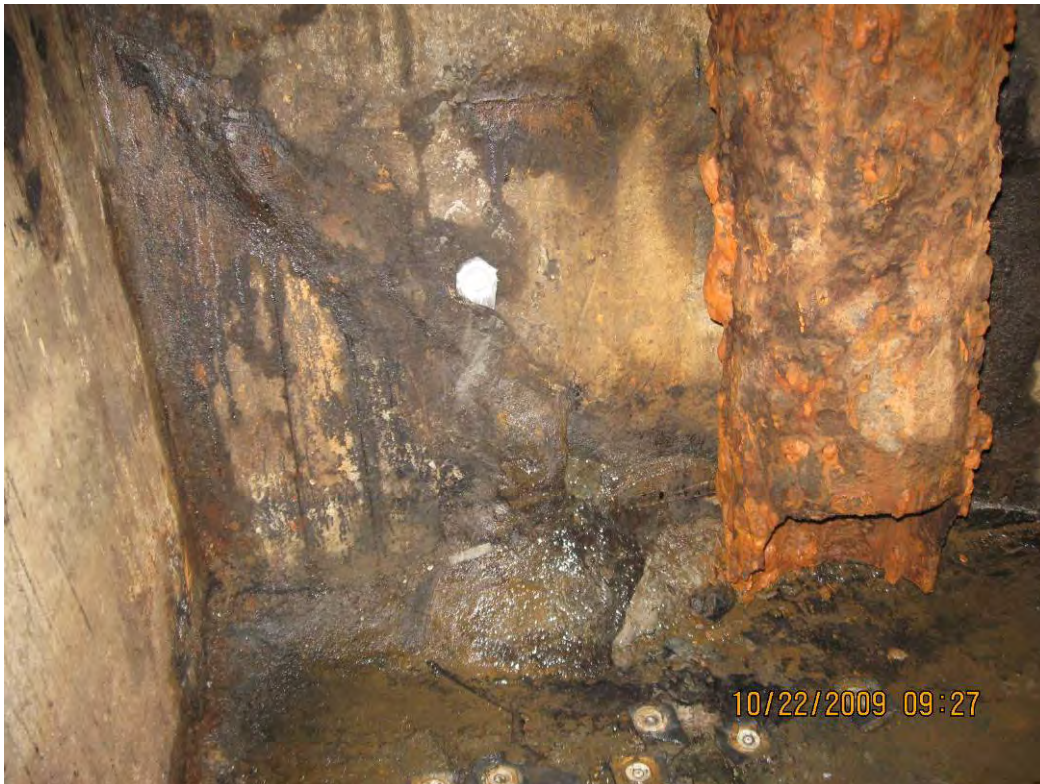
Photograph 10: Hole patched at the northern end of the eastern wall of the north tank.
