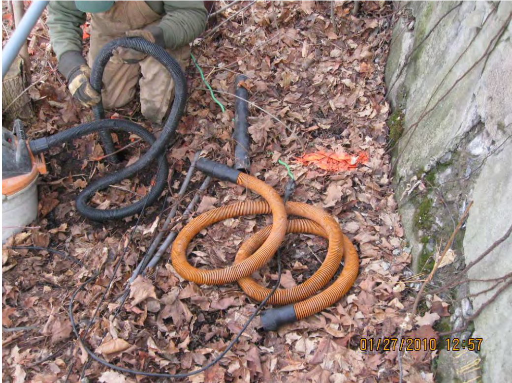
Photograph 22: Vacuuming out the vertical stand pipe located on the west side of the south tank.
