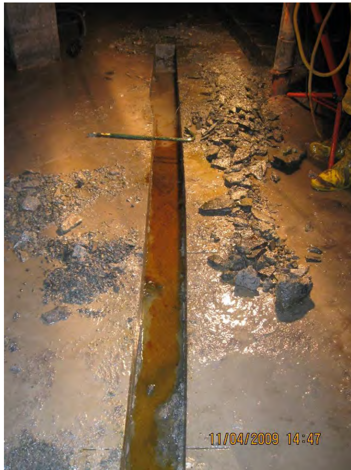
Photograph 17: Petroleum product entering T-2 below floor slab.
