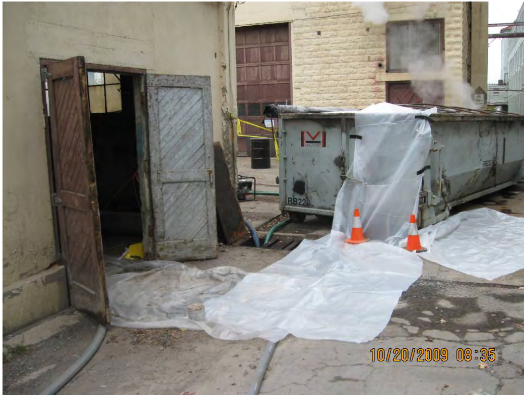
Photograph 2: Decontamination area leading to the hazardous waste roll-off.
