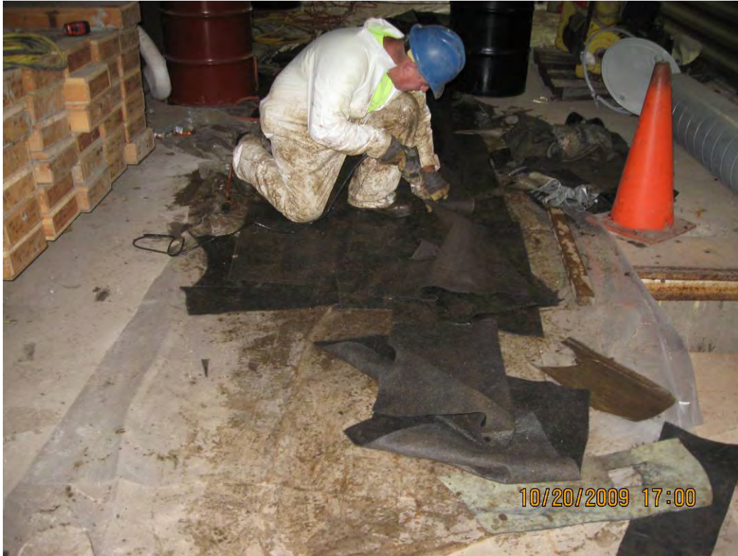
Photograph 5: Cutting the felt backing into squares for disposal into the hazardous waste roll-off.
