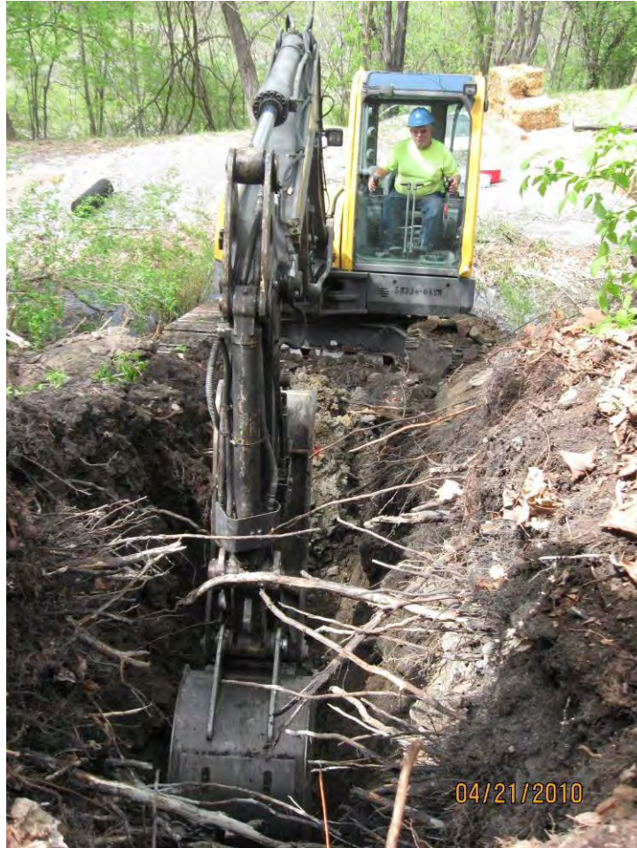
Photograph 24: Excavating up to the vertical stand pipe.
