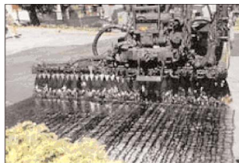
Close-up of unacceptable streaks of asphalt tack coat (refer to Part II C of this brochure).
