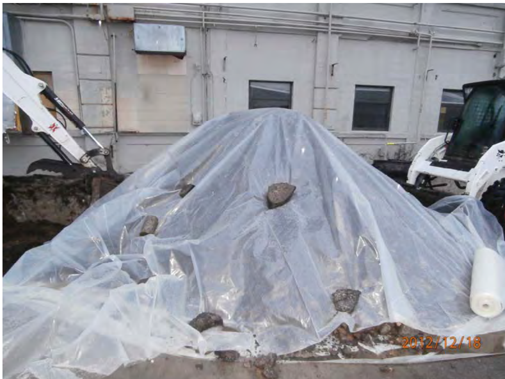
Photo 34: Excavated Material Stockpile
