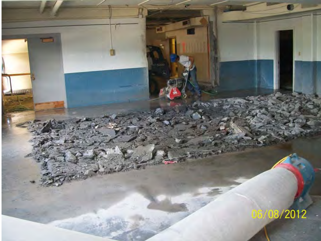
Photo 12: Saw-Cutting between Columns 87 and 89 – Building 4
