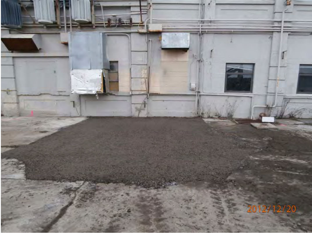
Photo 39: Completed Excavation with Compacted Stone
