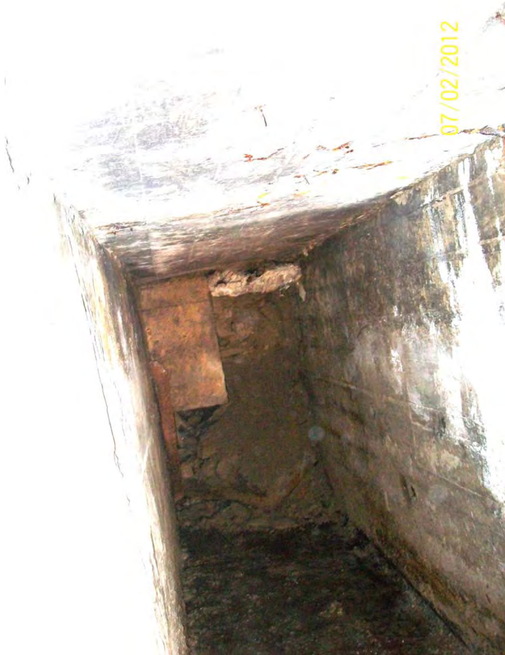
Photo 30: Removal of Impacted Soil Beneath the Transformer – Building 3
