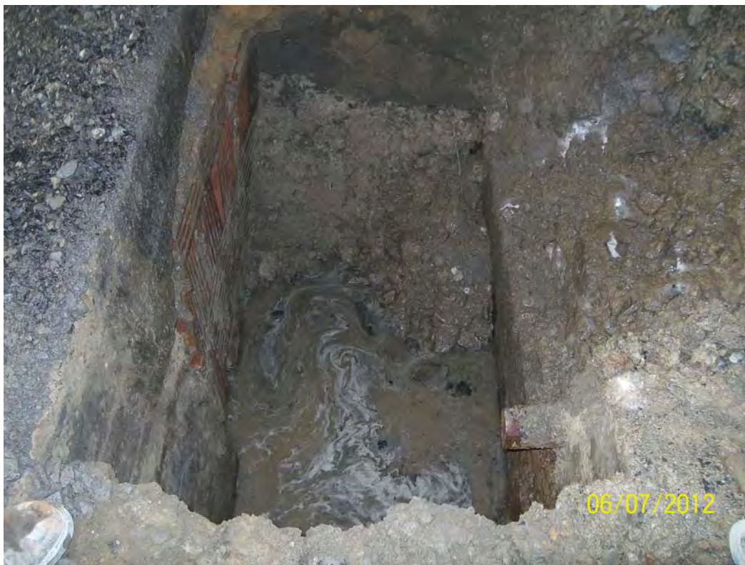
Photo 10: Discovery of the Conveyor Trench at Column 110 – Building 3
