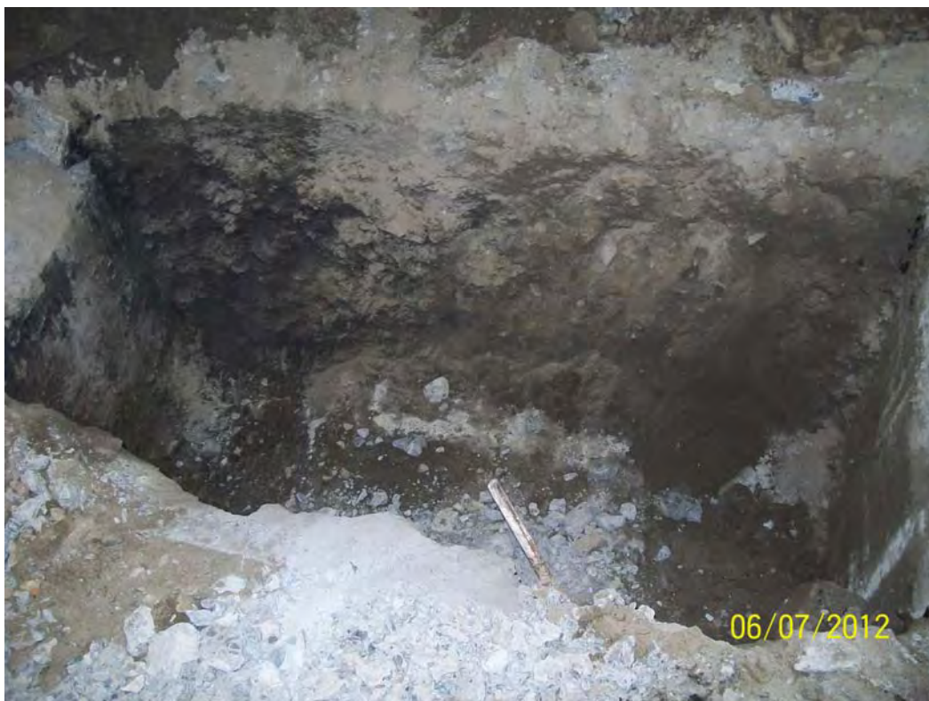
Photo 9: Test Pit Between Two Isolation Pads – Building 3
