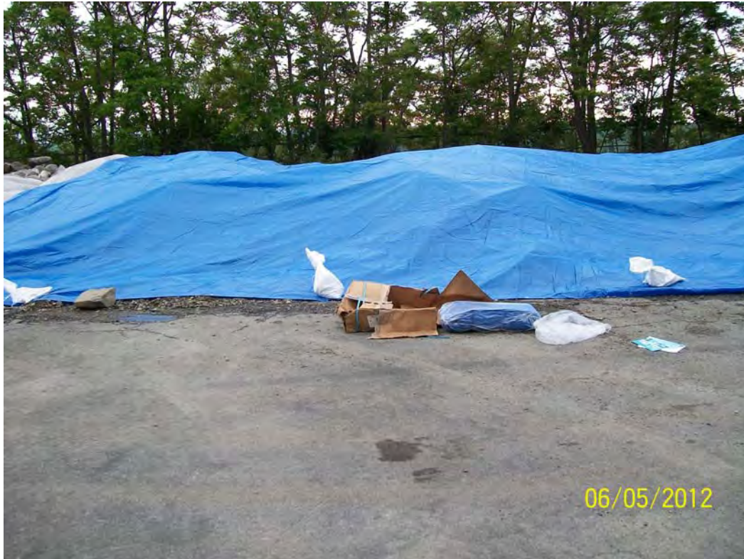
Photo 8: Concrete Stockpile - Bermed and Covered
