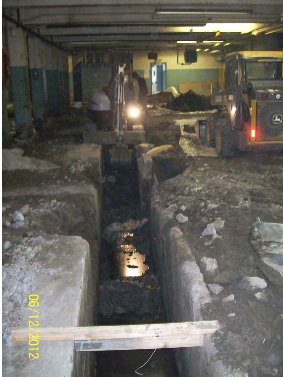
Photo 20: Removal of Impacted Soil from the Conveyor Trench – Building 3
