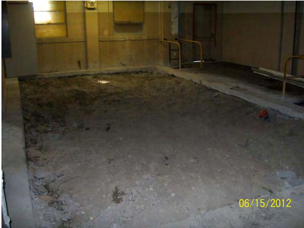
Photo 16: Former Depressed Floor Area – Building 4
