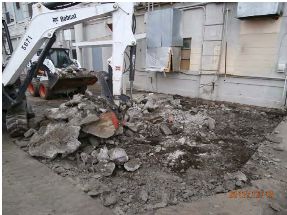
Photo 32: Concrete and Asphalt removal West of the Former Degreaser Area
