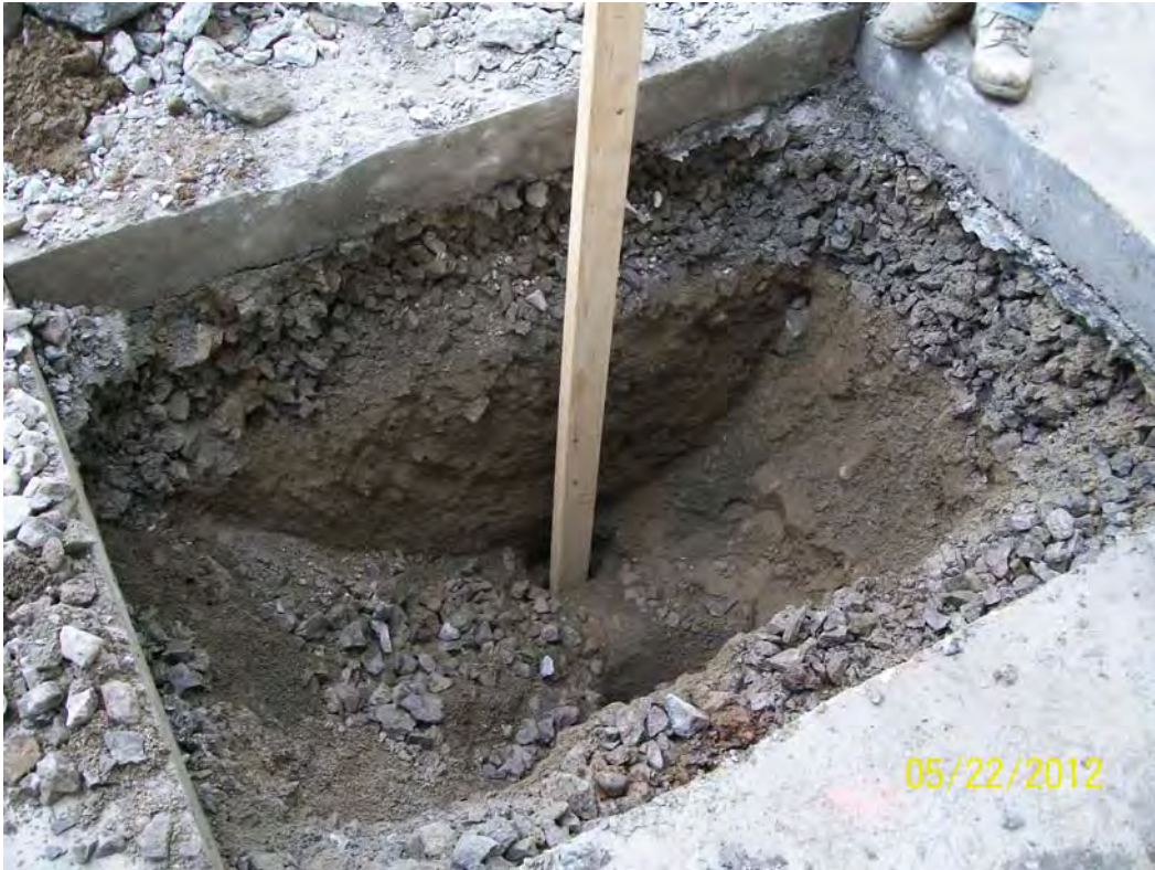
Photo 3: Test Pit 2 – 2x4 Installation Next to Sanitary Sewer Line
