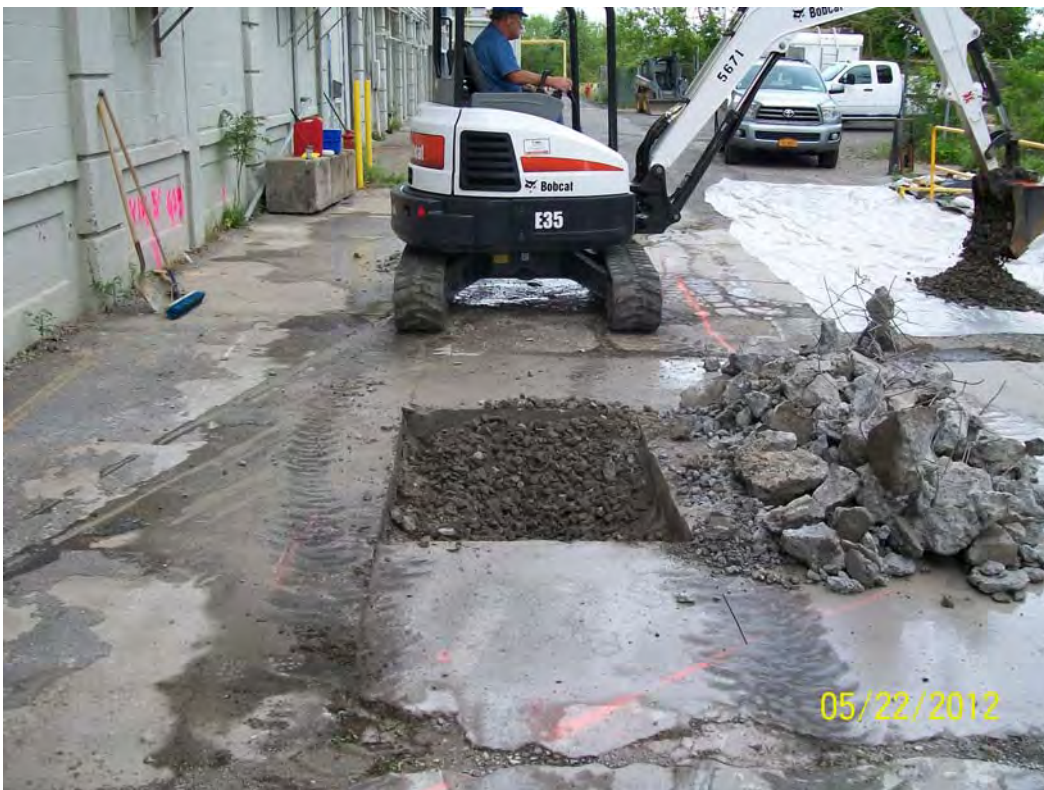
Photo 2: Test Pit 2 – Removal of Subgrade Material
