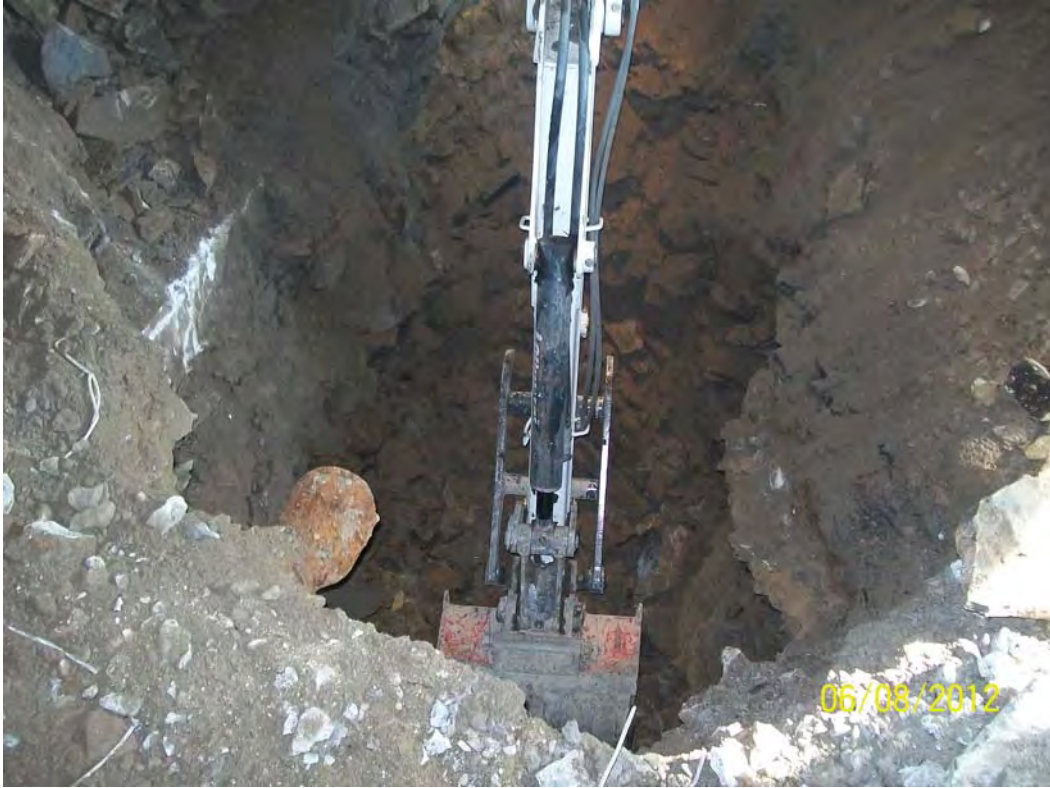
Photo 14: Test Pit West of the Sanitary Sewer Line – Building 4
