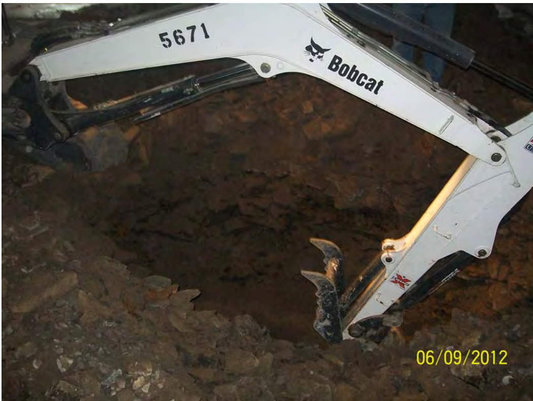
Photo 15: Test Pit East of the Sanitary Sewer Line – Building 4
