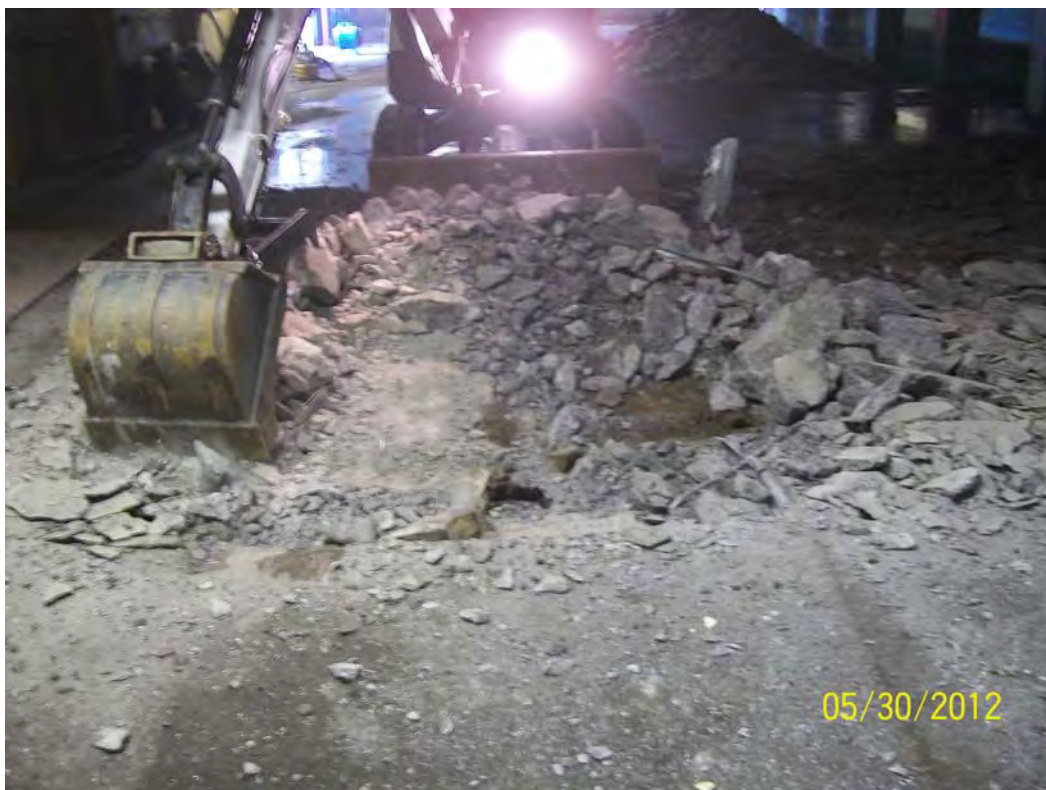
Photo 7: Mini-Excavator Removing Hammered Concrete – Building 3
