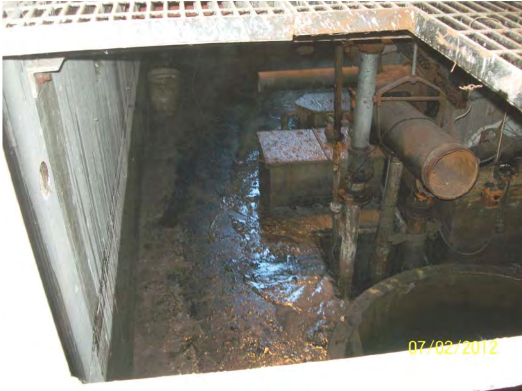
Photo 25: Dewatered Cooling Pit - Building 4
