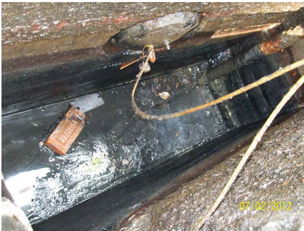
Photo 27: Cleaned Catch Basin Adjacent to the Fire Water Reservoir – West Compartment
