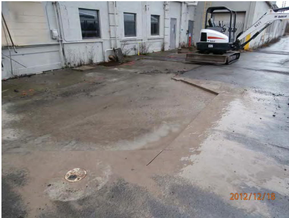
Photo 31: Test Pit Excavation between MW-10B and MW-25B (SB-101112-1) West of the Former Philips Degreaser
