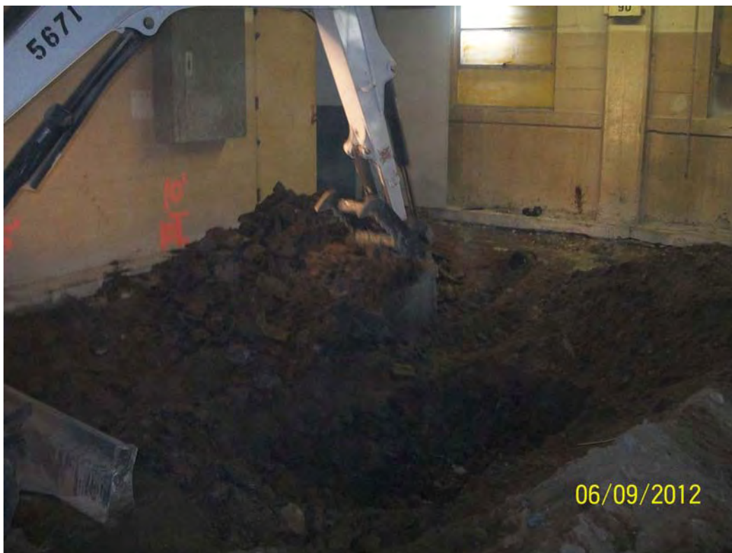
Photo 17: Test Pit in the Former Depressed Floor Area – Building 4
