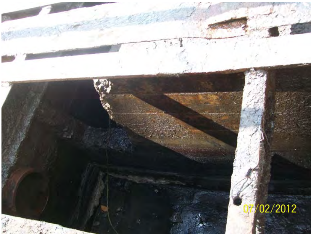
Photo 26: Cleaned Catch Basin Adjacent to the Fire Water Reservoir – East Compartment
