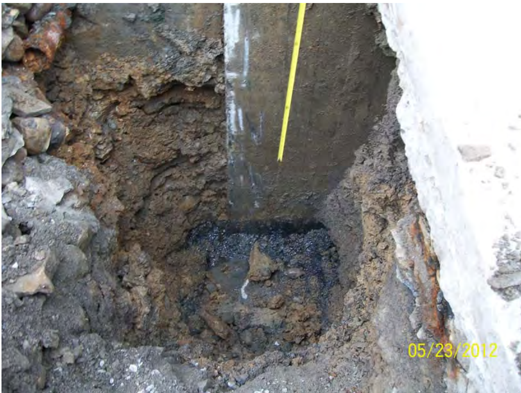
Photo 4: Test Pit at Column 107
