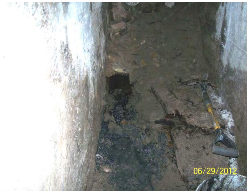
Photo 28: Removal of Impacted Soil Beneath the Transformer – Building 3
