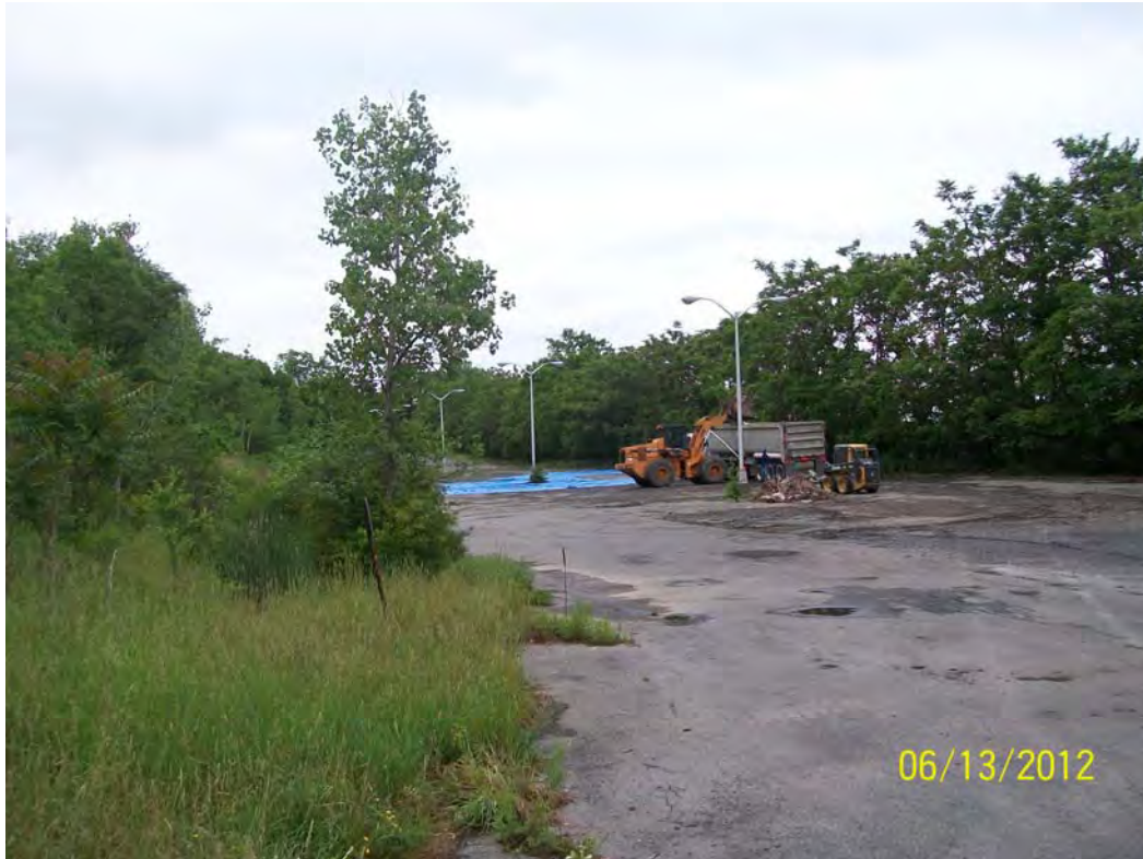
Photo 21: Loading the Final Truck for Concrete Disposal
