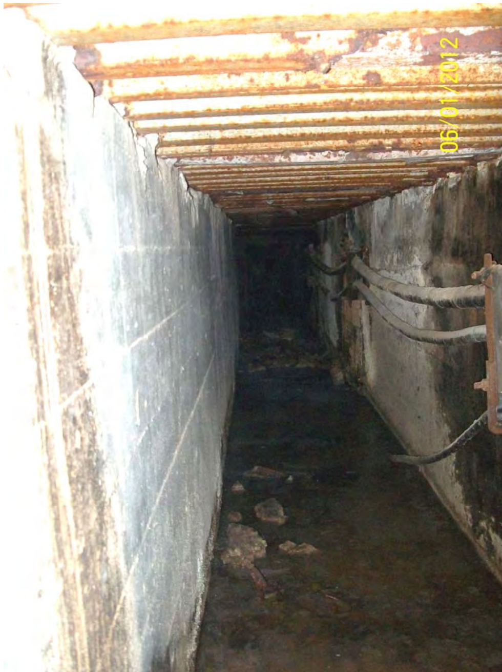
Photo 5: Utility Trench – Building 3
