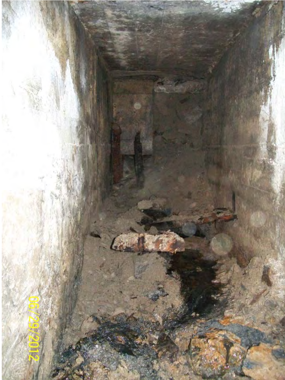
Photo 29: Removal of Impacted Soil Beneath the Transformer – Building 3
