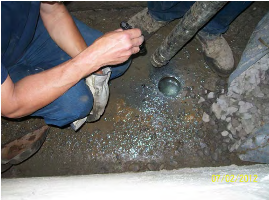
Photo 23: Core-1 Location – Building 3
