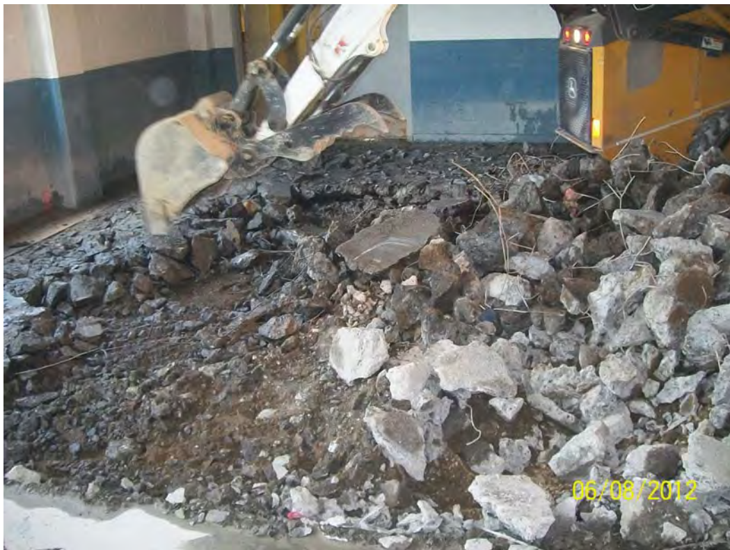
Photo 13: Removal of Concrete between Columns 87 and 89 – Building 4
