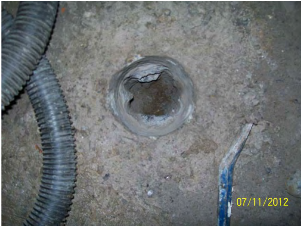
Photo 24: Core-2 Location – Building 4
