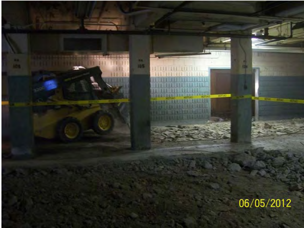
Photo 6: Skid Steer with Hydraulic Hammer – Building 3
