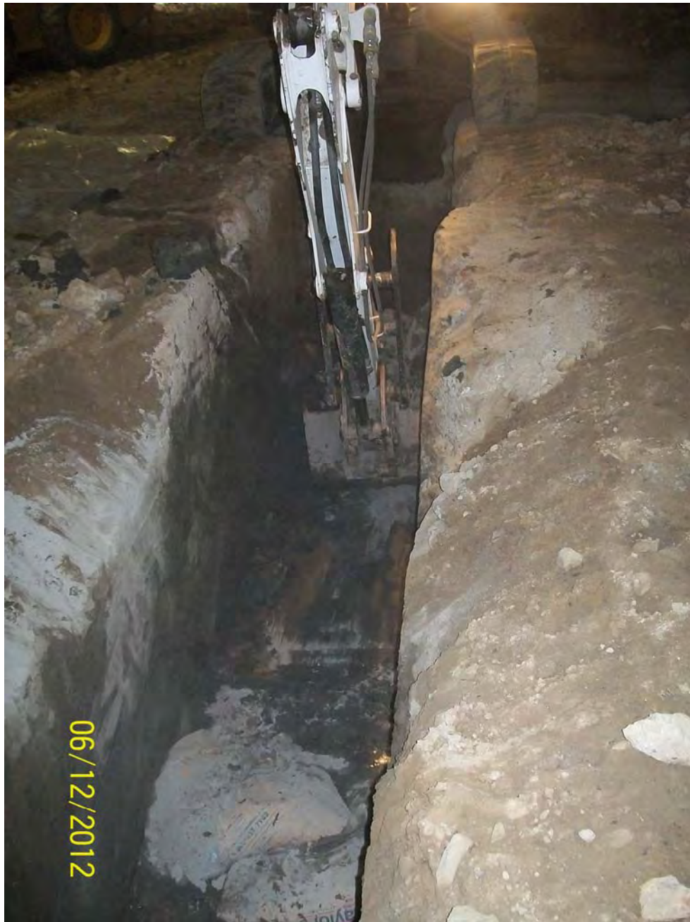
Photo 19: Removal of Impacted Soil from the Conveyor Trench – Building 3
