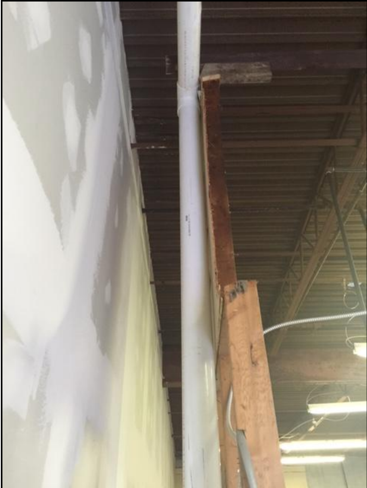
Photo #8: Photo of Exhaust Riser Pipe
