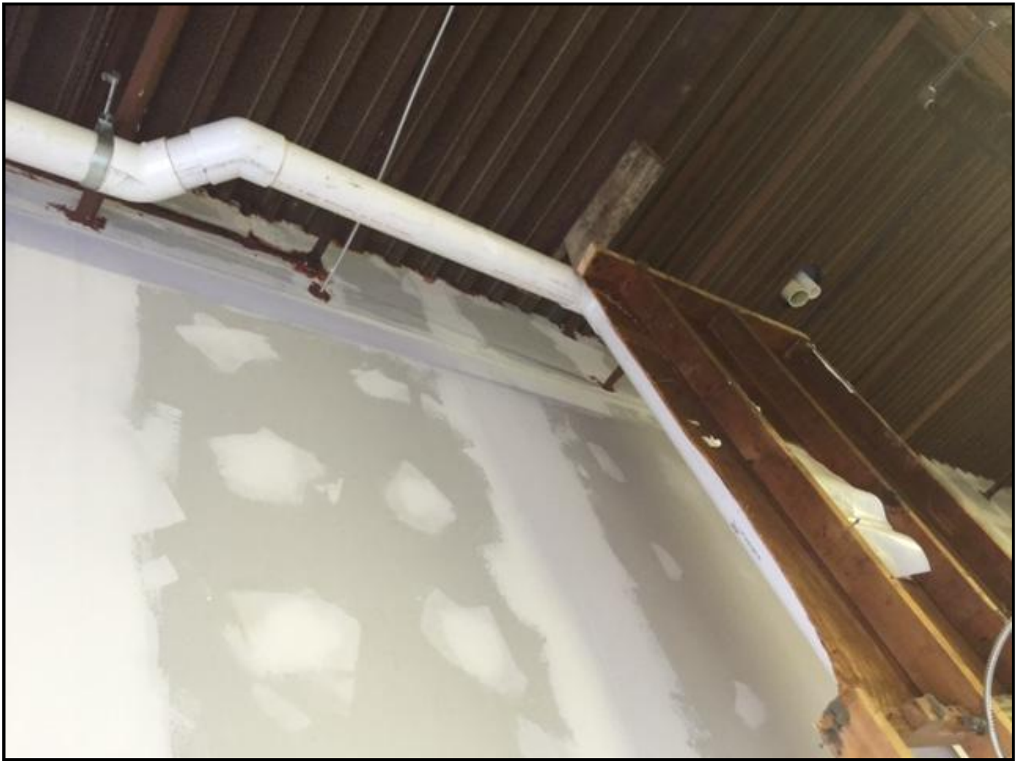
Photo #7: Photo of Exhaust Pipe and Riser
