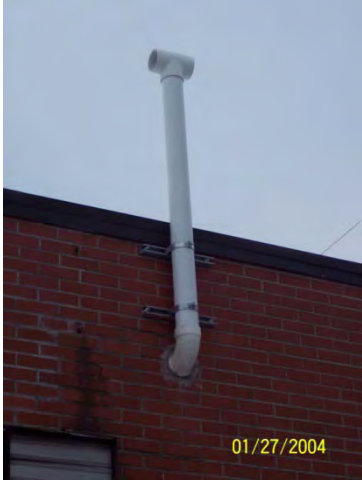
View of exhaust stack above building
