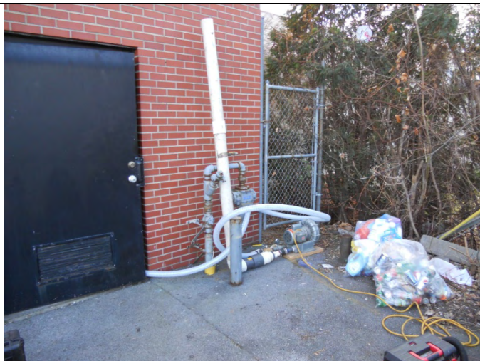
View of blower and effluent discharge setup from the west
