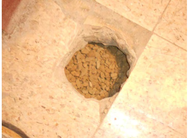
View of cored extraction point
