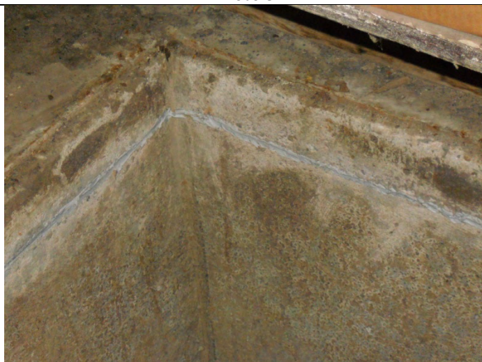
Seal applied to the slab and lint wall interface
