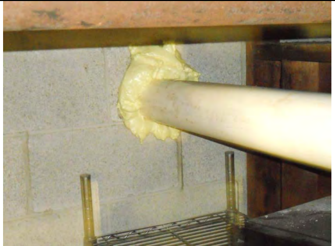
View of piping and seal through building wall
