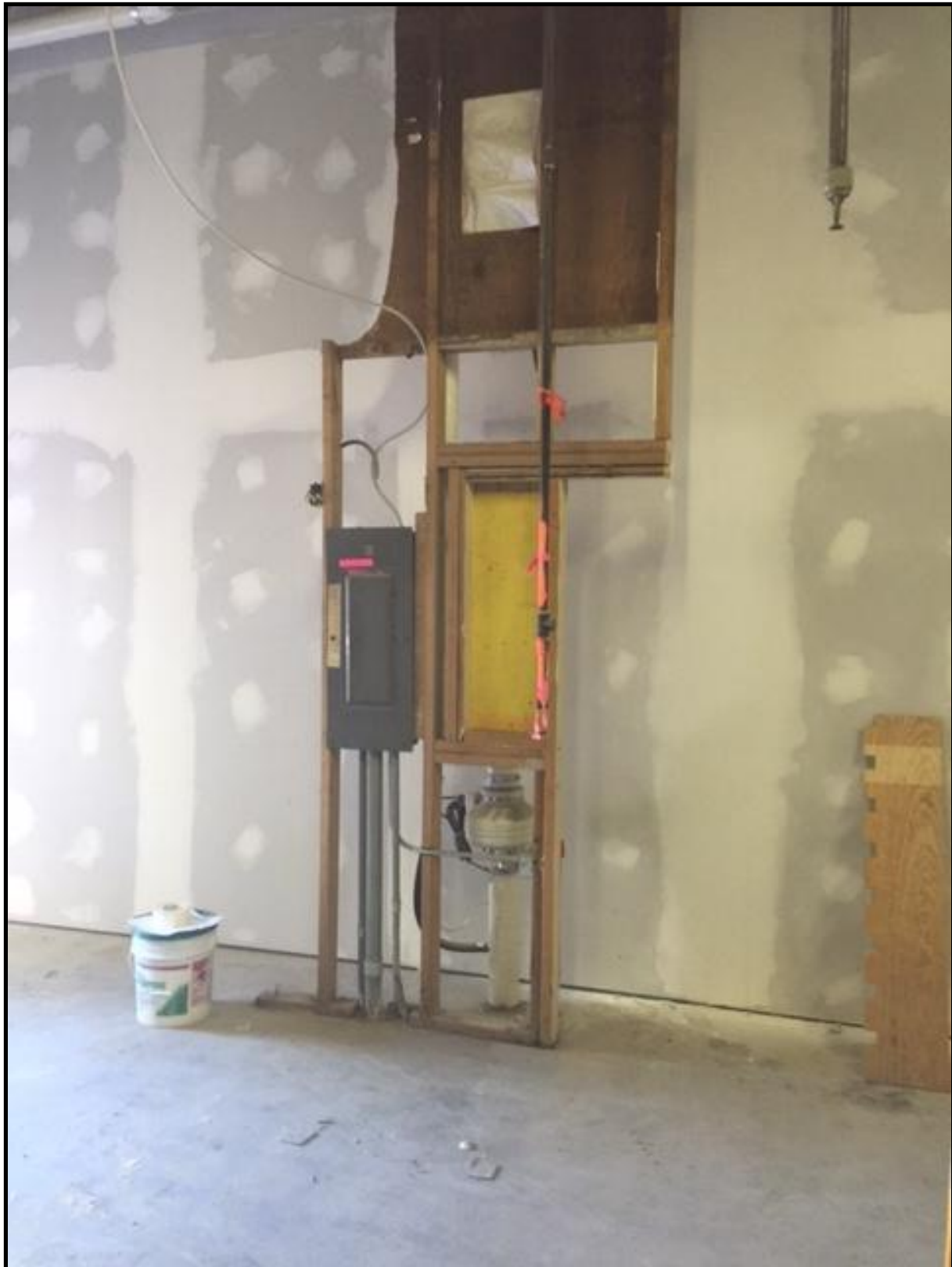
Photo #4: Photo of Electrical Panel and SSDS
