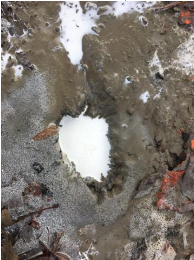
EOS substrate mixture forced upward at INJ-16
