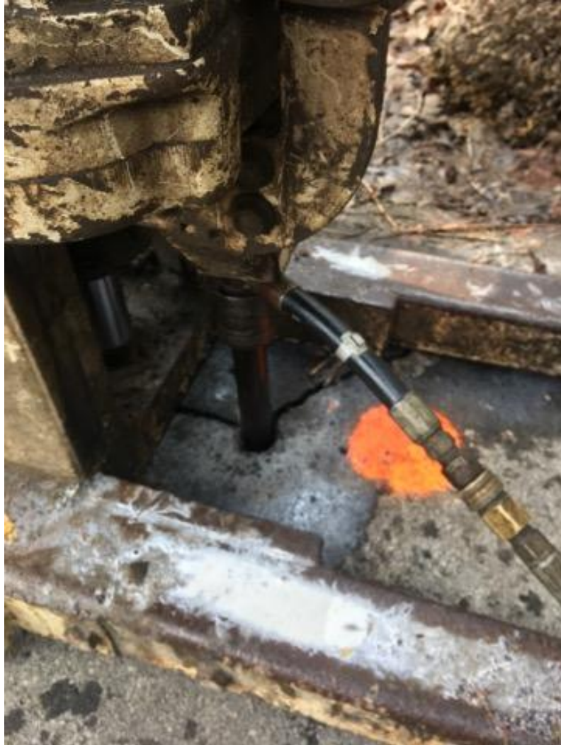
Ongoing EOS substrate Injection at INJ-15
