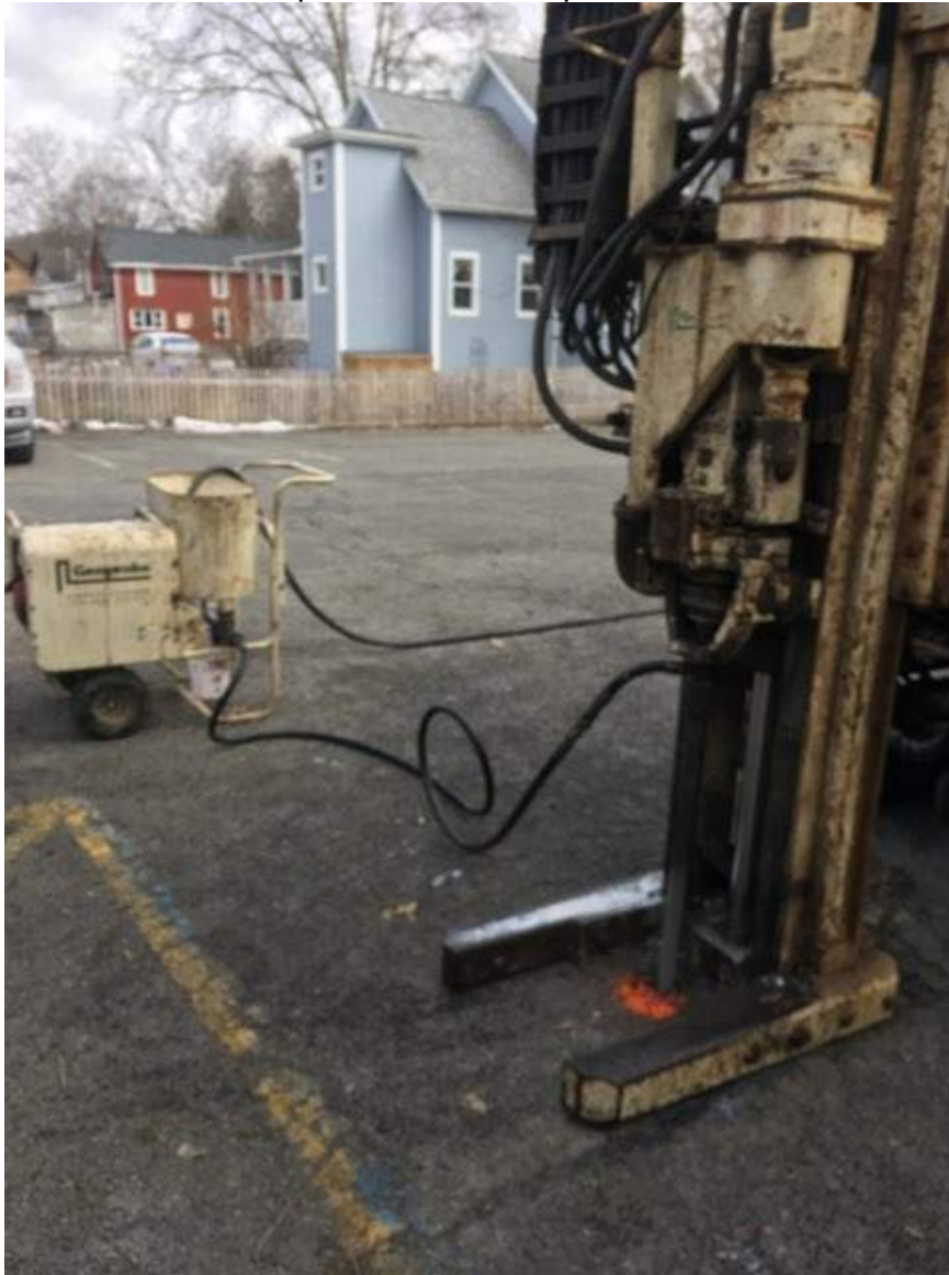
Geoprobe 6620 set-up at INJ-25
