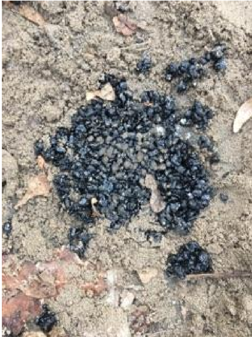
Borehole restored with sand and QPR
