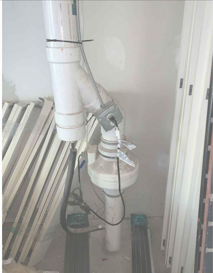
3 | SSDS FAN AND ENTRY INTO SLAB
