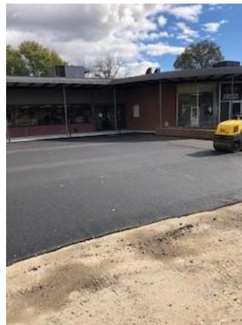
PHOTO NO. 8 VIEWING EAST AT BUILDING SHOWING BINDER COURSE PLACEMENT OF NEW PARKING LOT, 11/05/2021
