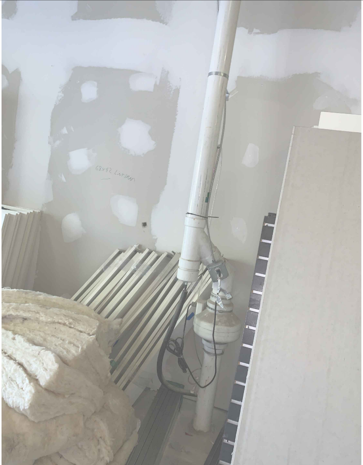
4 | SSDS FAN AND ENTRY INTO SLAB
