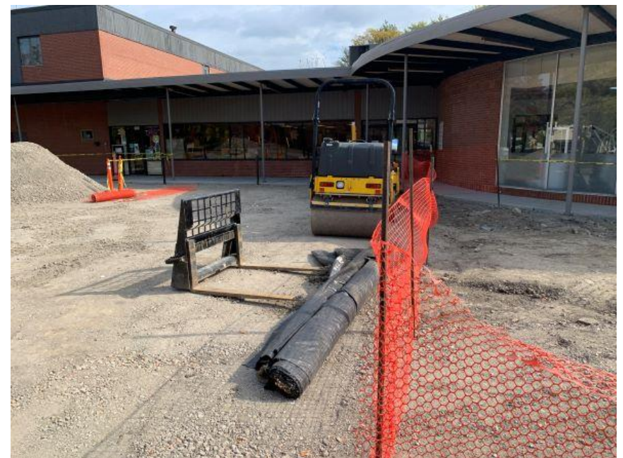
PHOTO NO. 4 VIEWING EAST/NORTHEAST AT BUILDING, SUB-BASE EXPOSED, 10/15/2021
