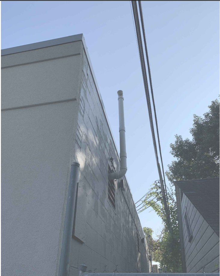
8 | SSDS EXHAUST TO EXTERIOR
