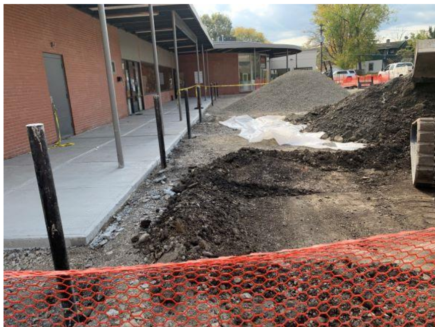
PHOTO NO. 7 VIEWING SOUTH AT BUILDING CANOPY SHOWING NEW CONCRETE WALKWAY AND PROPOSED LIMITS OF PARKING LOT AT STEEL POSTS (BOLLARDS) 10/15/2021
