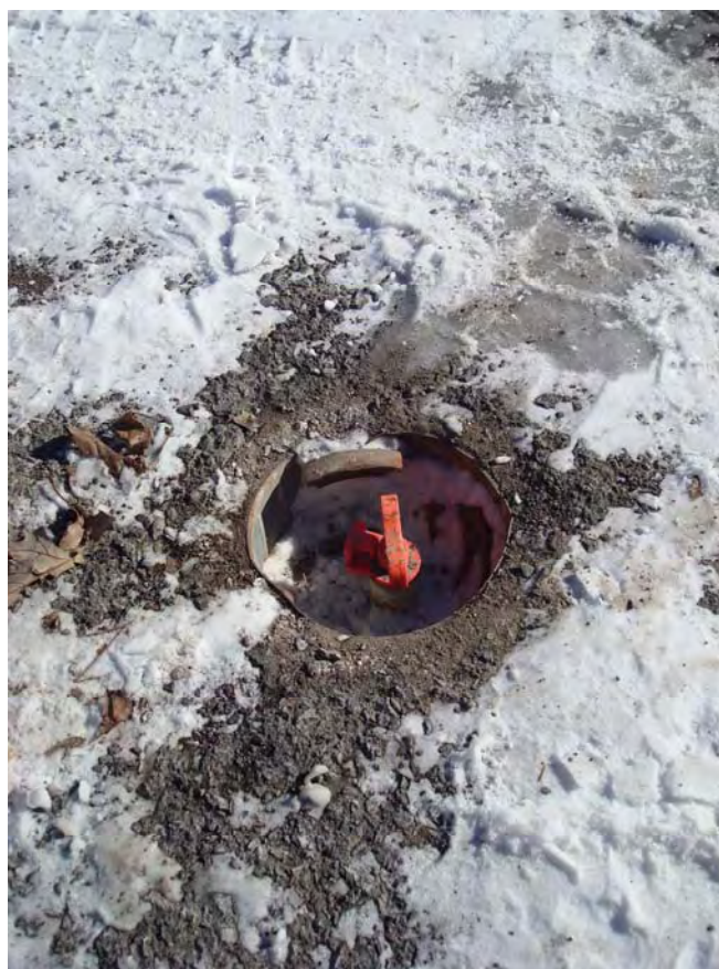
Well head missing from TPM-03.
