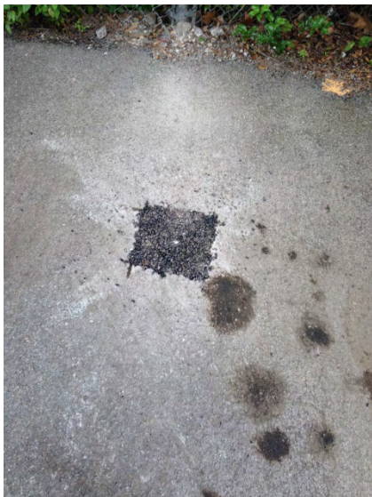
Decommissioned well MW-11 covered with asphalt patch
