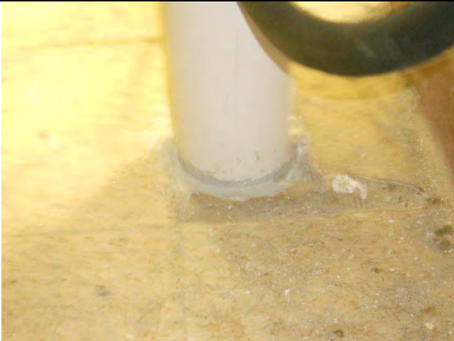
View of sealed extraction point
