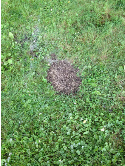
Decommissioned well MW-10 covered with top soil and seeded
