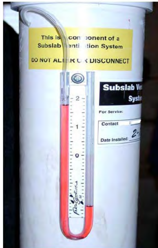
FIGURE 3: SAMPLE MANOMETER SHOWING PROPERLY OPERATING SSD SYSTEM
