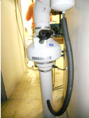
View of fan unit with condensate redirect
