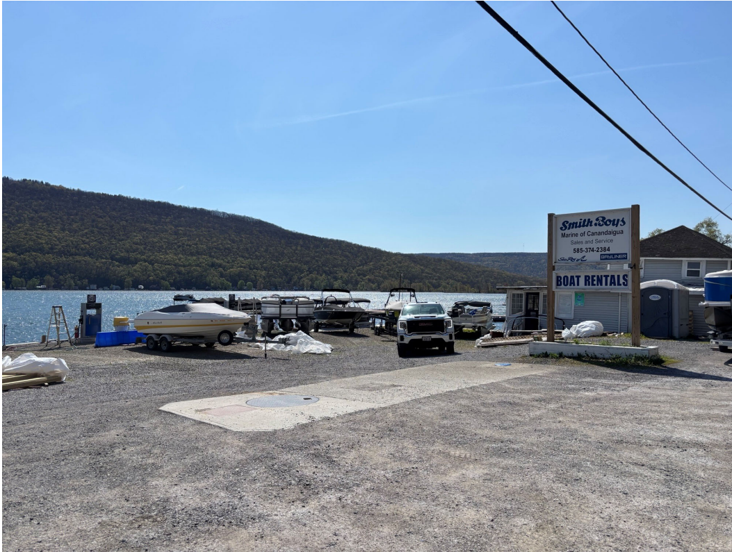
UST Tank pad – Tank 001 (4,000 gallon e-free gasoline)
