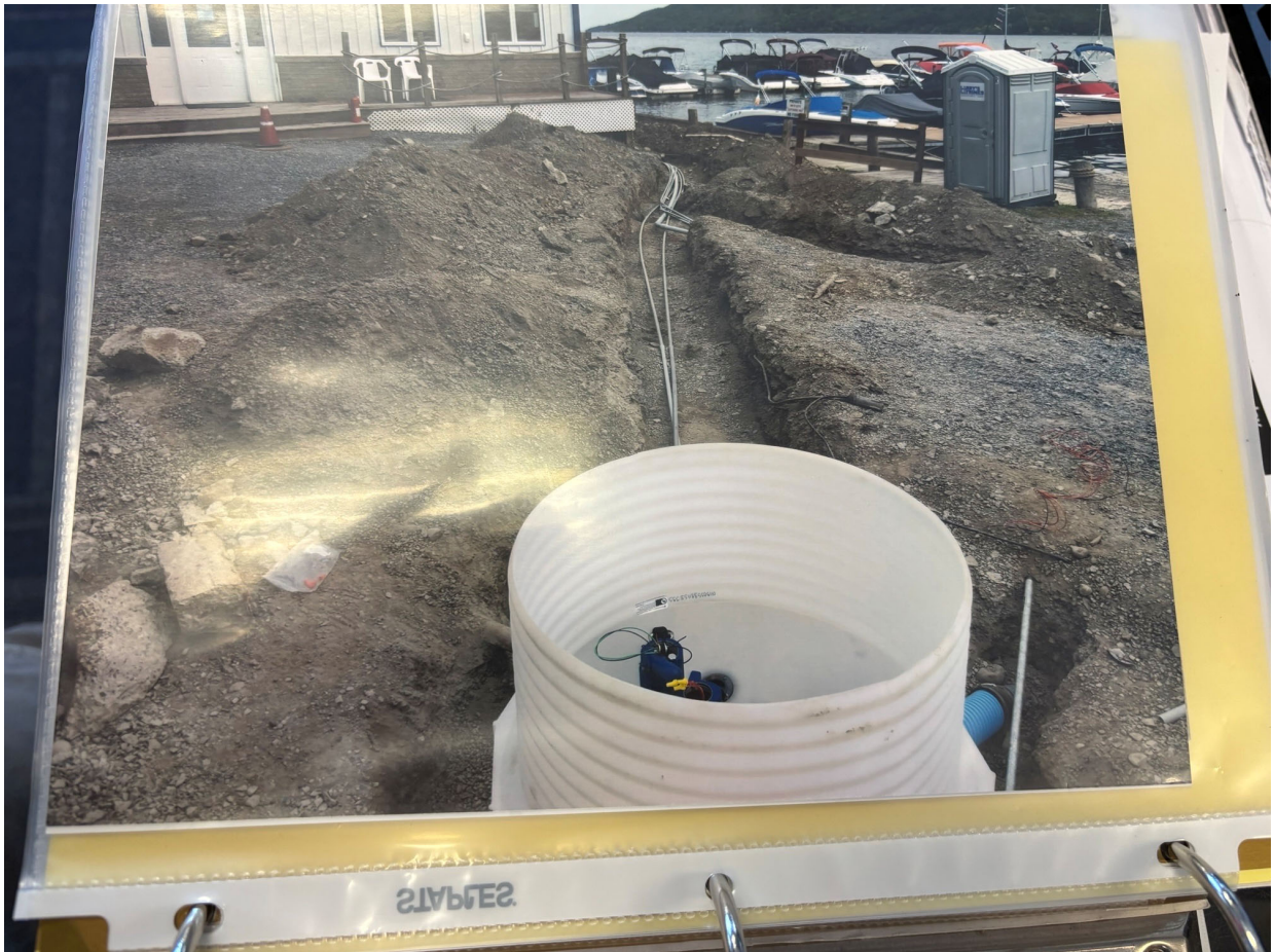
Photo of new tank top sump Sept 2023
