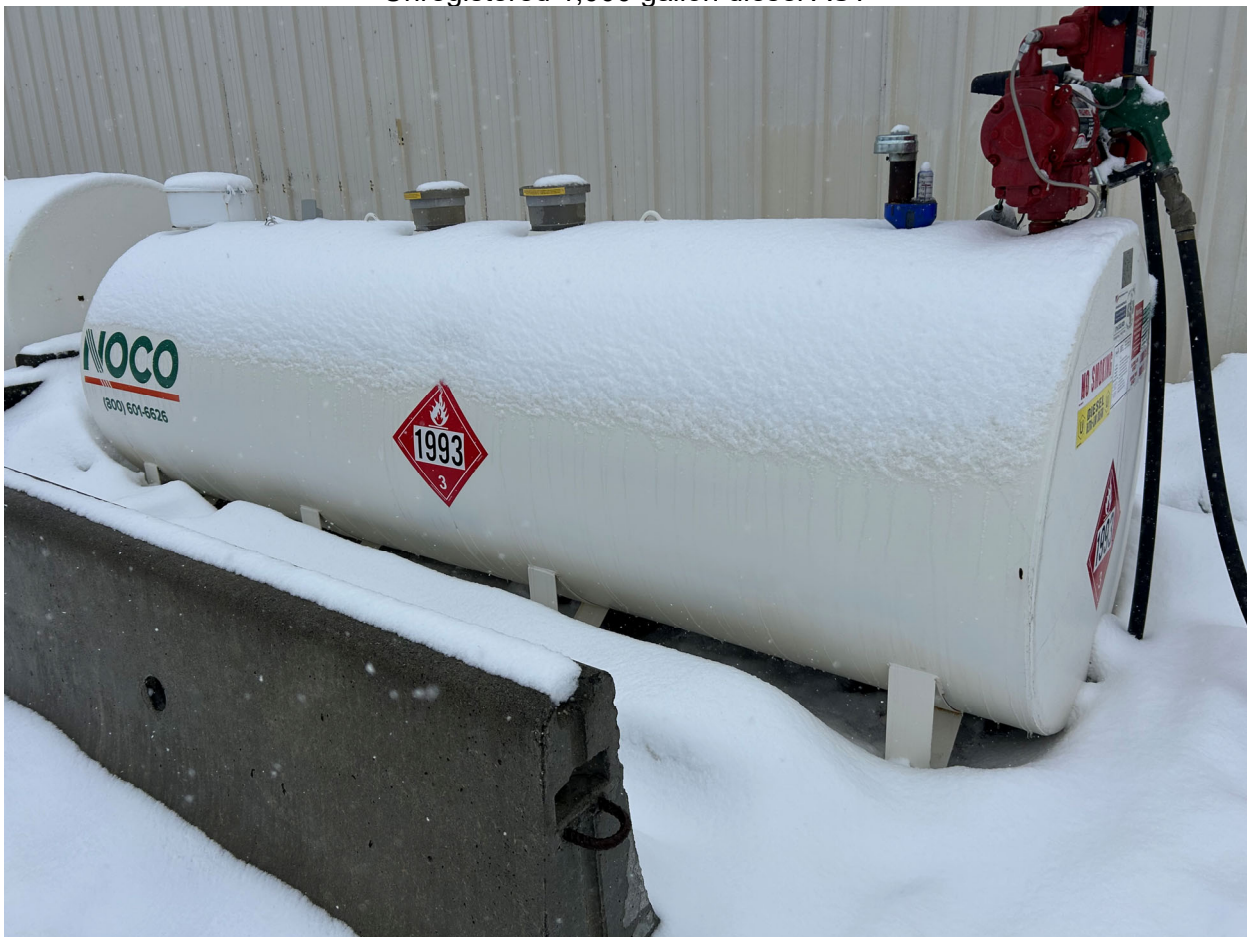
Unregistered 1,000 gallon diesel AST
