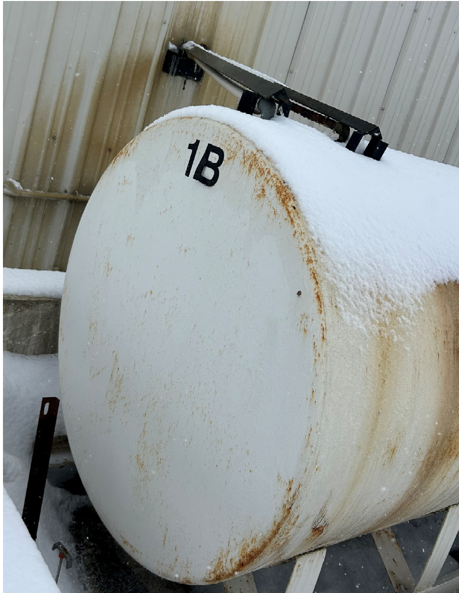
Tank 1B - 1,000 gallon used oil tank manifolded to tank 1A. Tank needs repainting and labeling (design and working capacities)
