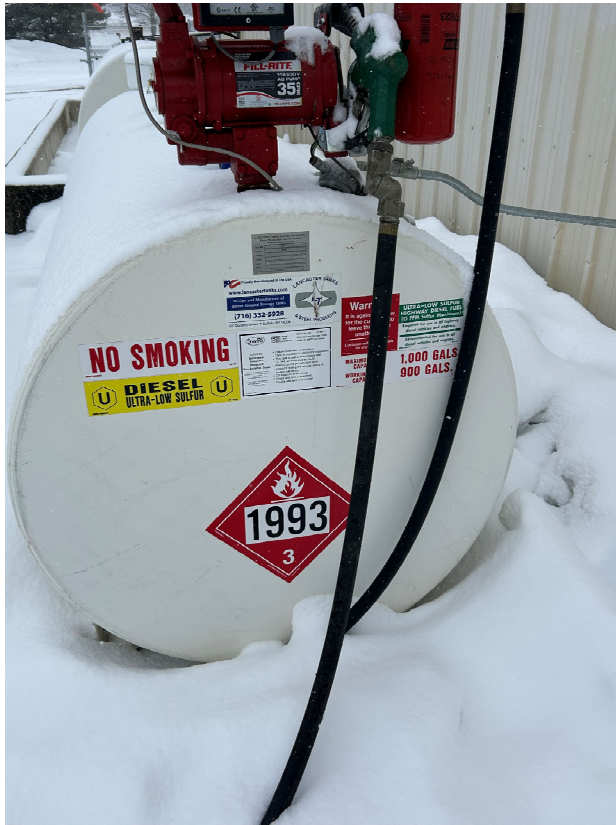
Unregistered 1,000 gallon diesel AST
