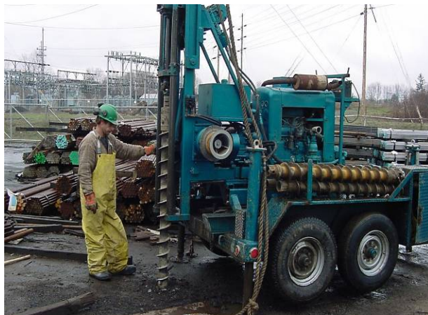
Figure 4.1 - Operating Drilling Rig: Drilling soil boring SB-242 on Trayer's property, looking northwest toward substation.
