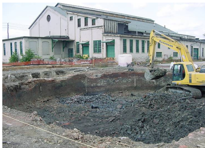
Figure 2.1 - Photo of Gas Holder No. 1 IRM: October 21, 2003. Excavating contents of Gas Holder No. 1, looking northwest.
