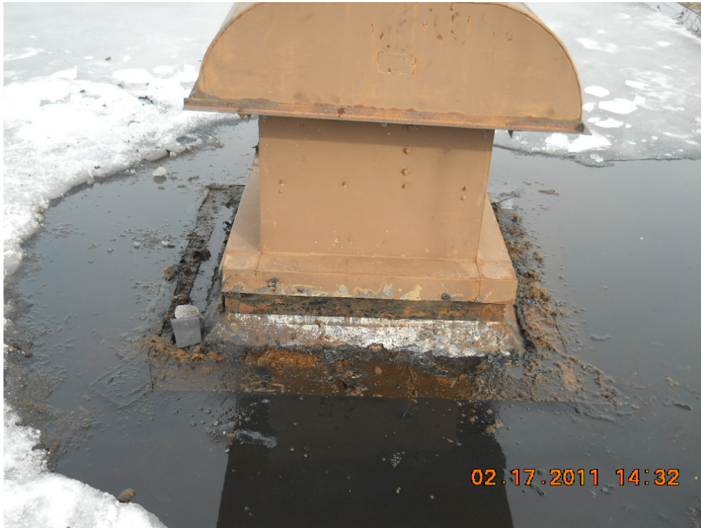
Photo #5: February 17, 2011 – ACM removal from roof flashing (front of building).
