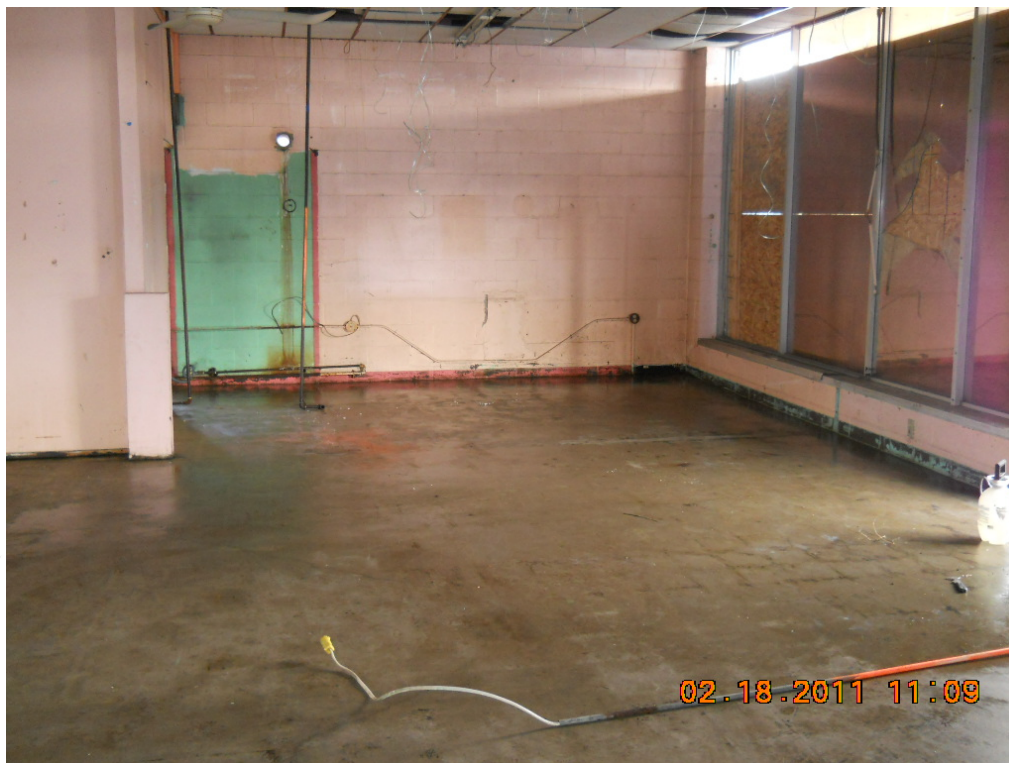
Photo #7: February 18, 2011 – ACM removal of tile/cement board from front/office area.
