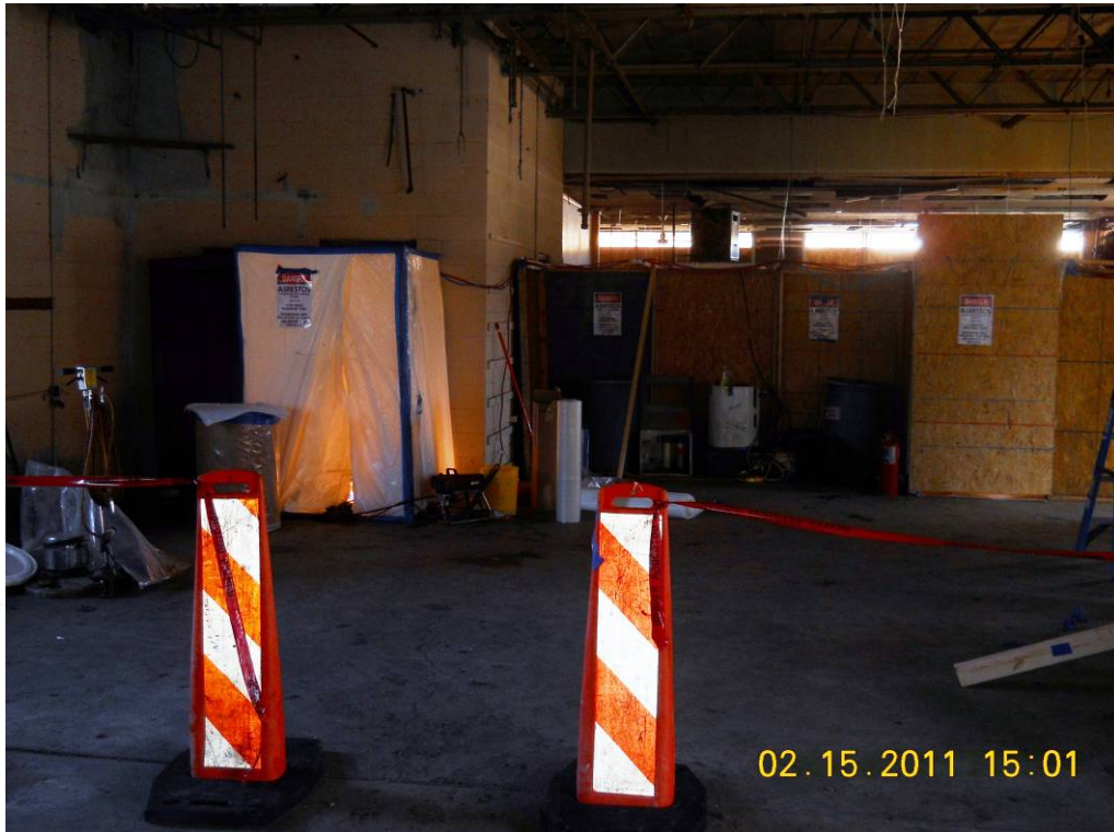
Photo #1: February 15, 2011 – Asbestos abatement preparation office area.
