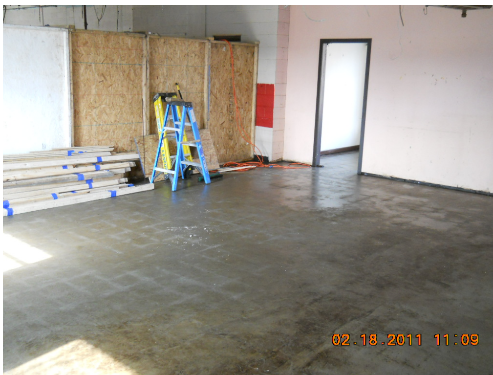
Photo #8: February 18, 2011 – ACM removal of tile from front/office area.
