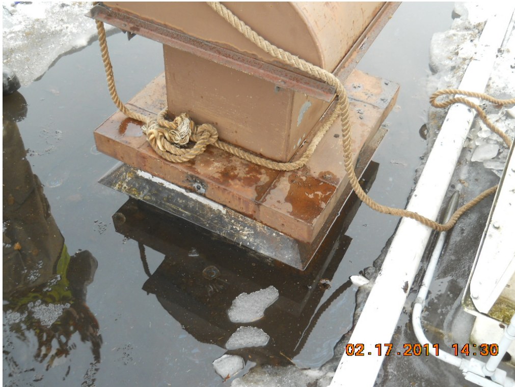
Photo #3: February 17, 2011 – ACM removal from roof flashing (back of building).
