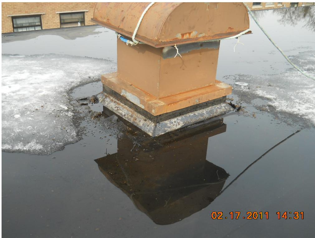
Photo #4: February 17, 2011 – ACM removal from roof flashing (center of building).
