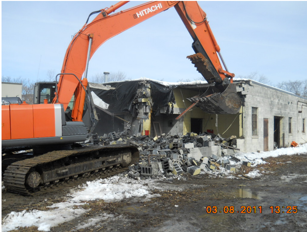
Photo #15: March 8, 2011 – Removal of steel from demolition debris.
