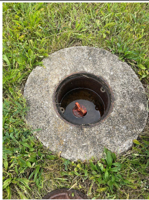
Photo 8: MW-004 had water inside the outer casing. The J-plug was secure and water did not infiltrate the well.
