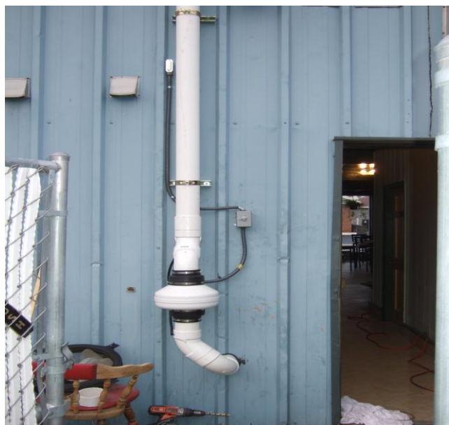
Photo No. 2: Blower and on-off switch.
