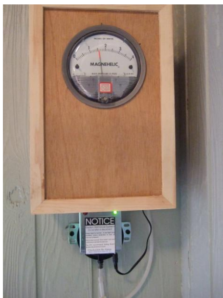
Photo No. 3: Magnehelic gauge and vacuum switch with indicating LED.
